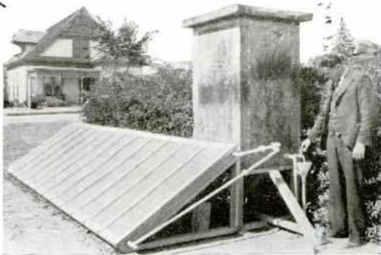
Solar Heater on Roof of Building; It Utilizes the Sun's Rays to Heat Water for Household Use
