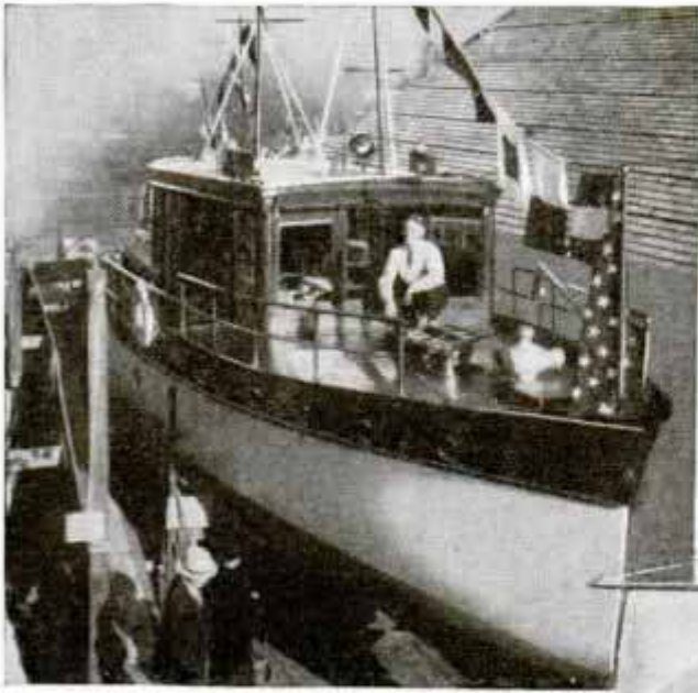
Combination Power and Sail Cruiser Built in the Designer's Backyard; the 150-Horsepower Engine Develops Twenty Miles per Hour
