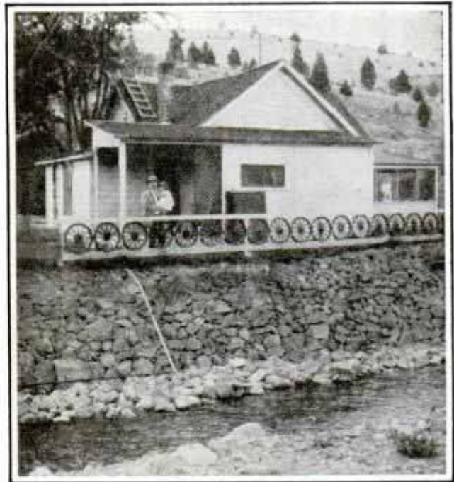
Discarded Auto Wheels, Held in Line by Rails at Top and Bottom, Make Unusual Fence
