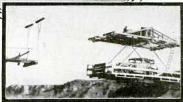
Two Views of Automobile Ferry Making Trip on Suspended Cables across the Colorado River
