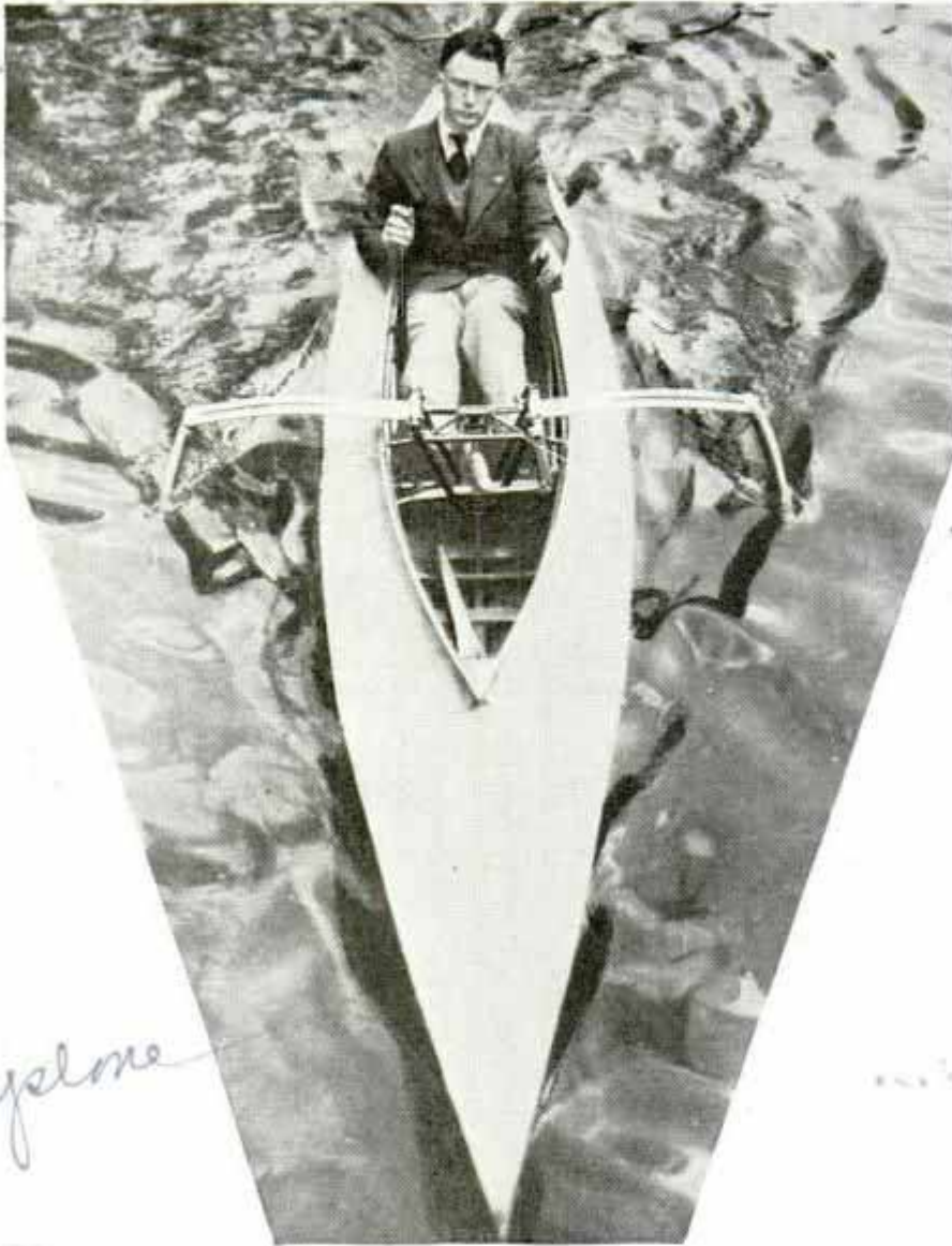
Water Craft with Two "Wings" Which Move Vertically Instead of Horizontally and Are Operated by Hand with the Aid of Two Levers
