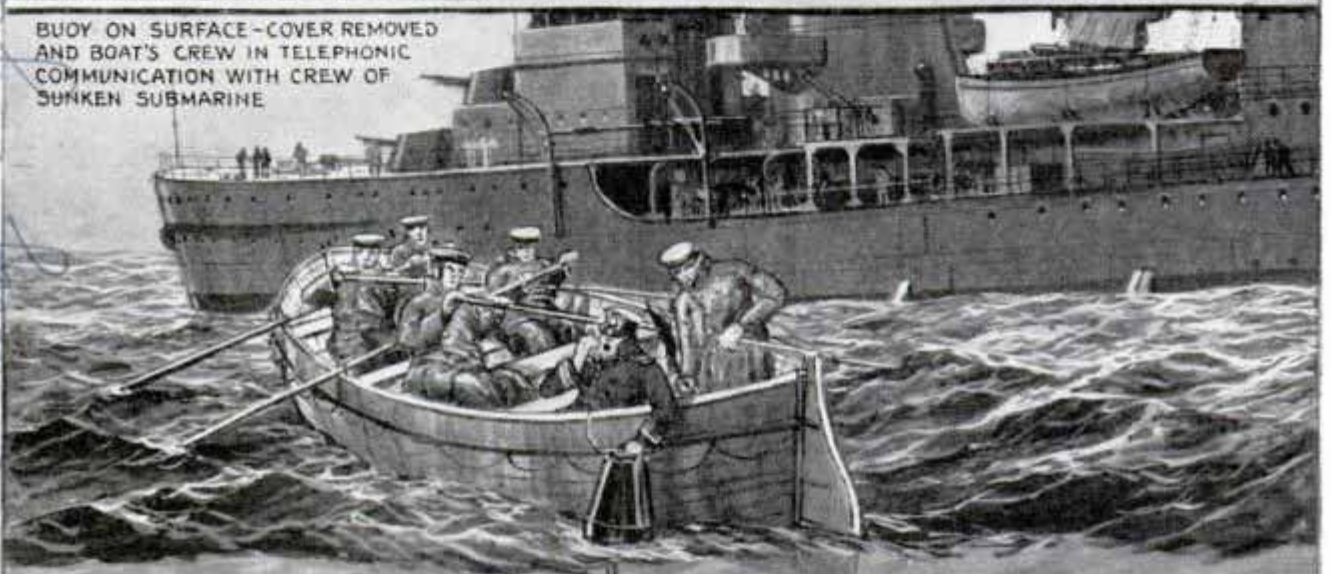
TELEPHONE AND LIGHT CABLES
