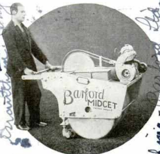
Hand Roller Operated by a Gasoline Engine at Speed of About Two Miles per Hour
