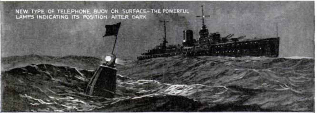
BUOY ON SURFACE - COVER REMOVED AND BOAT'S CREW IN TELEPHONIC COMMUNICATION WITH CREW OF SUNKEN SUBMARINE
