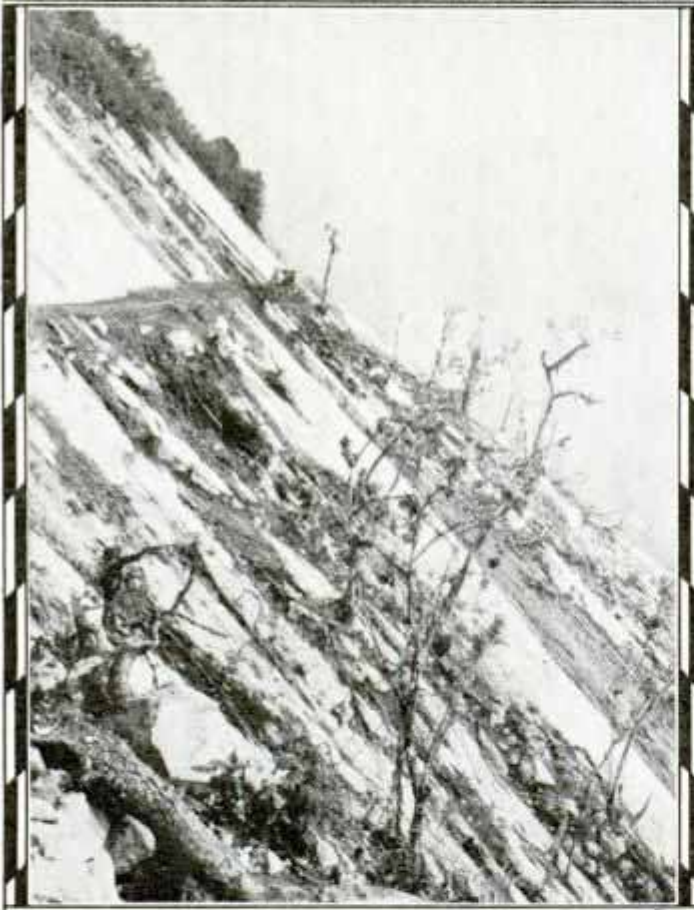
Laborers at Work on the Highway in Mexico and a Section of the Road Carved Out of Solid Rock
