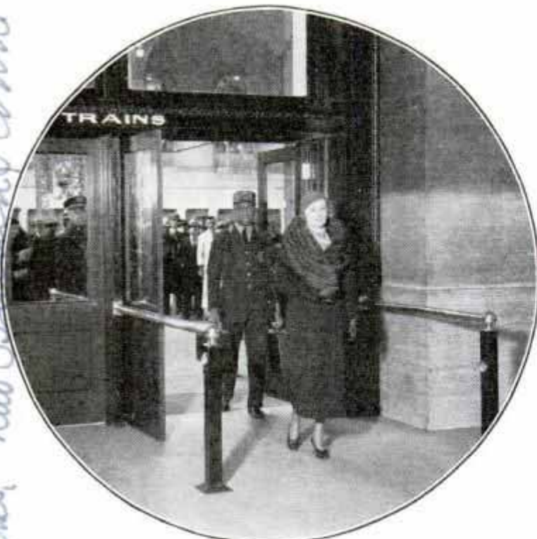
Traveler Passes through as "Electric-Eye" Arrangement Opens Doors at Station
