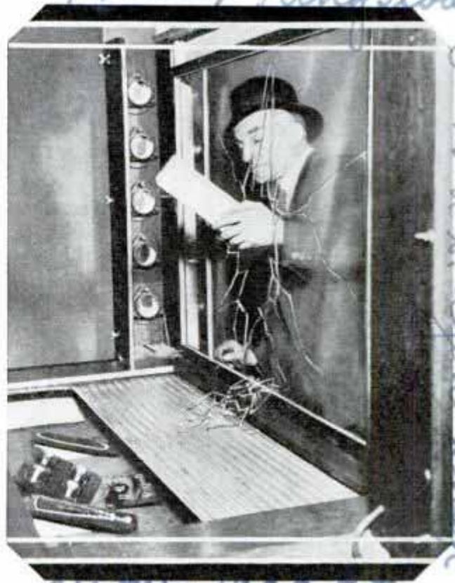
An Electric Eye Causes the Steel Guard to Slip in Place When Jewelry Store Window Is Broken
