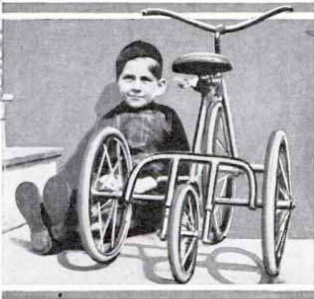
Cycle with Three Rear Wheels May Be Used as Tricycle or Bicycle by Making Adjustment
