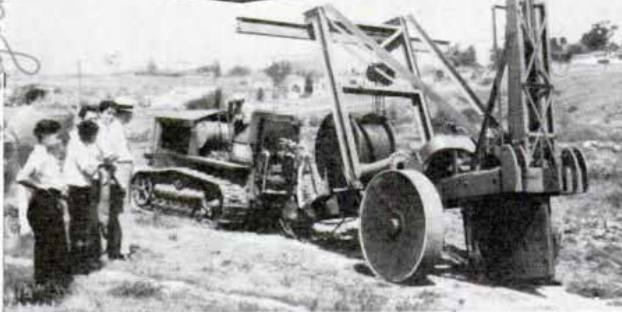
Two Views of Huge Plow Which Digs Trench and Lays Counterpoise to Guard Power Line from Lightning; It Weighs Twelve Tons
