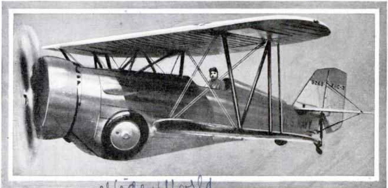
Latest Fighting Craft of the United States Navy as It Appears in Flight, with Landing Gear Retracted So That Wheels Fold against the Side; Plane Is Single-Seater and Attains High Speed
