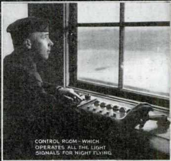
Operated from Control Room Shown at Bottom, Right, Lights in Form of Bars and Circles Direct Student Flyers at Night; When Lights in Circle on Building "E" Flash Red, They Warn of Accident
