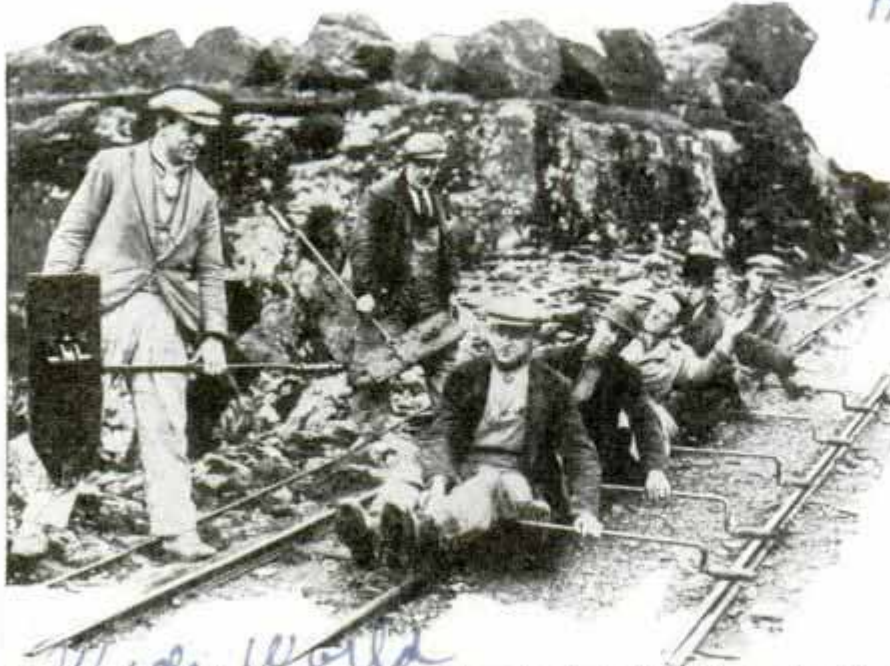
Showing How Individual Rail Cars Operate; Note One Worker Awaiting His Turn to Start for Home at Foot of Mountain After Day in Quarry
