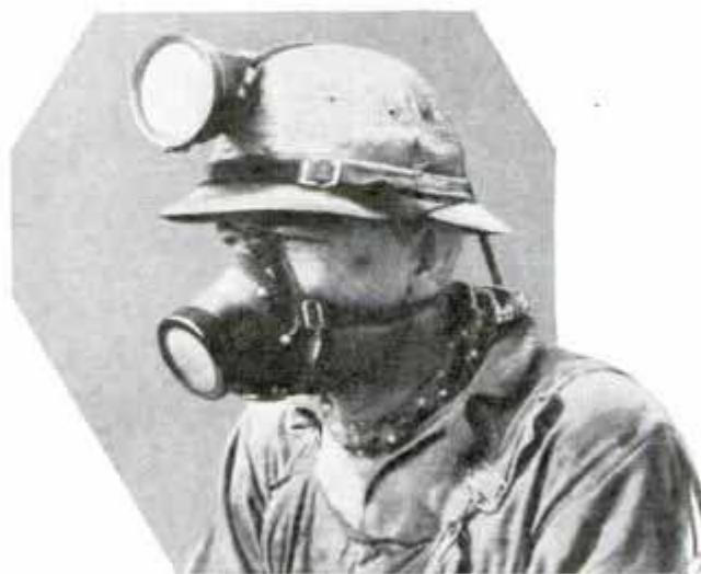
Bridge Builder Wearing Gas Mask to Protect Him from Lead Fumes, and Helmet with Lamp
