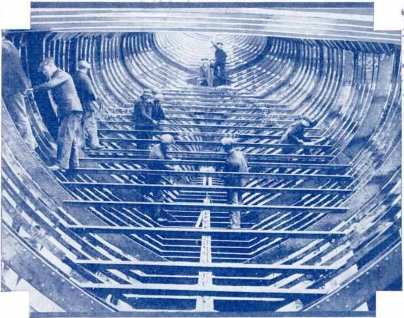
Hull of T. O. N. Sopwith's Challenger for America's Cup Is Shown under Construction; Christened "Endeavor," the Yacht Is Expected to Give "Rainbow" a Close Race
