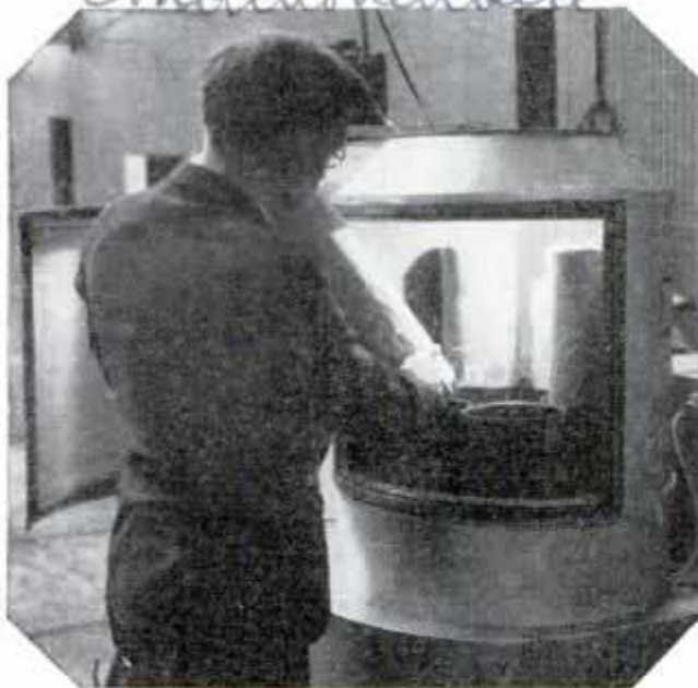
Loading Magazine of Home Heating Plant with Paper-Wrapped Coal "Sticks"
