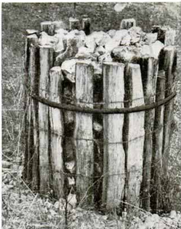
Circular Enclosure of Old Posts Is Filled with Rocks to Provide Sturdy Corner Fence Post
