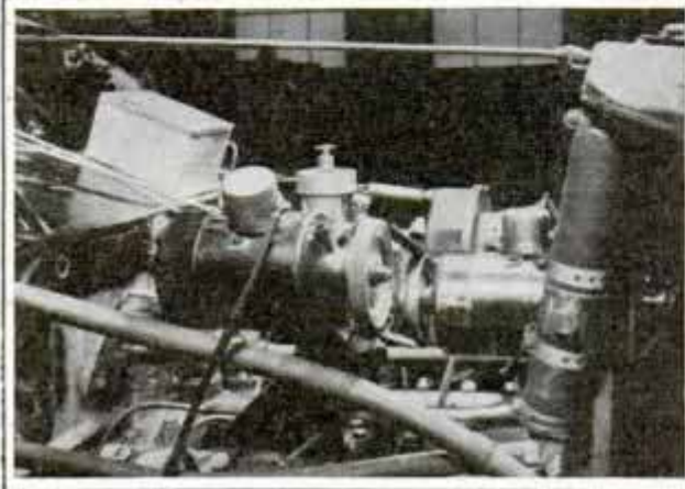
Additional Generator Installed; Above, Shaft and Pulley Details
