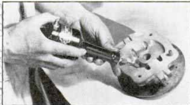
Lightweight Electric Grinder Is Handled as Easily as Pointing a Pencil
