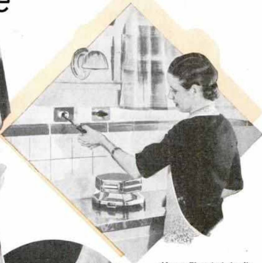
Above, Electrical Appliance Cord on an Automatic Reel; When Not in Use, It Is Disconnected, Given a Gentle Pull and Rolls Up and Disappears in the Wall
