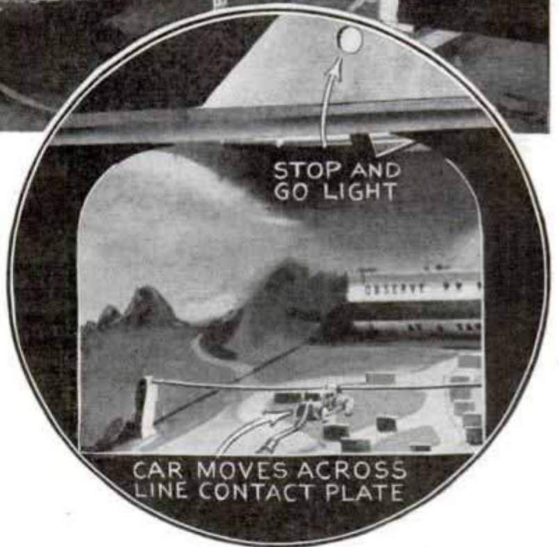
Dummy Car for Testing Driving Skill; Right, Toy Car and Moving Highway Screen Watched by Driver Tested
