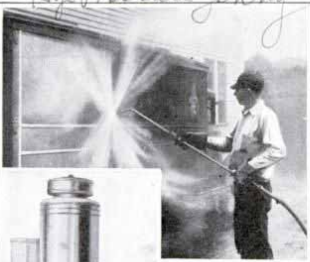
Top, Chemical Vapor Gun for Removing Paint Is Shown in Operation; Note Light-Colored Section from Which Paint Has Been Blown; Left, Sketch of Equipment
