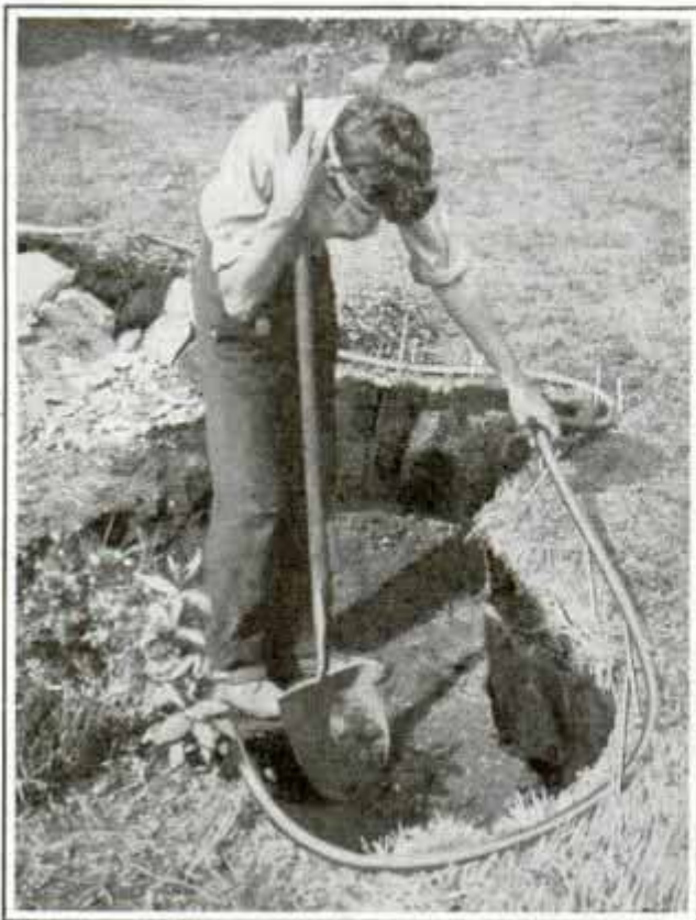
Garden Hose Used as Template to Lay Out Garden Pools of Irregular Shape
