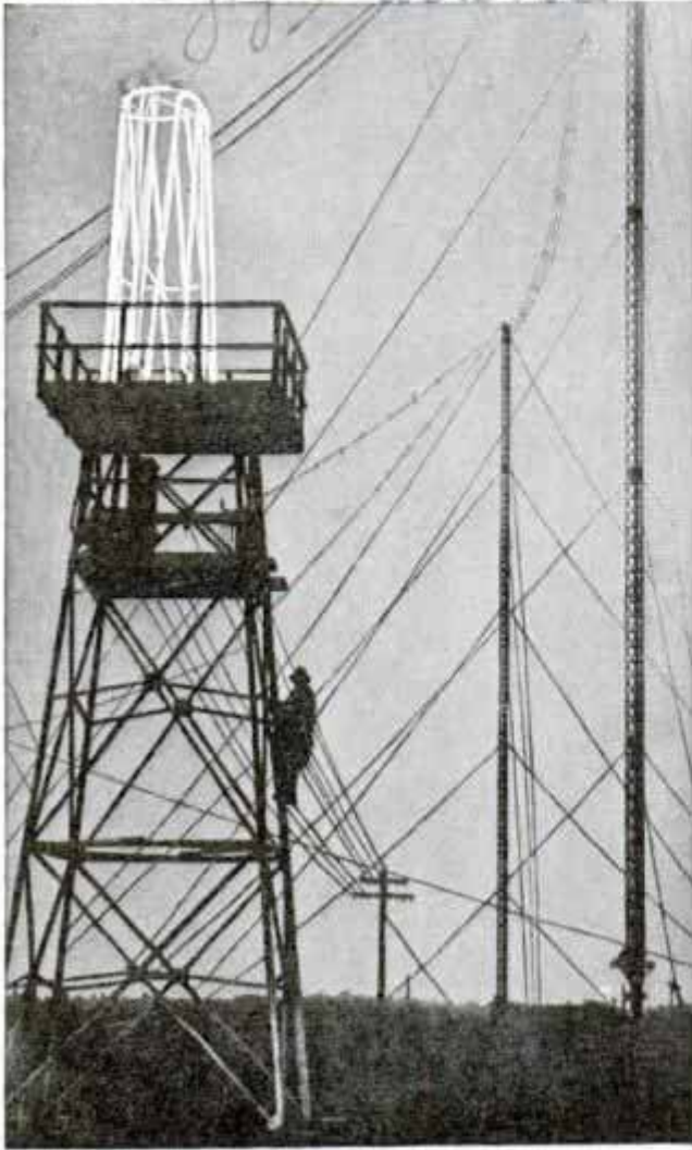
Tower Illuminated with Neon Tubes to Warn Aviators Away from Masts of Wireless Station
