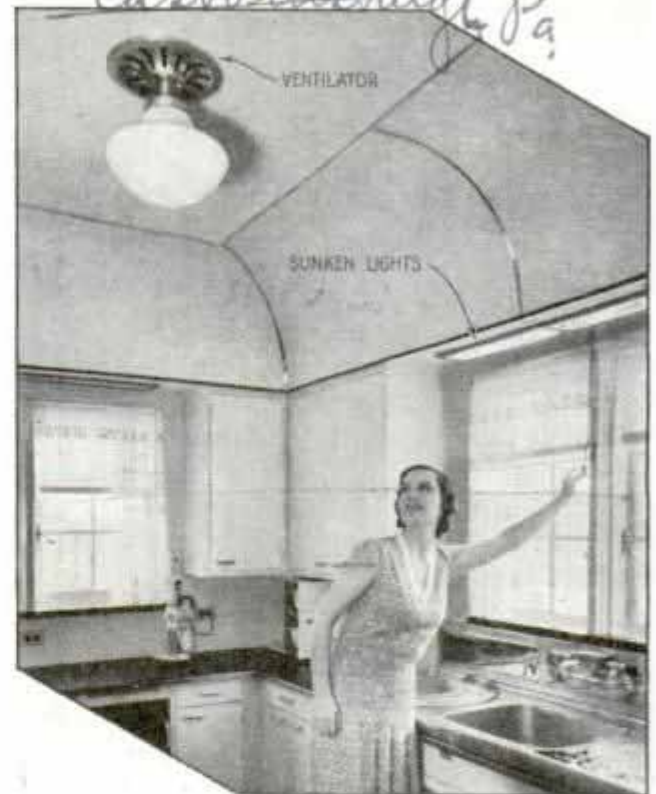
Switch at Center of Window Controls Ventilator Fan over Central Light in the Kitchen
