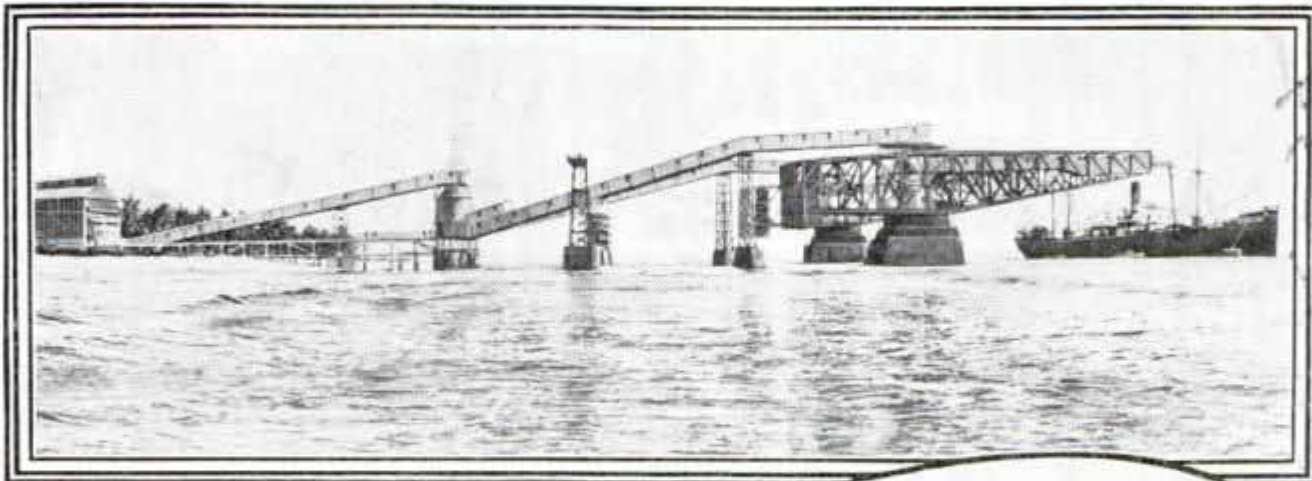
© Henry Simon Conveyor and Loading Arm Shown Discharging Phosphate into Ship's Hold; Right, Close-Up of Ship and Giant Arm
