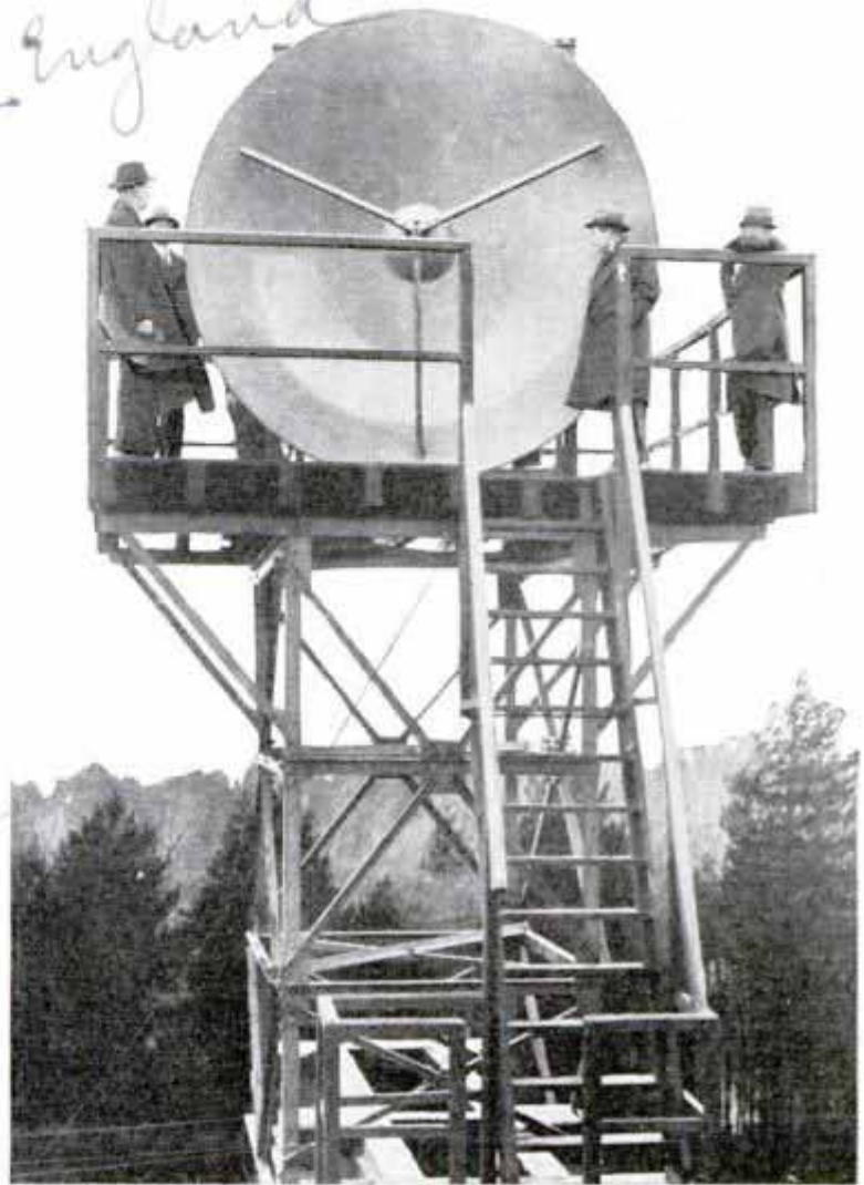
© Planet News Giant Reflector Mounted Atop Short-Wave Tower Is Used in Cross-Channel Radio Communication
