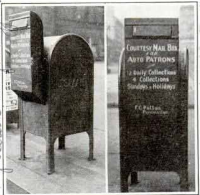
Special Chute Attached to a Curbside Mail Box, Making It Easy for the Motorist to Mail Letters
