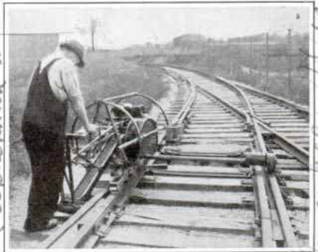
Latest Track Wrench with Its Own Motor Is Rolled along the Tracks as Shown Here
