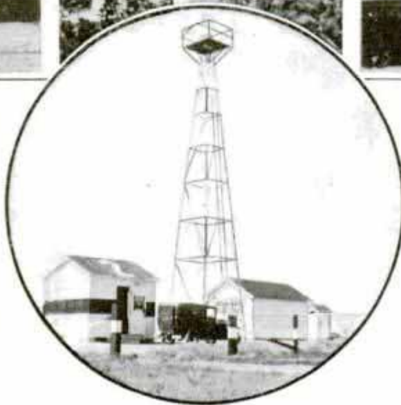
Top, Left to Right, Automatic Lamp Changer for Beacon, Acetylene Flasher and Astronomic Clock; Below, Isolated Beacon and Its Electric Plant
