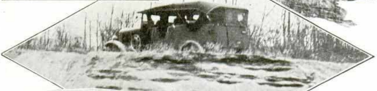
Car for Cross-Country Travel Which Has Four-Wheel Drive, Ten Speeds Forward and Four Reverse
