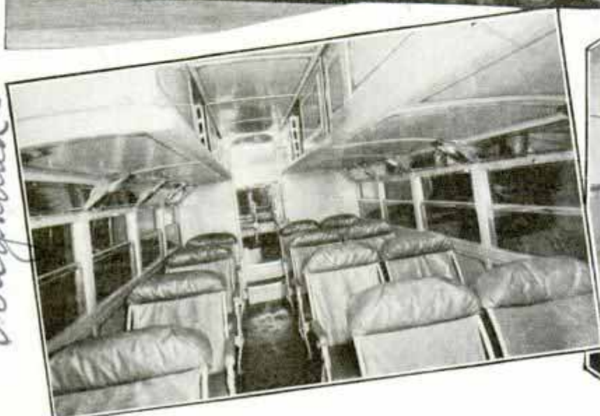
Interior and Exterior Views of Motor Coach for Travel across Syrian Desert; It Seats Thirty-Five Passengers and Is Powered with a Diesel Engine; Note Buffet Arrangement
