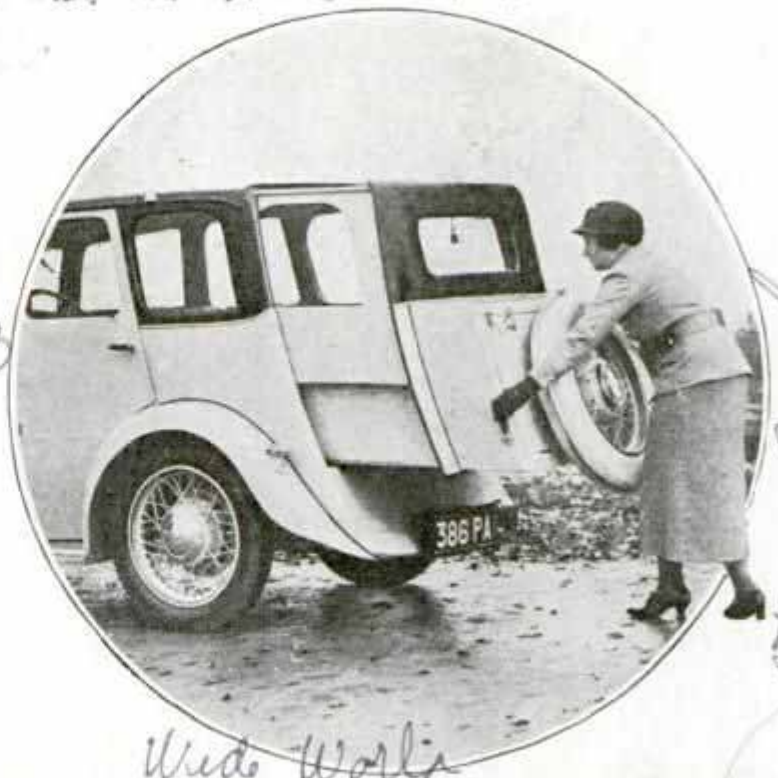
Walter Gooche Automobile Body with a Telescoping Rear Section Which, When Extended, Transforms It into a Bed
