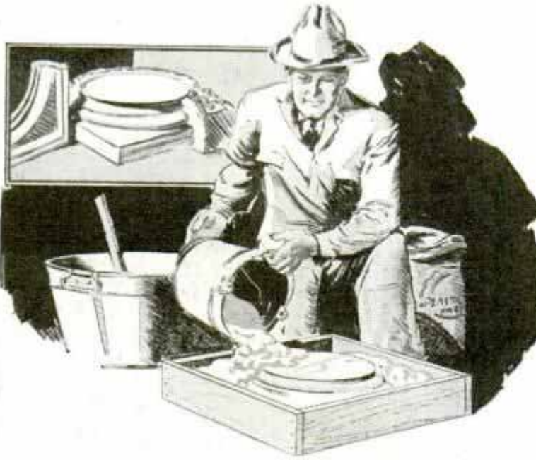
Plaster-of-Paris Mold of Rotted Porch-Column Base Used to Form Permanent Base of Concrete
