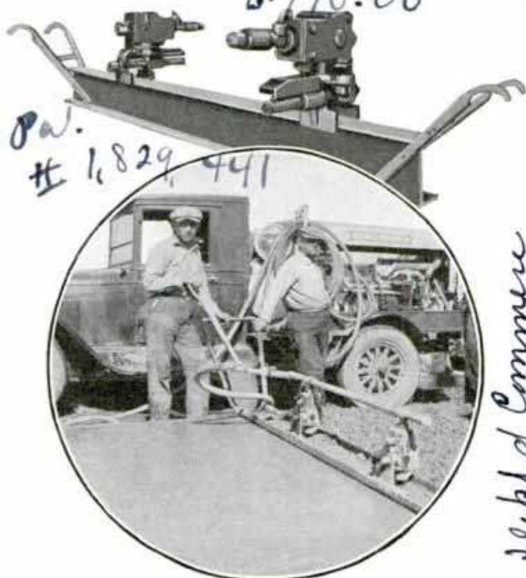
Vibrator Board for Tamping Concrete Is Handled Easily; Vibrators Are Air Driven
