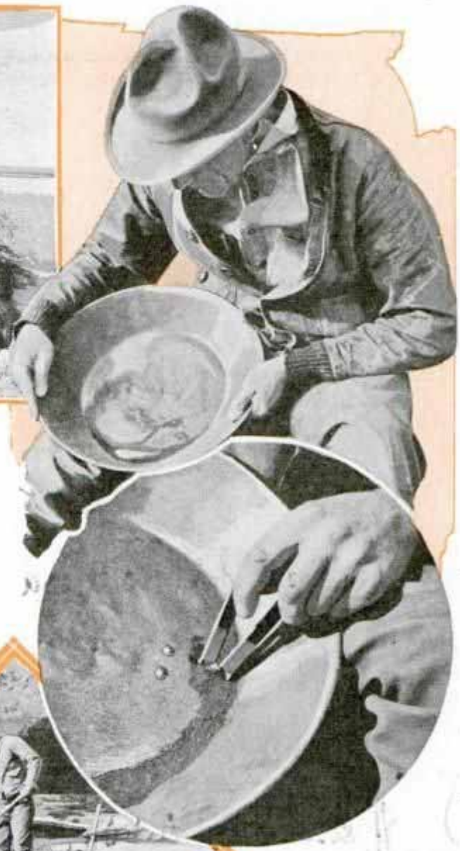
Above, Panning Operations; Removing Gold with Quicksilver, and Black Sand with a Magnet
