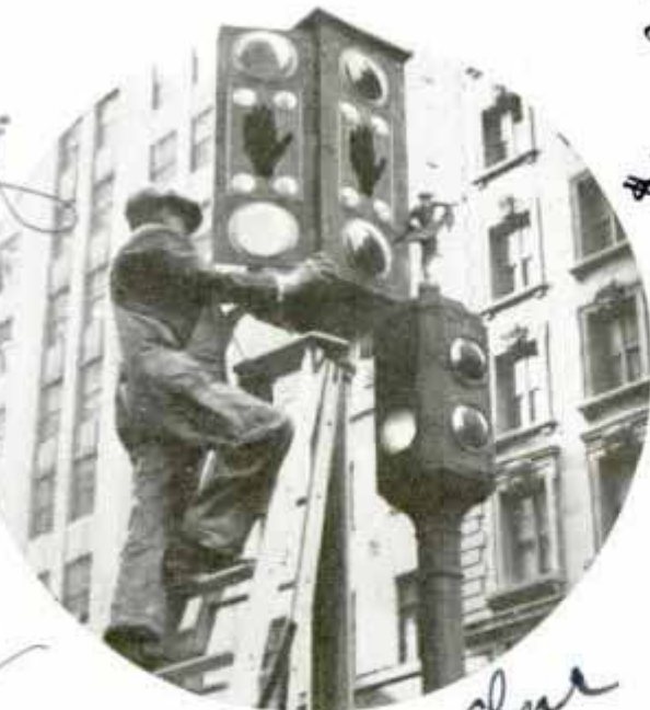
Traffic Signal with Lighted Hands Which Stop All Vehicles for Pedestrians to Cross
