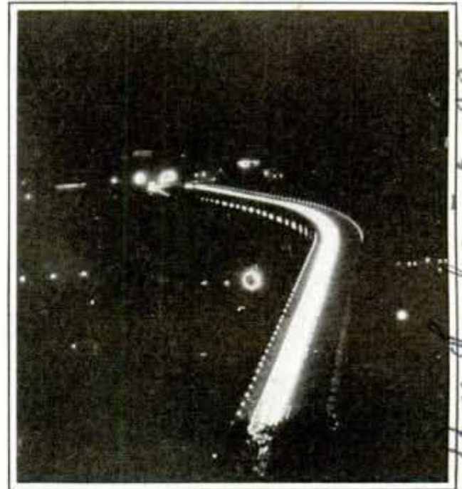
Cincinnati Bridge Illuminated with Underfoot Lights Which Eliminate Most of Glare
