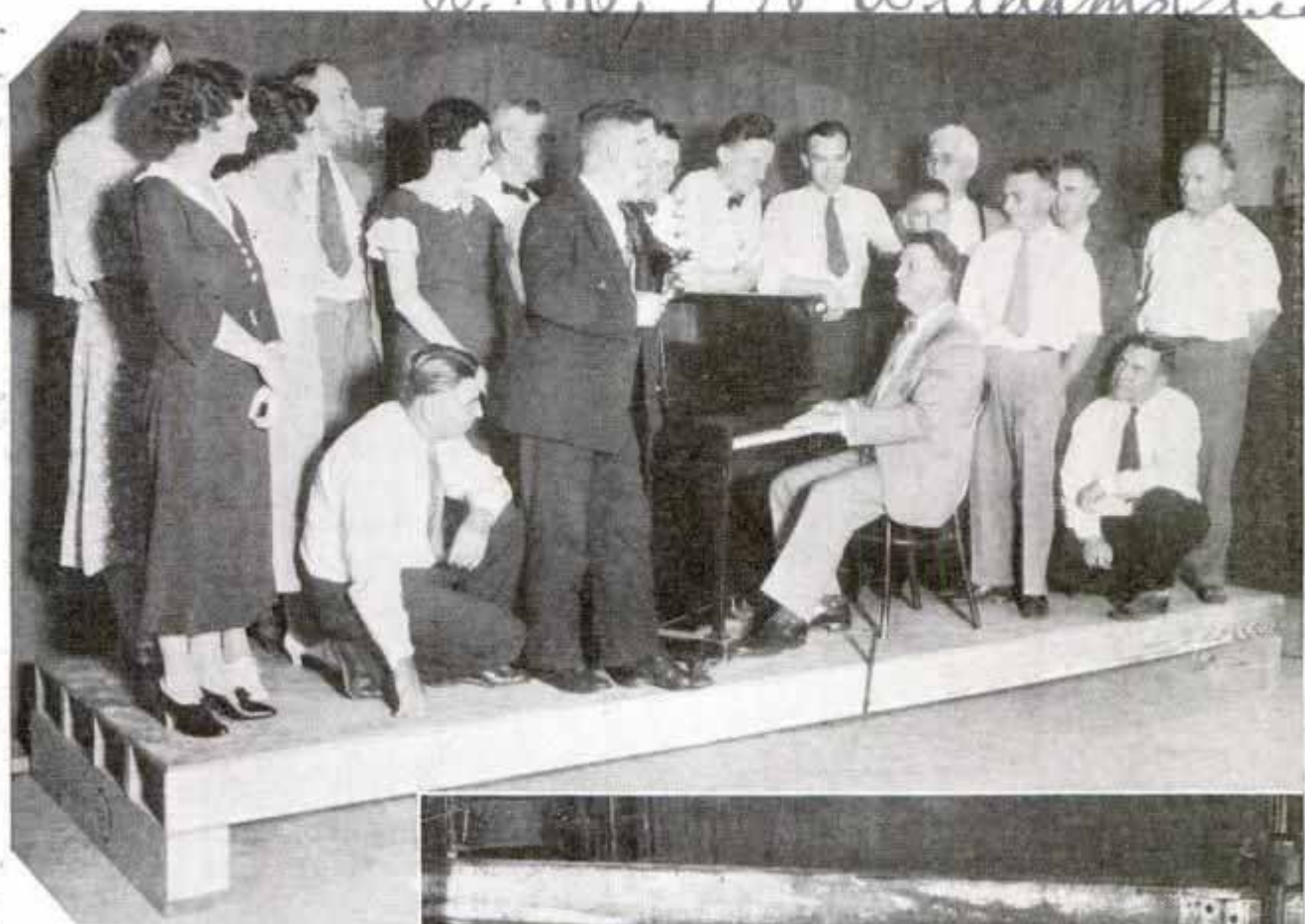
Top, How New Floor Panel Supports Unusual Loads; Bottom, Showing How New Type of Panel Occupies Less Space
