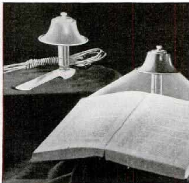
Electric Reading Lamp Only Four Inches Tall Which Can Be Attached to the Book Cover
