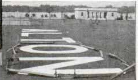
Cities Are Marking Their Names on the Ground with Huge Letters to Aid Lost Flyers in Identifying the Towns; Left, Cutting away Sod Preparatory to Filling Shallow Trench with Rock or Concrete; Below, Finished Marker
