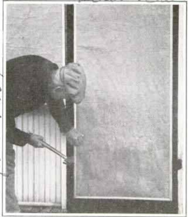
Tacking Special Paper on Screen Door to Make It Proof against Cold and Wind
