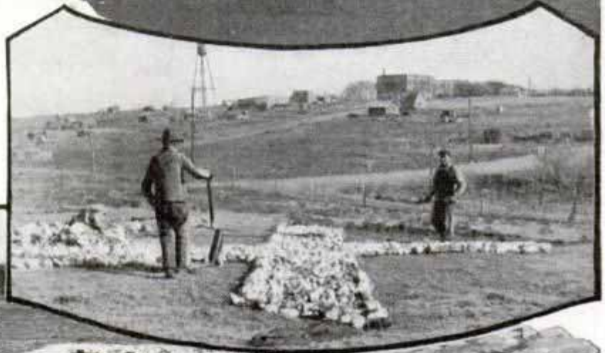
Right, Finishing a Skyway Marker by Filling Outline of Letters with Broken Concrete Which Is Then Sprayed or Painted with Lime Solution, Making the Letters, Twenty by Twenty-Six Feet, Visible at Great Heights; Below, Part of a Marker Made of Sandstone
