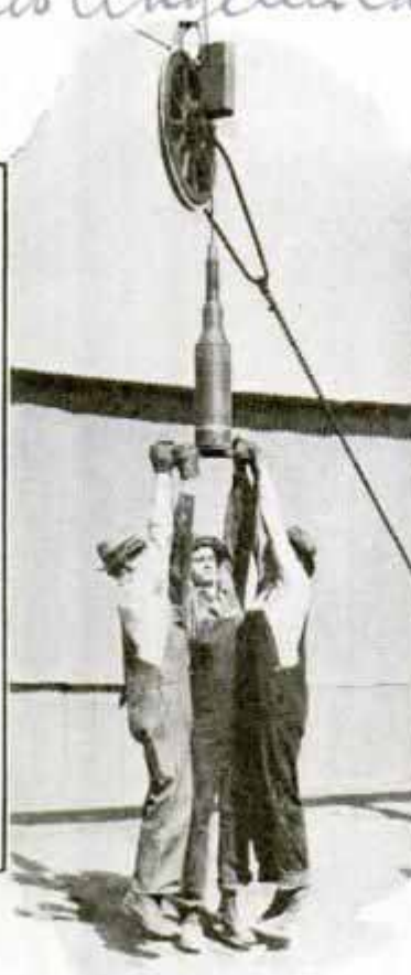
Two Demonstrations of Power of Electromagnet Used in Oil-Well "Fishing"
