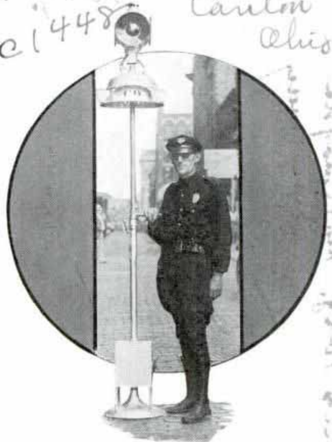
Policeman Operates Signal Light Which Derives Its Current from Storage Battery
