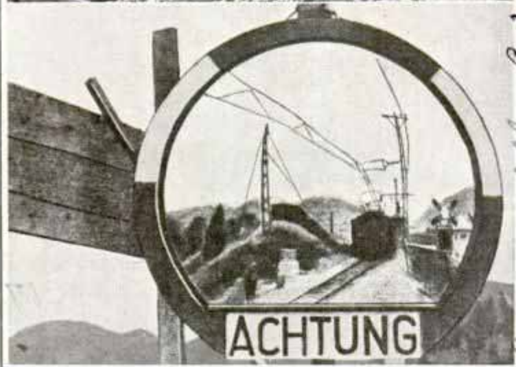
Large Mirror at Railroad Crossing Which Shows Motorist When Train Is Approaching around a Curve
