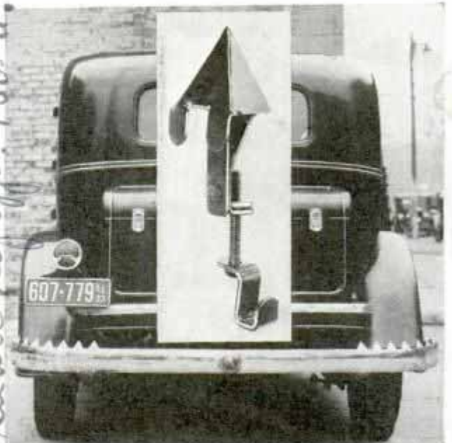
Sharp-Pointed Device for Keeping Hitch-Riders Off Bumpers; Enlarged on White Strip
