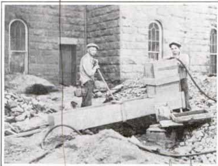
Backyard of Old Carson City Mint Where Mining Operations Are Being Carried on to Recover Gold Lost in Sweepings
