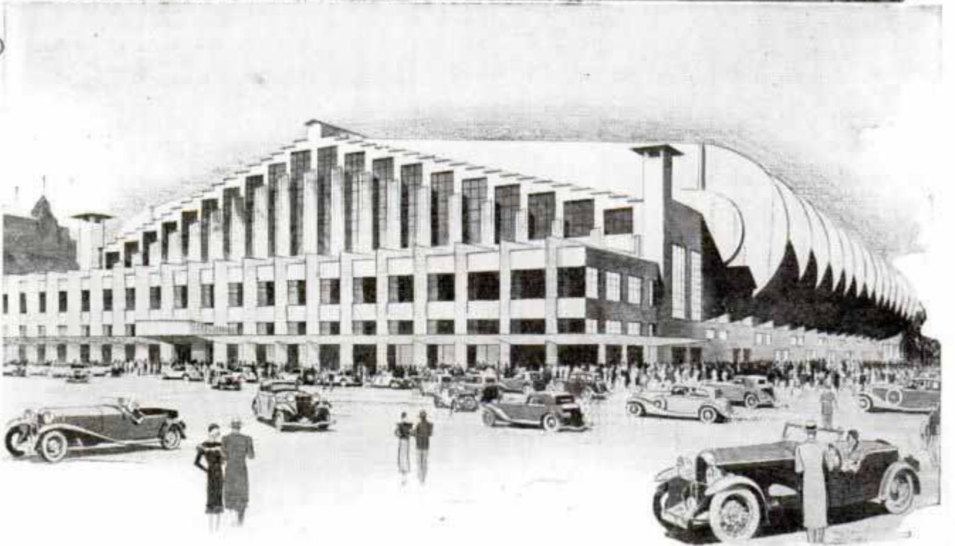
Glass Swimming Stadium, Seating 8,000 Spectators, Being Built around a Lake at Wembley, England; Waves Are Produced Artificially and Pool Can Be Frozen for Ice Sports
