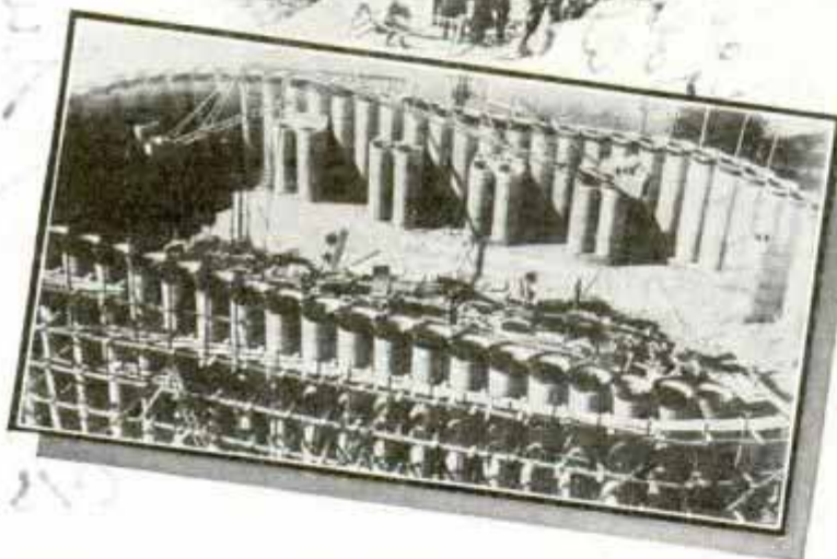
Top, Launching Tube Unit for Bridge; Bottom, Left, Building Unit; Right, Preparing the Arches
