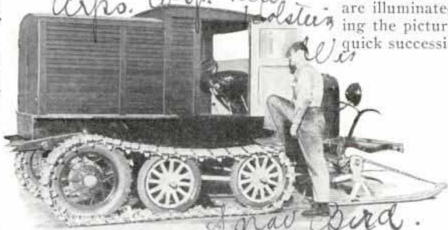
This Strange Vehicle Will Enable Antarctic Explorers to Travel over Snow; Note Special Tread Provided for the Six Wheels
