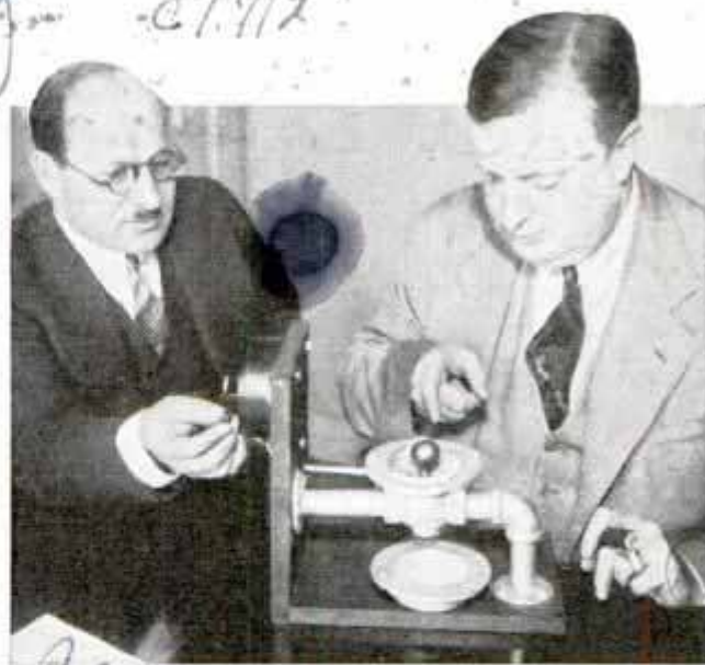
Man at Right Points to Balanced Ball Which Actuates Gas Shutoff When Earthquake Strikes
