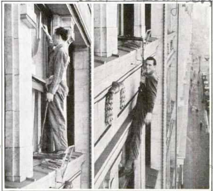
Left, Window Washer Standing on Safety Platform; Right, Worker Hanging by Safety Belt After He Has Fallen from the Platform
