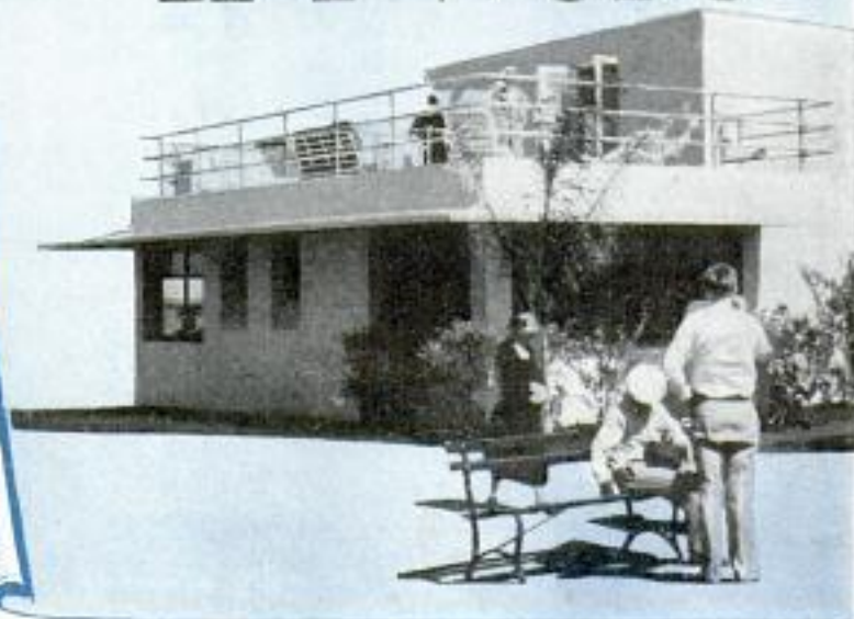
Top, Left, Brick House with Floors, Walls, Ceilings and Roof as Unit Held in Place by Steel Rods; Bottom, Florida House
