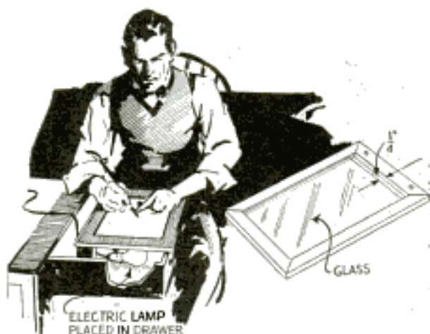
Tracing Drawing on Mimeograph Stencil with Equipment Improved from Glass and Picture Molding
