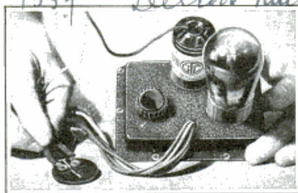
Short-Wave Converter That May Be Used with Any A.C. Broadcast Receiver
