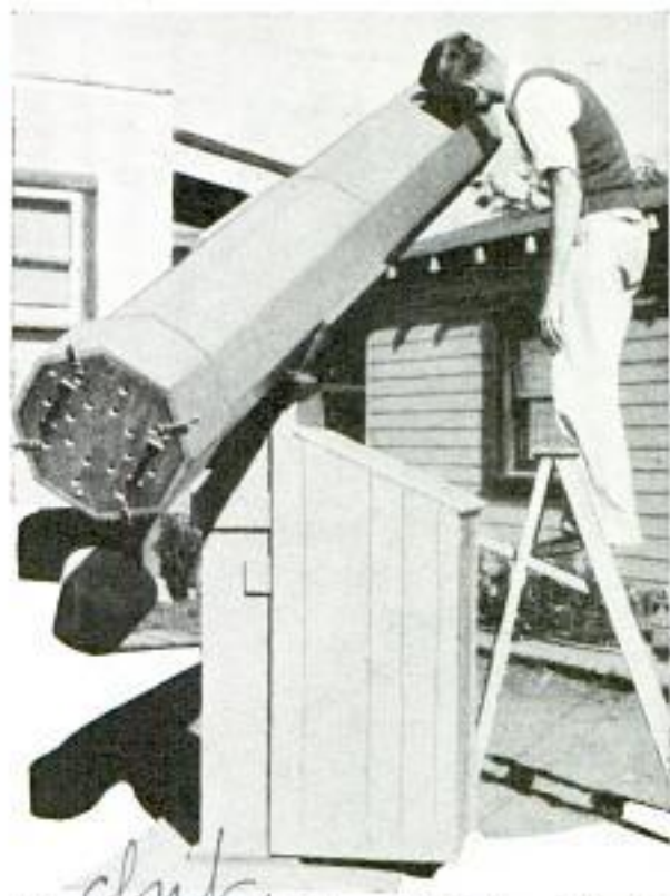
Telescope Constructed of Parts of Old Auto, Discarded Phonographs and Other Odds and Ends
