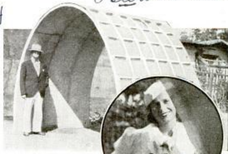
How New Concrete May Be Shaped; Inset, Showing Mirrorlike Characteristics of the Finish
