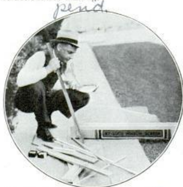
How Window Screen May Be Assembled
