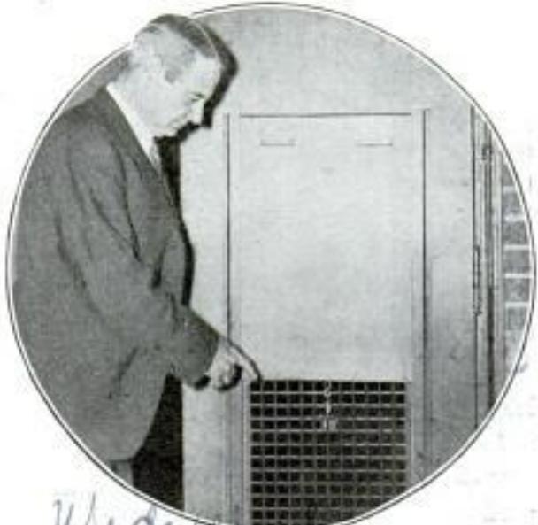
Sliding Shutter in Steel Door Which Closes Ventilator Panel in Case Fire Breaks Out
