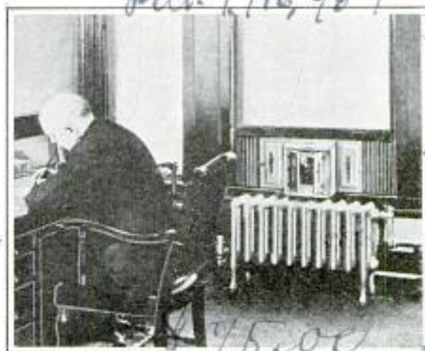
Apparatus in Window Keeps Air Conditioned in Office; Air Is Drawn from the Outside
