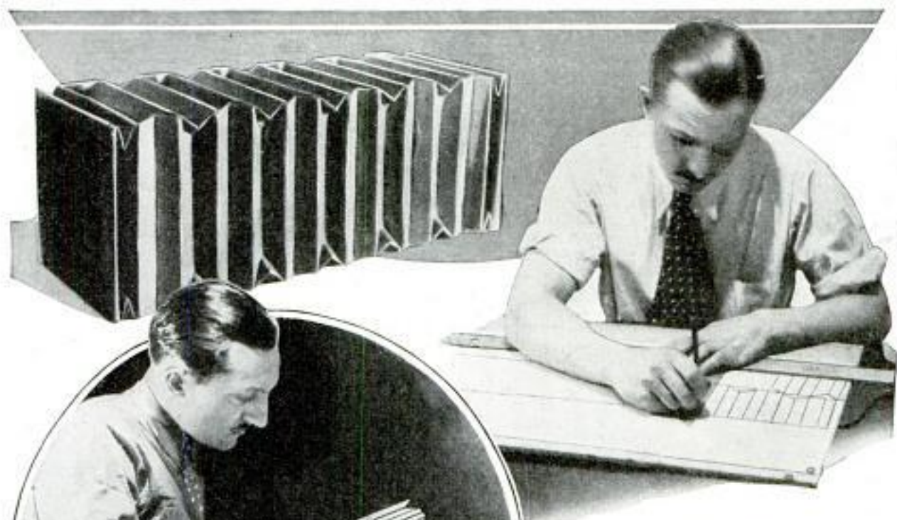
Sides of the Bellows Consist of Numerous Segments Glued between Two Pieces of Heavy Black Satteen
