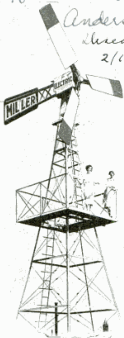
Tower and Three-Blade Propeller of Wind-Power Plant; Blade Unit Has Speed Governor
