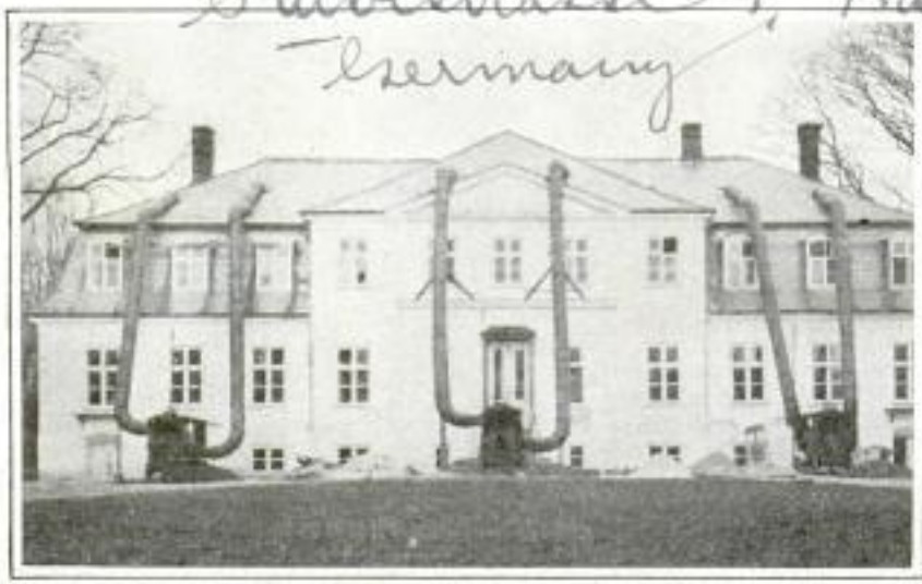
Three Gas-Air Blower Plants Shown in Use, Drying Out Interior of New Building; This Method Reduces Delay Before Structure Is Occupied
