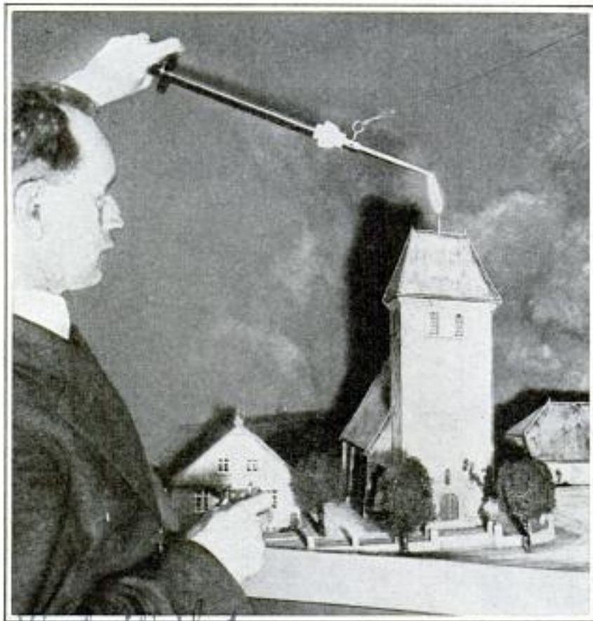
Wide World Model of Village Church Helps to Demonstrate How Conductors to Ground Protect the Structure against Artificial Bolt of Lightning
