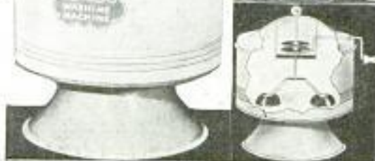
Right, Nine-Inch Washing Machine Operated by Turning Hand Crank; There is a Detachable Wringer with Rubber Rollers; Vacuum Cups Rotate Like Those in Full-Size Washers
