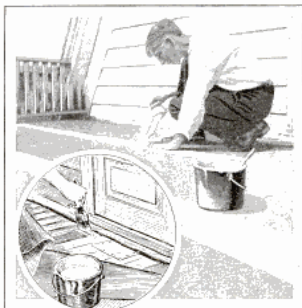
Annual Painting of Canvas-Covered Porch Decks Is the Best Preventive against Leakage
