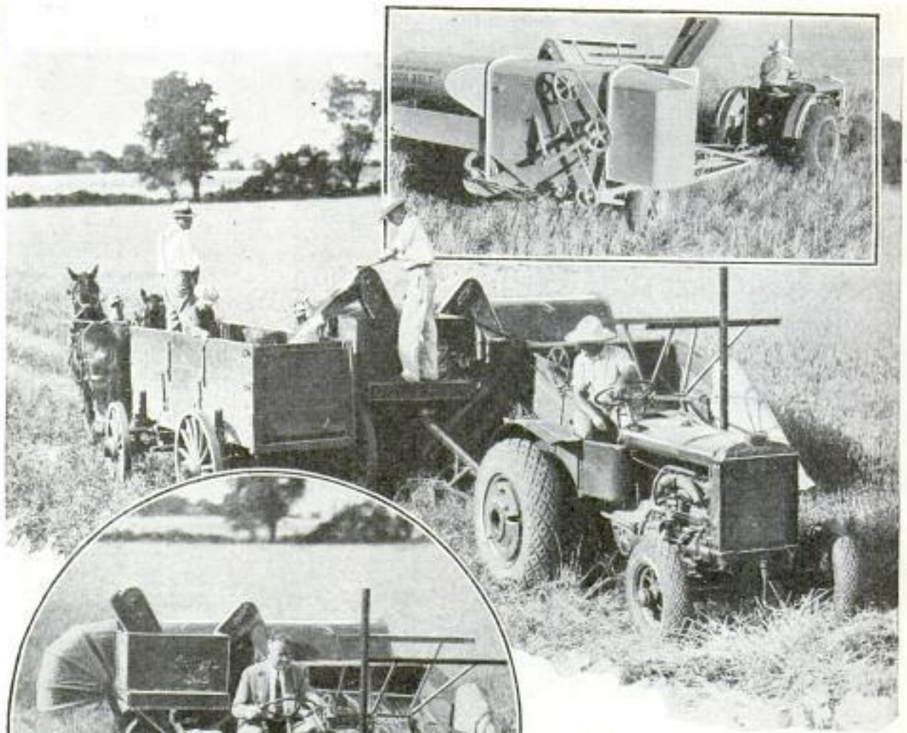
Two-Wheeled Baby Combine Being Operated by Tractor with Pneumatic Tires; It Cuts a Five-Foot Swath
