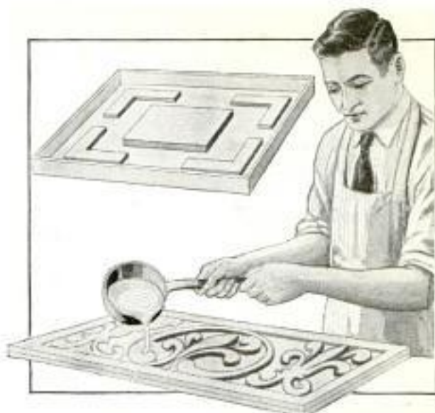
Buhlwork Imitated by Pouring Colored Concrete into Molds Containing Patterns of Wood or Metal
