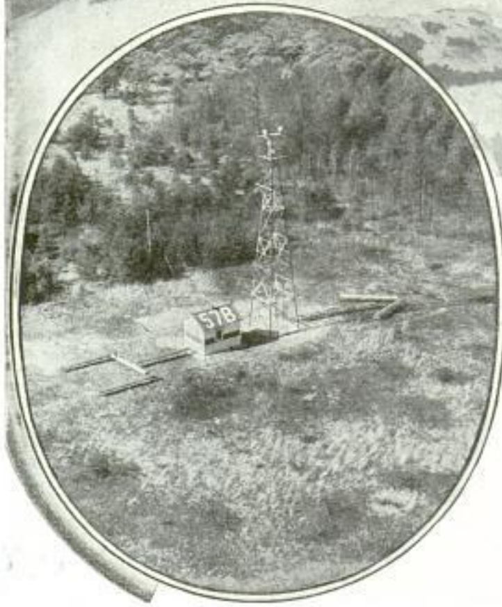
Left, Latest-Type Rotating Airways Beacon That Flashes Green if Landing Field Is Located Near; Note Number of Beacon on the House
