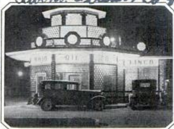
Made of Glass Blocks. This Illuminated Filling Station Is Visible for Long Distances
