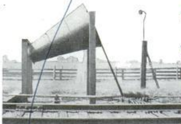
Megaphone-Shaped Device Catches Steel Pins Used in Locking Stretch of Tracks
