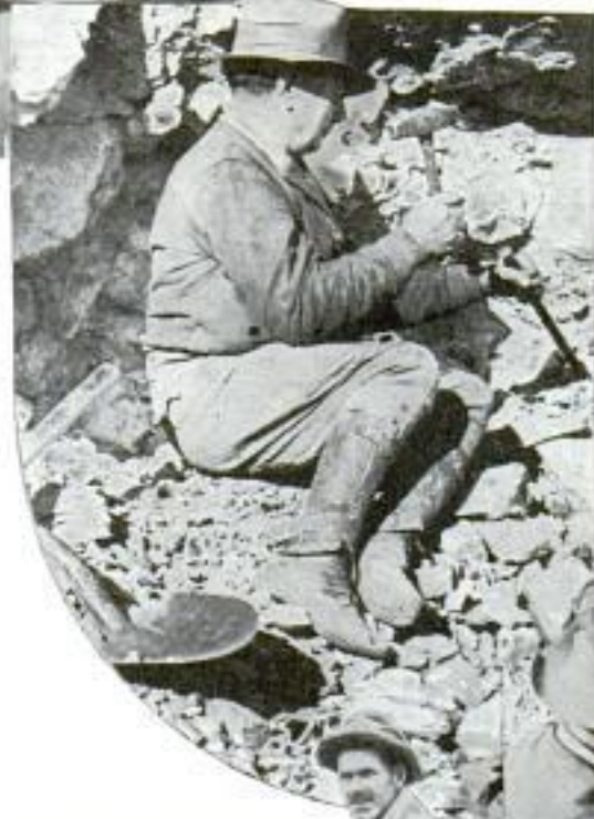
Above, Drilling for Blasting; Below, a Homemade Dry Washer
