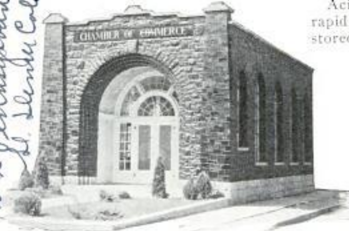
This Building Contains More Than Sixty Tons of Coal; the Walls Resemble Stone, but Are Rough-Hewn Blocks of Coal
