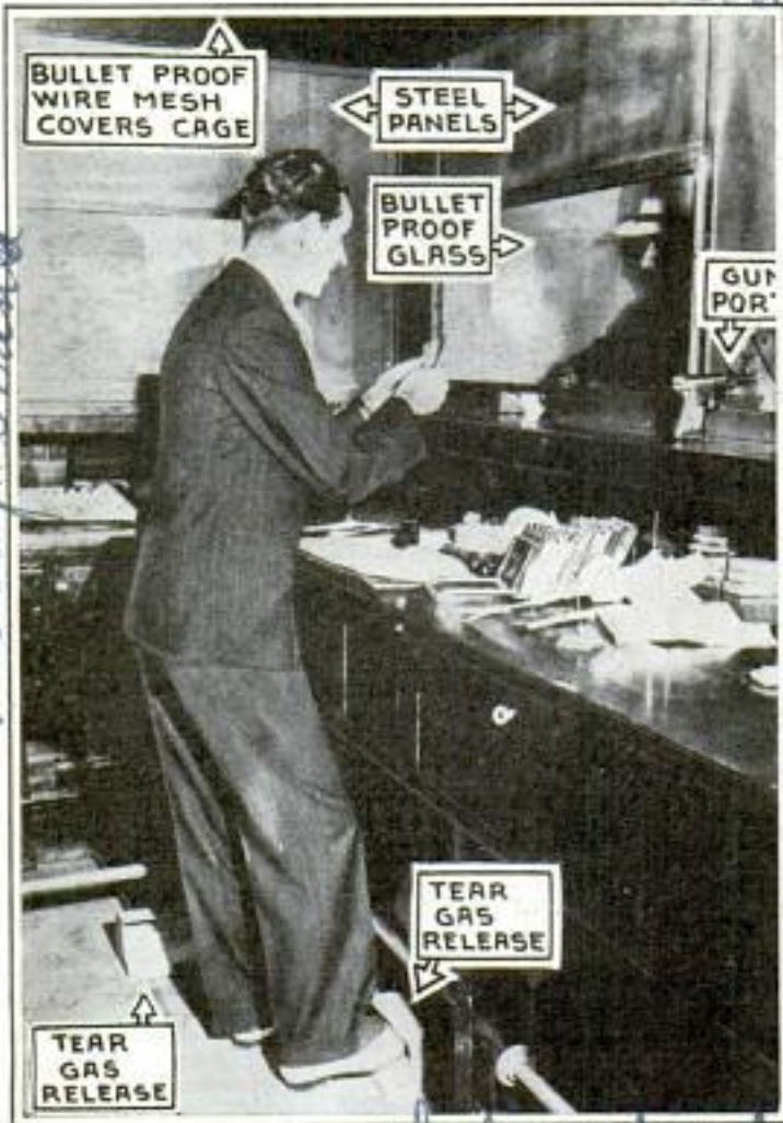
Photo Points Out Protective Devices in Teller's Cage; Note the Gun Port at Extreme Right and Tear Gas Releases on Floor
