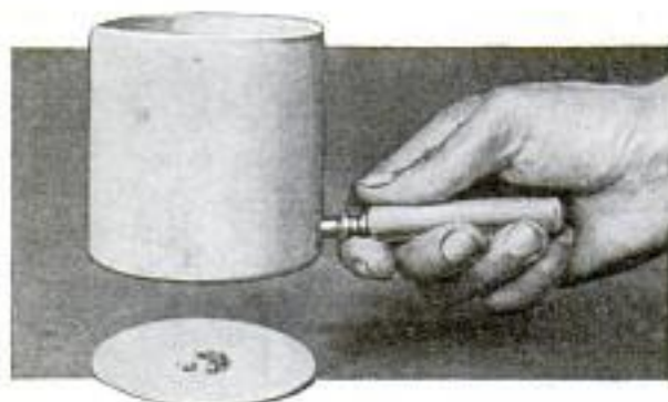
A Reading Glass Can Be Improved by Mounting It Inside of a Cardboard Tube
