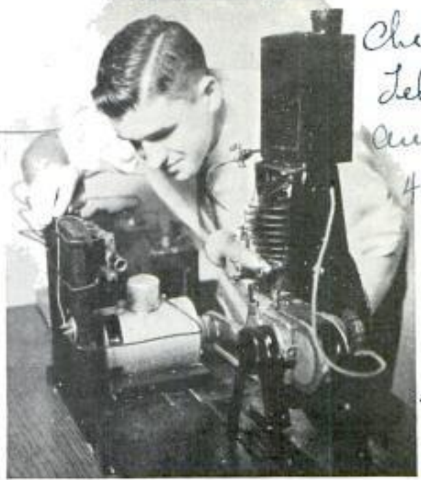
Small Engine at Right Drives This Arrangement for Lighting a House of Fourteen Rooms
