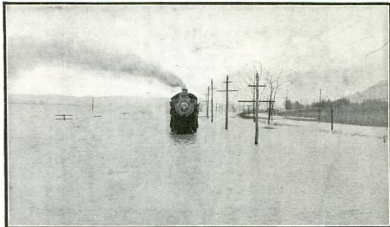
Train Nearing Outskirts of Portsmouth While the Ohio River Was at Flood Stage and Had Covered the Tracks; the City Itself Is Now Protected from Water by a Flood Wall
