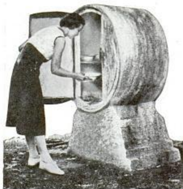
Large Concrete Tile with Ends Closed and Shelves Fitted Inside, Provides Efficient Iceless Refrigerator
