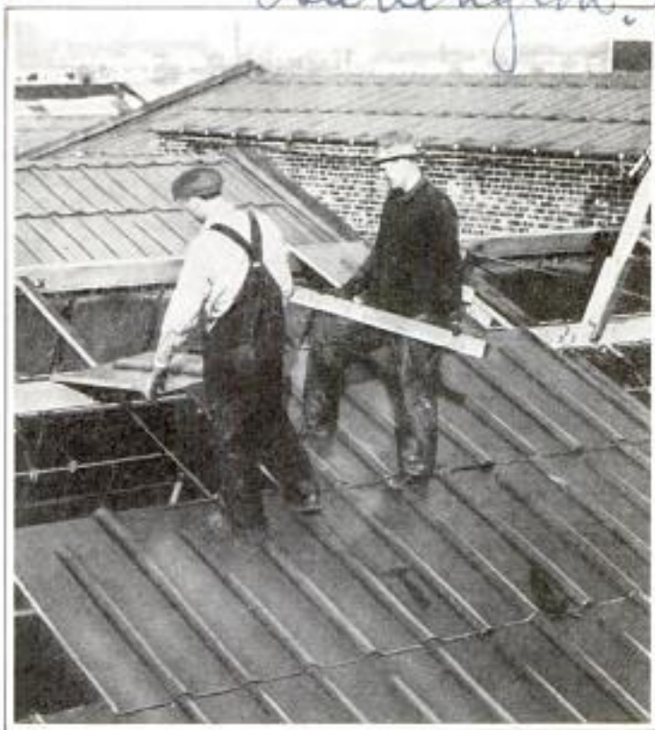
Roofing Made of Cast-Iron Plates Which Looks Like Tile When Laid; a Locking Key Holds Slabs in Place
