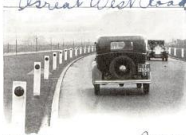
© Planet News Red Reflectors on Roadside Posts Warn Motorists at Night and Indicate Path of Highway
