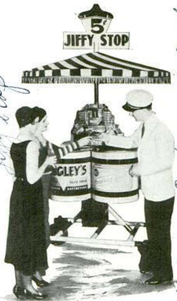
Refreshment Stand Equipped with Wheels for Moving; Note Containers for Iced Goods
