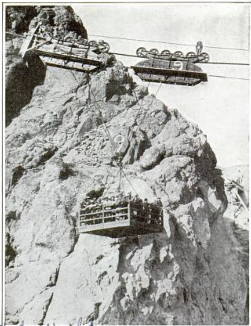
Workmen at Hoover Dam Crossing the Colorado River in an Aerial Car Traveling on a Cable 600 Feet above the Bed of the Stream
