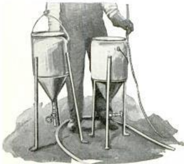
Improved Paint Containers Hoisted Near Ceiling to Utilize Gravity in Spray Painting
