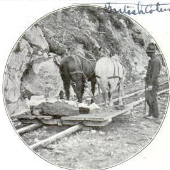
This Unusual Drag Sled on Poles Is Used for Hauling Away Rock Blasted from Highway Excavations in Canada
