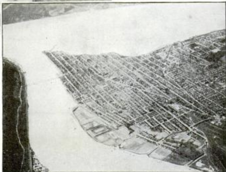
Above, Flood Wall Holding Back Ohio River; Below, Aerial View of Portsmouth Showing Section Which Would Have Been Flooded, Except for the Wall
