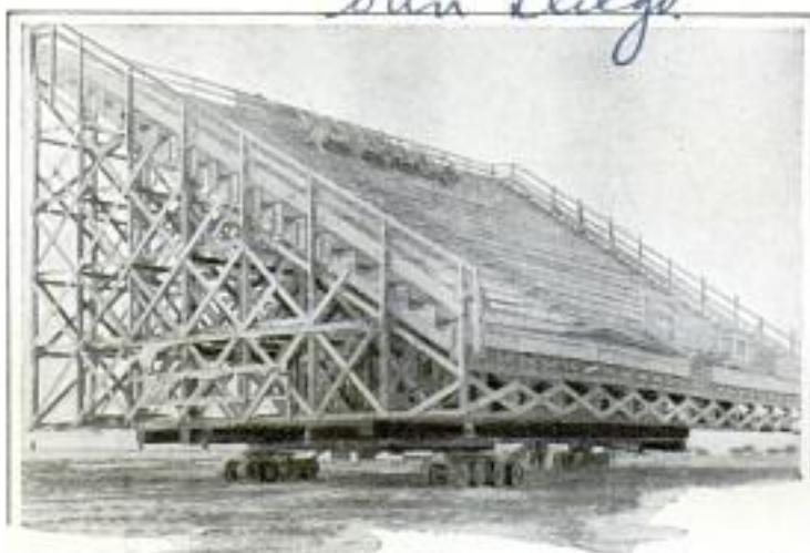
How Rollers Helped in Moving Race-Track Grandstand; After Being Placed on Wheeled Base, It Was Pulled to New Site
