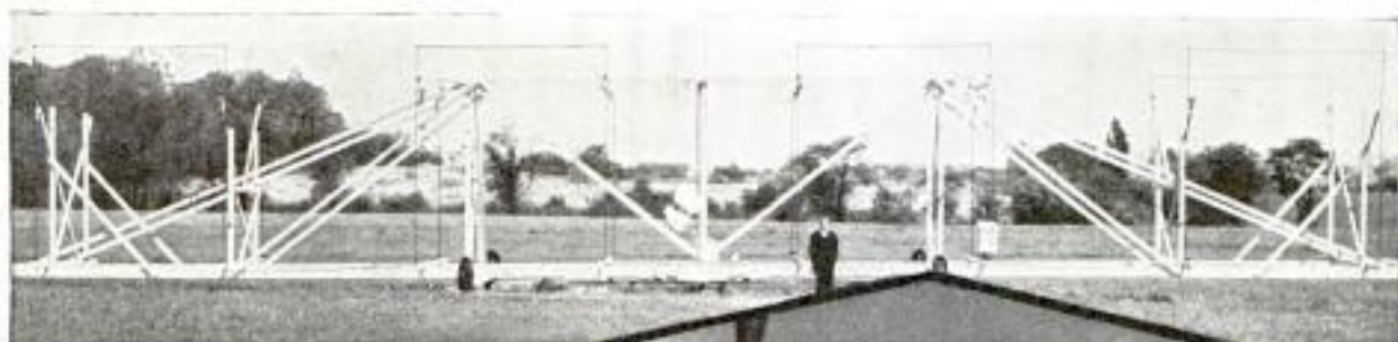
Top, Rotating Directional Antenna Used by Karl Jansky in Seeking Causes of Static Interfering with Short-Wave Communication; Right, Mr. Jansky Listening in as Static Recorder Operates on 14.6-Meter Wavelength
