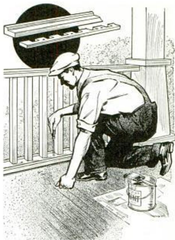
Vertical Slats in Porch Railing Made Removable by Holding Them in Place with Notched Pieces
