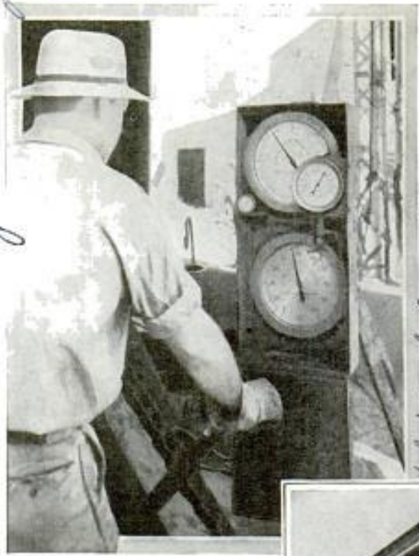
Top, Instruments for Gauging Amount of Pressure on Drilling Equipment; Right, Framework That Incloses Drill and Other Apparatus
