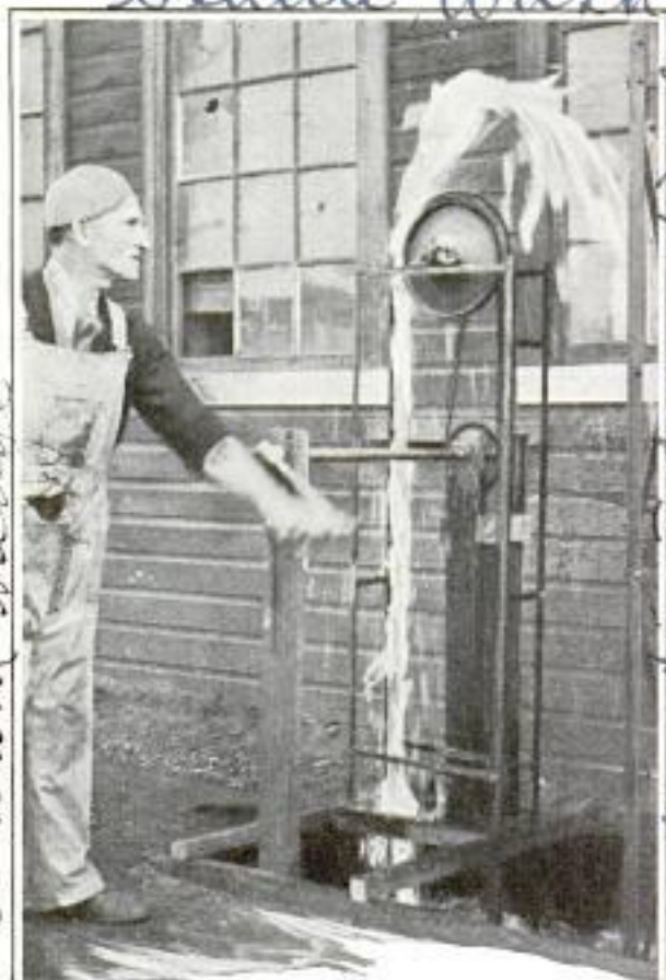
Stream of Water That Coil-Spring Arrangement Lifts Twenty-Seven Feet or More from Source
