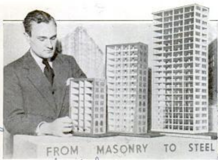
Showing Progress of the Building Industry; Model at Left Is Masonry Construction, at Right, Latest Steel Framework
