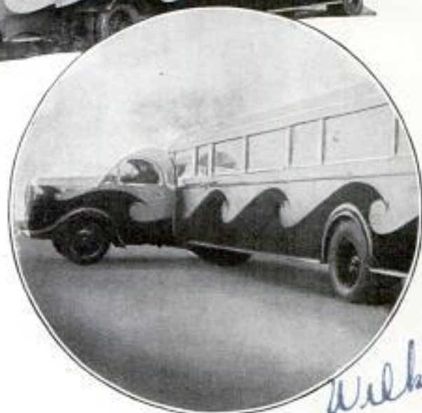
Passenger Bus in Two Sections; Circle Shows How Easily Vehicle Is Maneuvered around Corner
