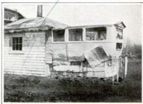
Extra "Room" Is Made from Discarded Sedan Body of Auto; It Serves as Sun Parlor
