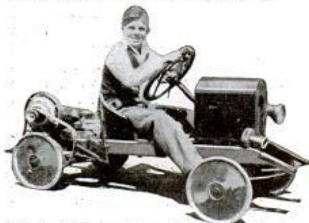
Schoolboy's Homemade Auto Which Derives Its Power from a Washing-Machine Motor
