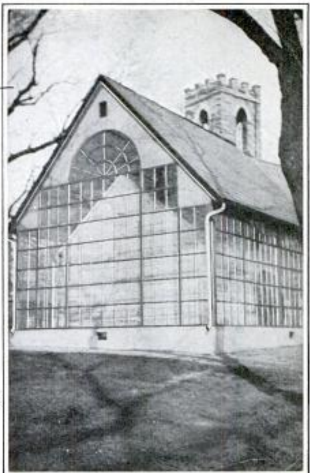
Historic Pennsylvania Church Inclosed in Glass to Permit Inspection but Prevent Vandalism
