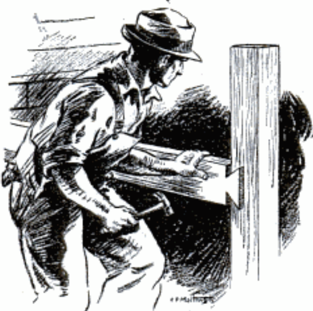
Porch Frame with Dovetailed Joints Is Rigid and Does Not Loosen if Foundation Settles
