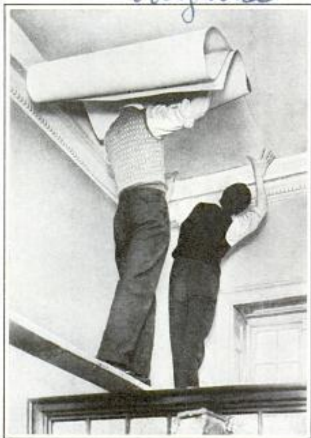
How Paper Containing Heating Element Is Applied to Ceiling: It Plugs into Electrical Outlet
