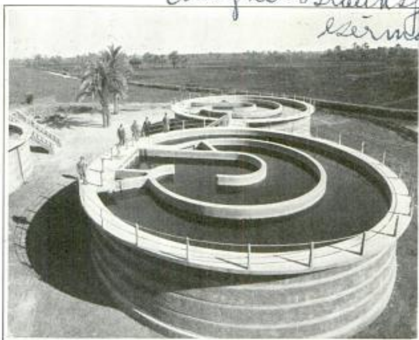
Water Containers for Desert Regions Divided into Sections; It Is Claimed This Form of Construction Decreases Evaporation
