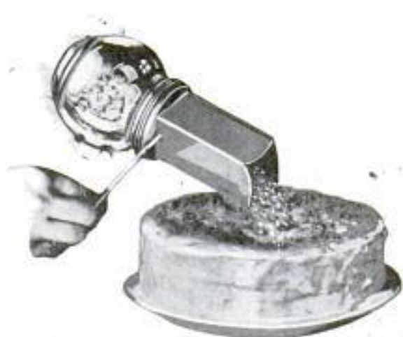
Top, Pouring Nut Meats on Cake from Handy Chopper; Nuts Are Cut Up Uniformly by Turning Crank of Chopper Attached to Top; Glass Jar Holds the Nuts; If Jar Breaks, Its Top Fits Standard-Size Mayonnaise Jars; Device May Be Used for Chopping Olives, Cherries and Hard-Boiled Eggs
