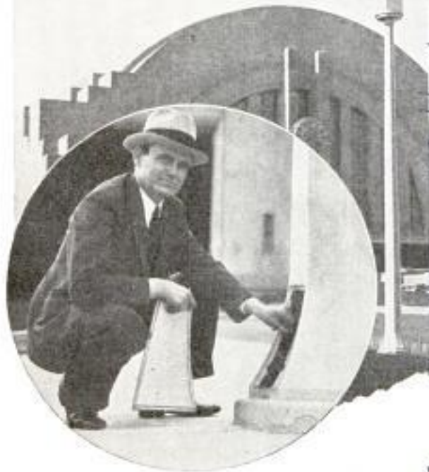
New Lighting Standards; Inset, View of Door Removed from No-Fuse Compartment in Base
