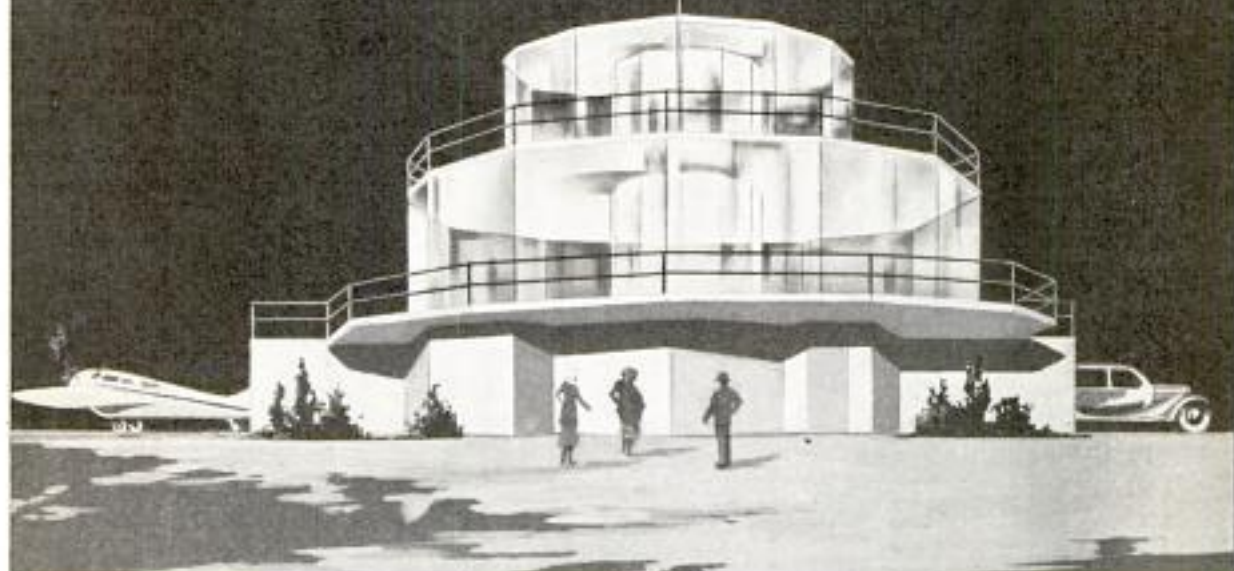
Walls of This House Are of Glass and Support No Weight; the Frame Consists of a Steel Mast Set in Concrete from Which Arms Radiate to Support Second Floor and Roof
