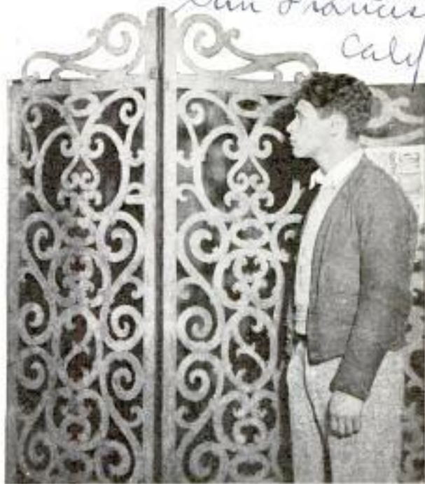
Grill of Scroll-sawed Wood Has Surfacing Treatment to Make It Appear Like Metal
