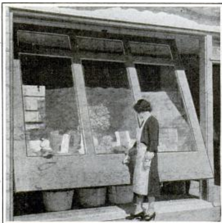
Disappearing Garage Door Which Forms an Attractive Shop Window When Lowered; It Can Be Raised by One Person
