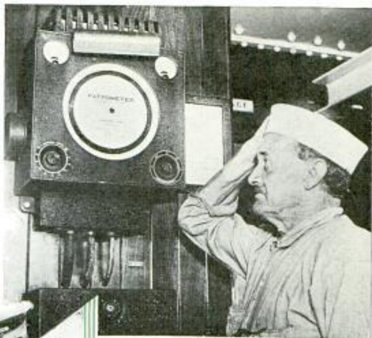
Top, Old Sailor Inspects Fathometer That Replaces Lead-Heaving in Determining Depth; Left, the "Mariposa's" Gyro-Compass Repeater and the Polaris
