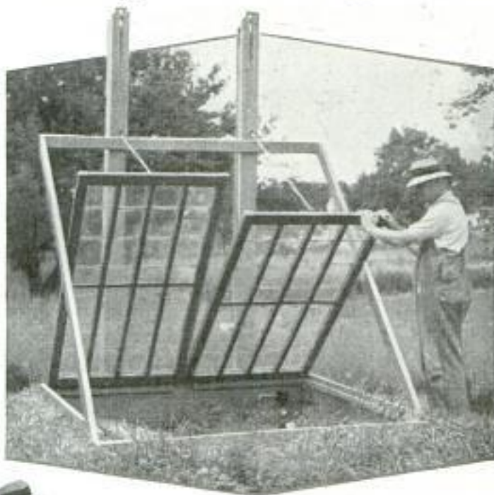
Hotbed Sash Is More Easily Handled by Using Counterweights That Slide in U-Shaped Posts Centered behind the Beds
