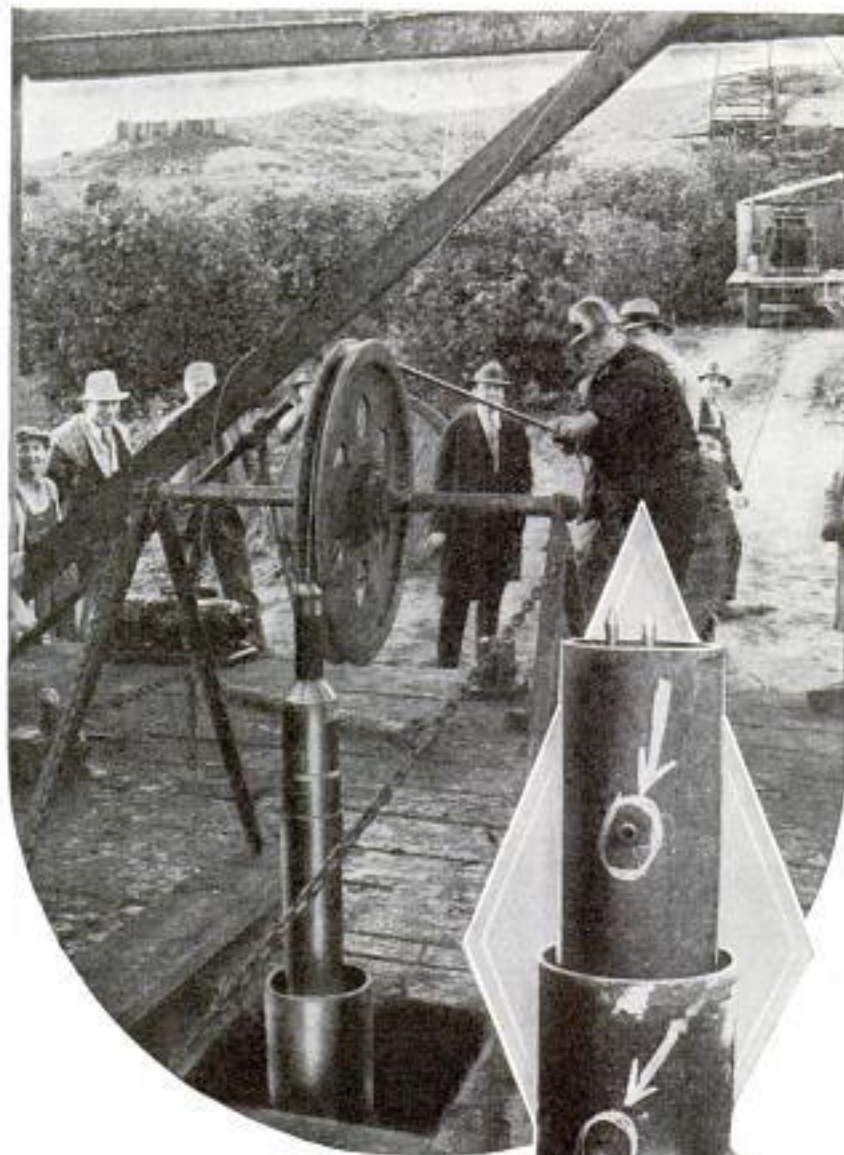
Top, Withdrawing Gun after Firing Charge Far Below Surface; Center, Bullet Holes in Four Casings Encircled in White; Bottom Diagram Shows How One Bullet Penetrated Four Casings
