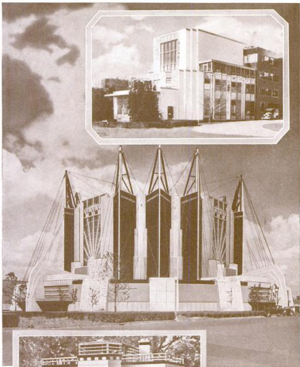
Top, Corner of Administration Building, a Striking Example of the New Methods of Building with Its Bolted Steel Frame, Walls of Asbestos Wallboard and Ground Newspapers and Cornstalks as Insulating Materials; Center, Transportation Building Which Has Roof Suspended by Cables; Left, Ferro-Enamel House, One of the Many Modern Homes Visitors Will See at the Exposition
