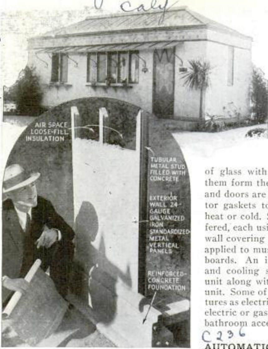
Top, Steel House; Bottom, Construction Features That Make It Easy to Heat or Cool
