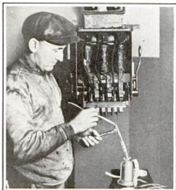
New-Style Gasoline Torch in Use; It Is Especially Adapted to Electrical Work
