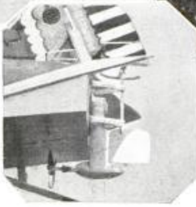
Views of Boat Built Like a Plane and Capable of High Speed; Note the Airplane Type of Rudder and the Wide, Flat Bottom Which Reduces Water Resistance
