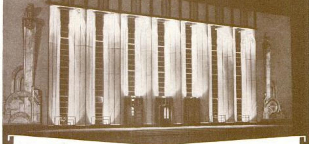
Night View of Front of Administration Building, Showing How Lighting Is to Be Used for Decoration; This Is One of the Few Permanent Structures Built for the Fair
