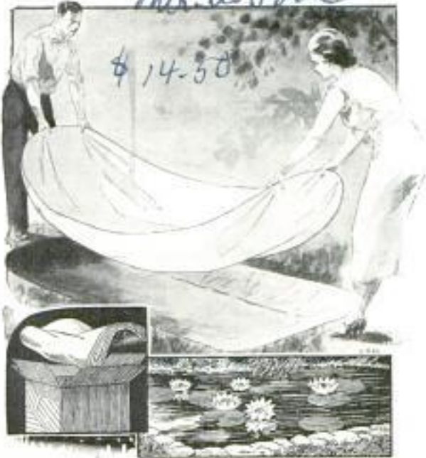
How Waterproof Lining Is Installed After Pool Has Been Dug in Garden or Yard
