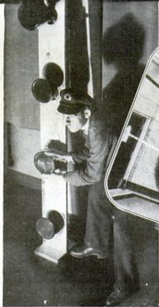
Left, the Invisible Rays Can Be Reflected by a Mirror, so Their Direction Can Be Altered at Will; Above, Line Indicates Path of Rays Guarding Bank Vault
