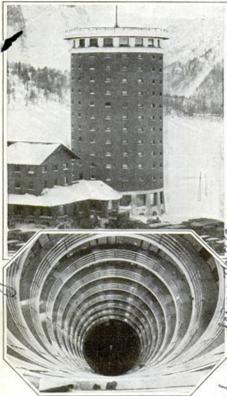
Top, Hotel Resembling Tower of Medieval Castle; Bottom, Looking Down the Well; Ramp Is Used Instead of Stairway
