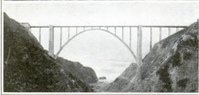
Successive Stages in Construction of Concrete-Arch Bridge on Roosevelt Highway; the 714-Foot Structure Has an Arch of 342 Feet and Carries the Roadway 270 Feet above the Ocean
