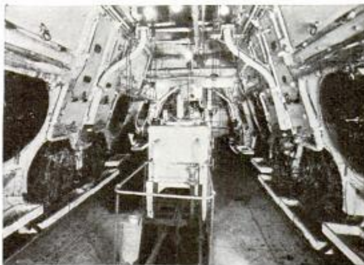
View of Part of the Boiler Room of the "Aquitania"
