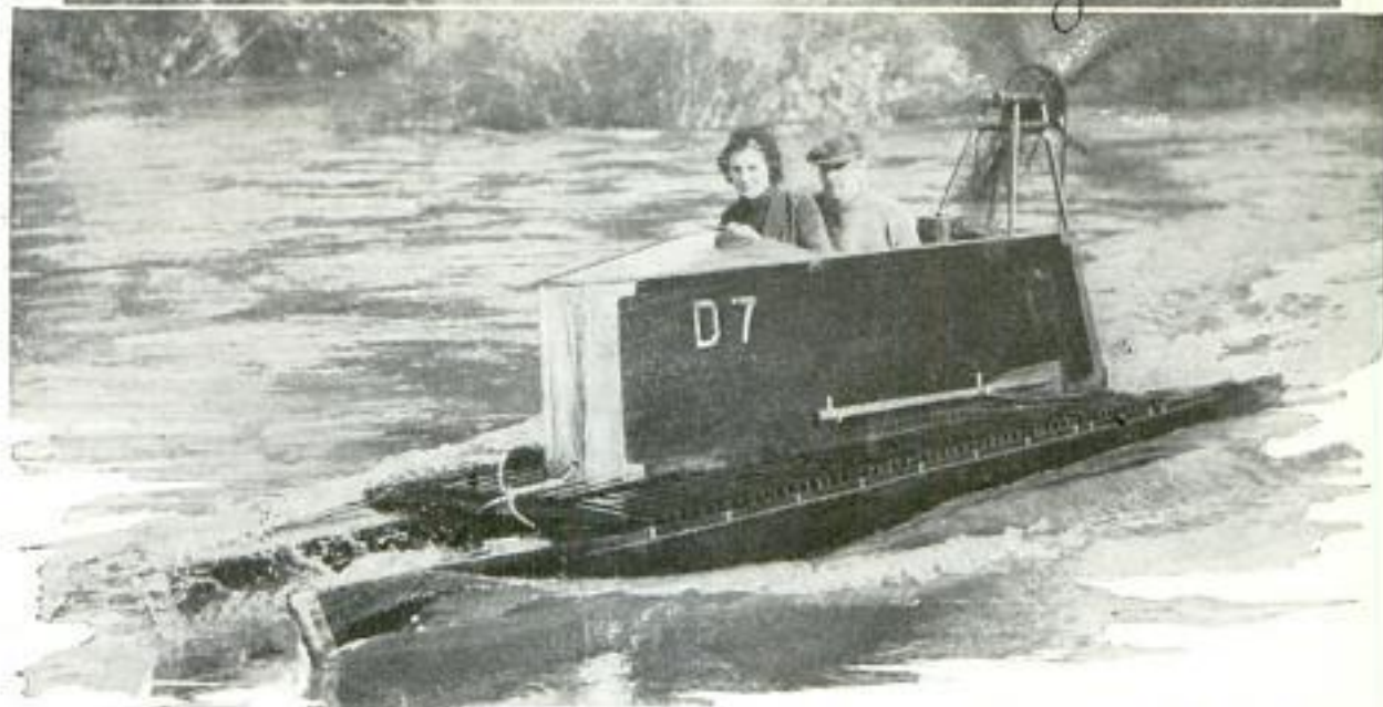
Boat for Use in Very Shallow Water; It Is Driven by an Air Propeller Powered by a Small Auto Engine
