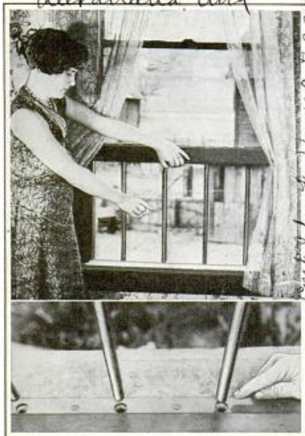
Bars Appear as Window Is Raised and Slide into Holes as Window Closes
