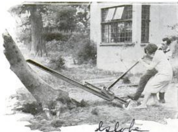
Jack with Long Leverage Which Pushes over Small Trees Easily
