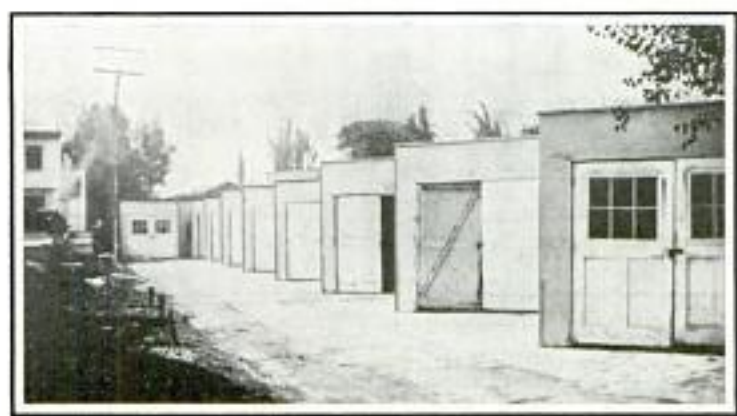
Nine Garages, Built at an Angle along a Narrow Alley, Permit Easy Access without Maneuvering the Cars
