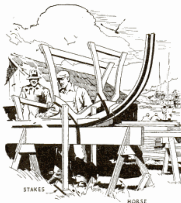
Stakes Driven into Ground Hold Struts and Frames Rigid When Building Boat Outdoors
