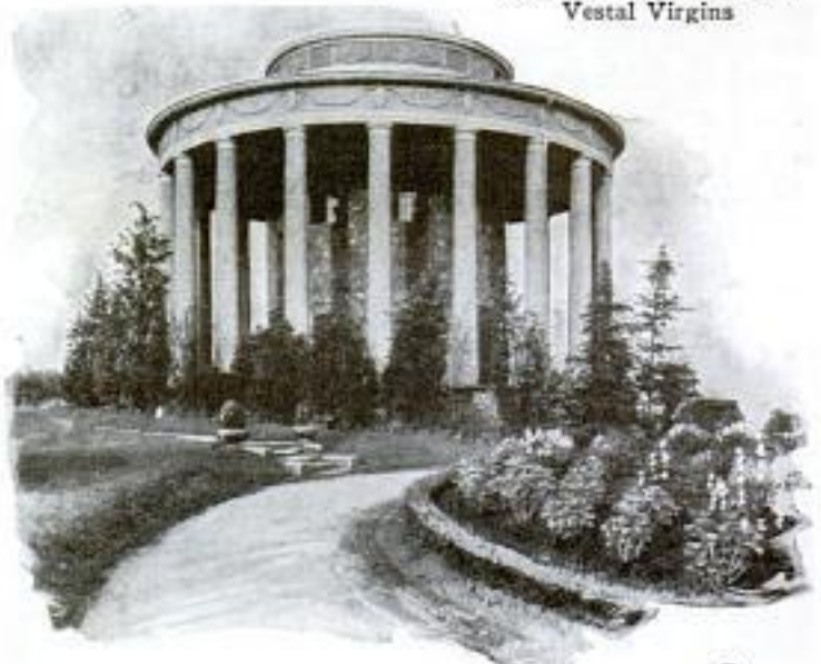
Home near Birmingham Modeled after the Ancient Temple of the Vestal Virgins
