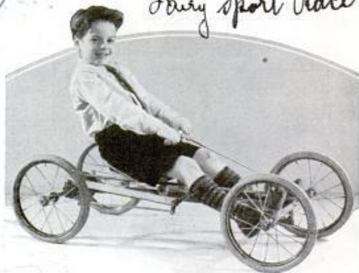
When the Rider Pulls Strap, Racer Moves Ahead and Free-Wheels While the Strap Is Rewound Automatically
