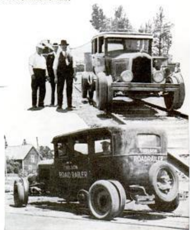
Auto with Flanged and Rubber Wheels Which Can Be Lowered and Raised for Rail or Highway Travel
