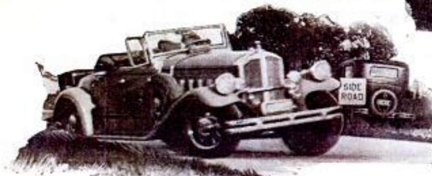
One Wheel off Pavement on a Soft Shoulder; the Driver Should "Float" Back on the Road without Trying to Apply Brakes
