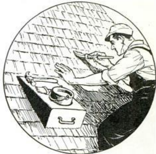
A Square Can, Cut in Two, Makes Holder for Bucket When Painting Roof
