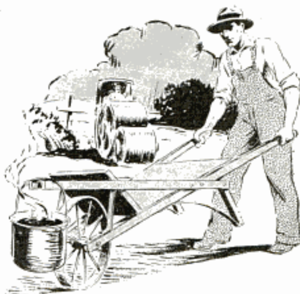
Wooden Arms Permit Hot Tar to Be Carried on Wheelbarrow without Splashing on Workmen
