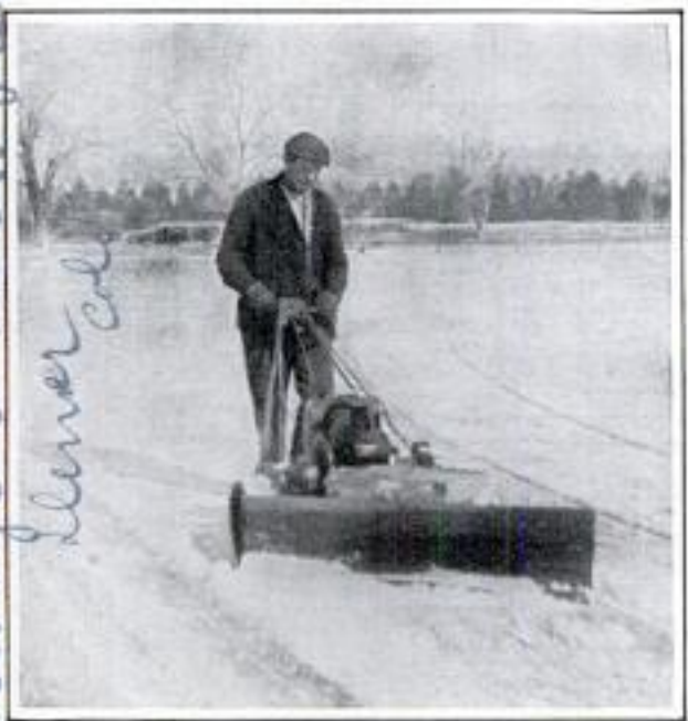
Instead of Being Stored in Winter, This Lawn Mower Pushes a Small Snowplow in Denver
