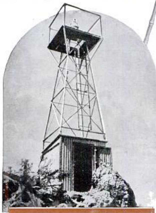
Top, Airway-Station Attendant Going down Mountain for Supplies; Below, Beacon Tower Whose Flashing Light Guides Pilot through the Night
