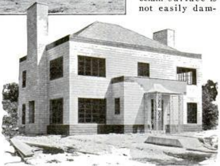
Top, the Window Casements Are Made of Steel; Center, the Structural-Steel Framework; Below, the Porcelain-Steel House Almost Completed
