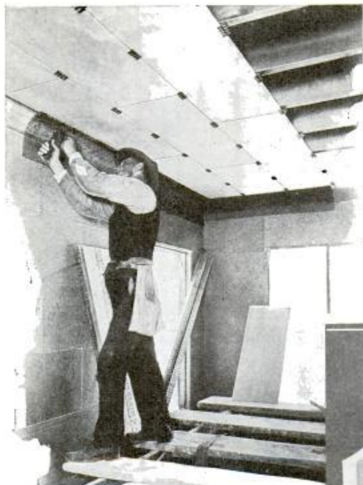
Above, Ceiling Suspended on Springs to Deaden Sound; Right, Close-Up of Spring Construction
