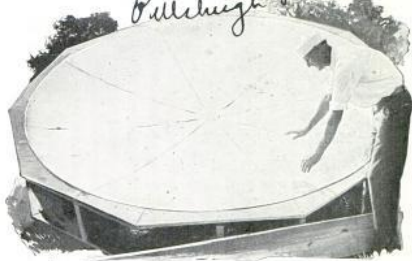
Solar Furnace Capable of Producing a Temperature of 5,000 Degrees; Heat from the Sun Is Focused Seven Feet above the Furnace
