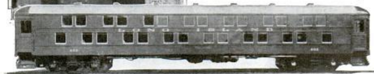
Double-Deck Railway Coach Which Seats 120 Passengers; It Contains One Center Aisle from Which Passengers Step Up or Down to Reach the Top or Lower Tiers of Seats
