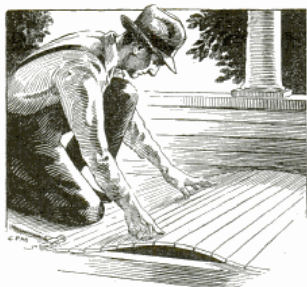
Tongue-and-Groove Boards Pressed into Place to Make Tight Porch Floor
