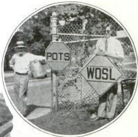
Left, Viewing Highway Sign through a Shutter Momentarily Opened to Determine Type with Best Visibility; Right, Some of the Signs Tested; Note the Scrambled Letters
