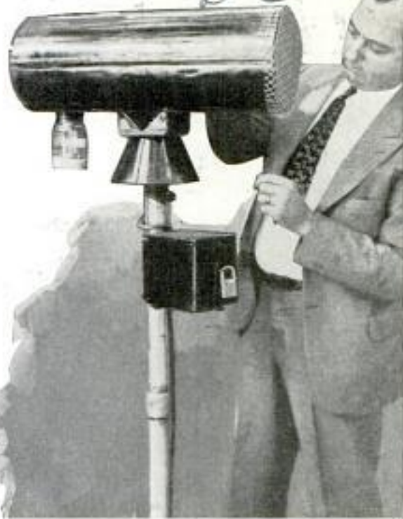
Insect Trap with Electric Light to Attract the Pests and a Fan to Draw Them Inside
