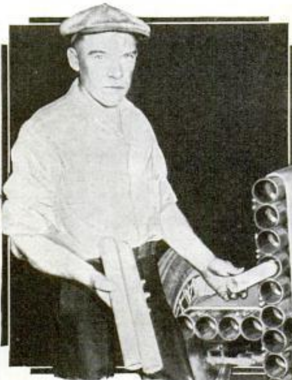
Sig Haugdahl, Veteran Race Driver, with His Rocket-Powered Race Car; the Rocket Tubes Are Located along the Sides and below the Body and May Be Discharged Independently
