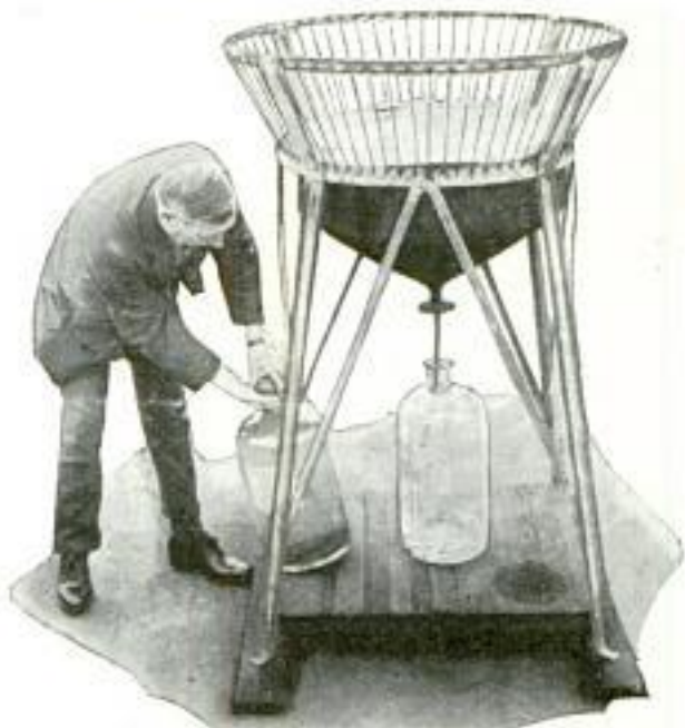
Observer Removing One Month's Catch from Soot-and-Dust Gauge in London
