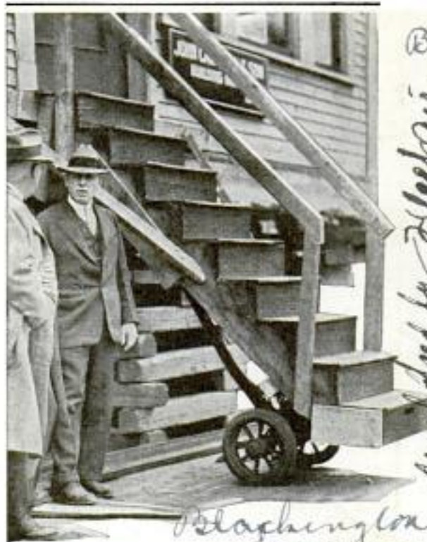
This Stairway on Wheels Rolled Along as Building Was Moved, Avoiding Interruption of Business
