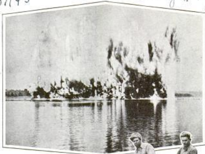
Right, Cable to Which Dynamite Is Attached Is Shown Being Laid in River; Top, Water Hurling into the Air When Explosive Digs Trench on the River Bottom for a Pipe Line
