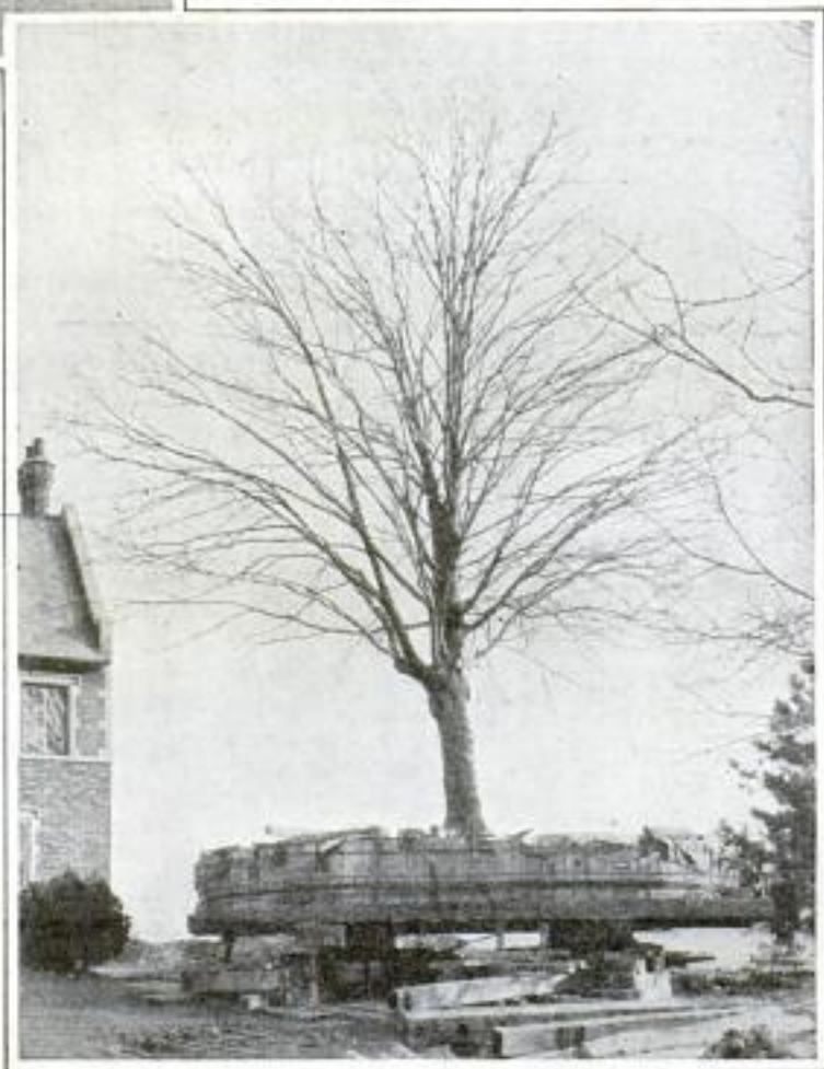
Right. Sixty-Foot Tree Being Moved on Rollers to a New Location, Shown Above
