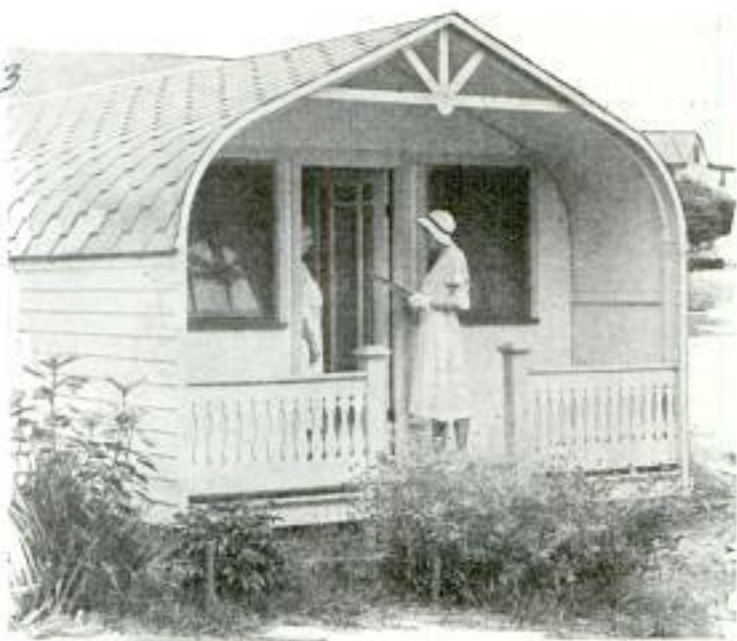
Form of Arch Roof Construction Intended to Lower Building Costs; the Walls Extend into the Roof
