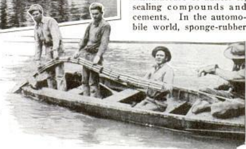
Right, Cable to Which Dynamite Is Attached Is Shown Being Laid in River; Top, Water Hurling into the Air When Explosive Digs Trench on the River Bottom for a Pipe Line
