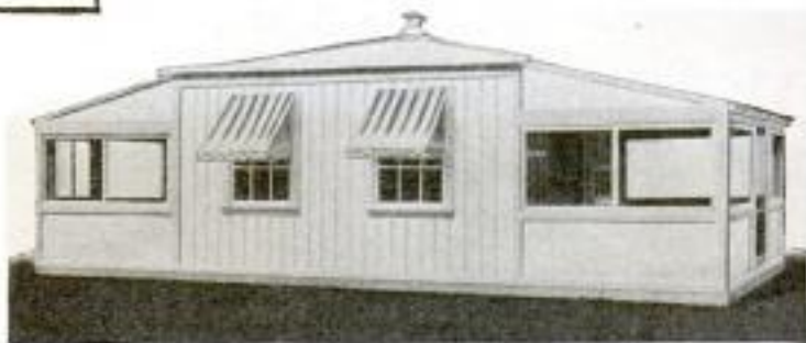
Two Workmen Set Up This Factory-Made Metal Home in a Single Day (Continued to page 138A)
