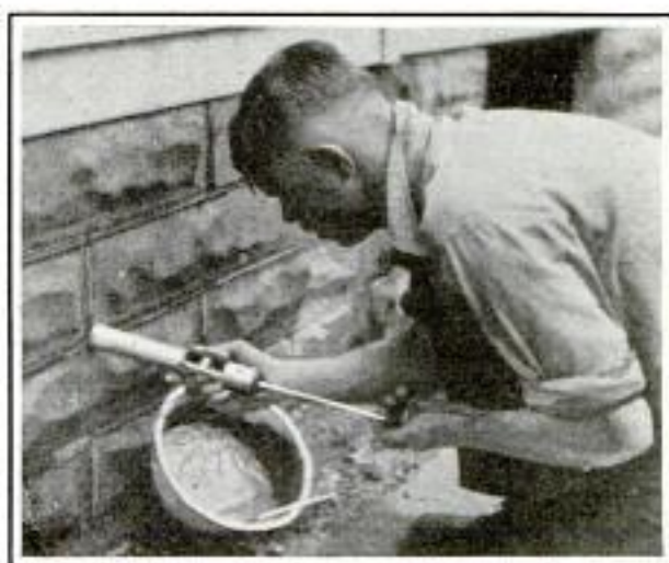
Cement Forced into Cracks with Altered Spray Gun
