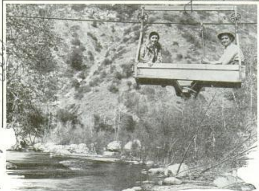
This Form of Rail-Car Is in Use Where a Bridge Was Washed Out; It Is Pulled by Strap Iron Shown Hanging from the Cable
