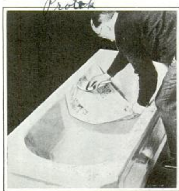
Newspapers to Protect Enamel Fixtures from Damage Are Held in Place by Paste
