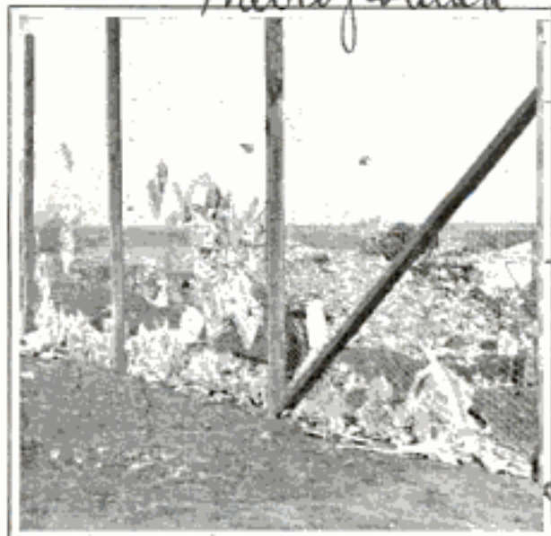
Wire Fence Erected between an Airport and a Dumping Location to Keep Refuse Off Landing Field
