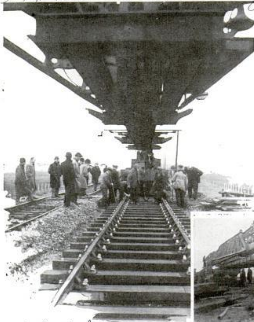
Wide World Above, Workmen Bolting Sections of Track Together; Right, Track Layer Deposits Another Section
