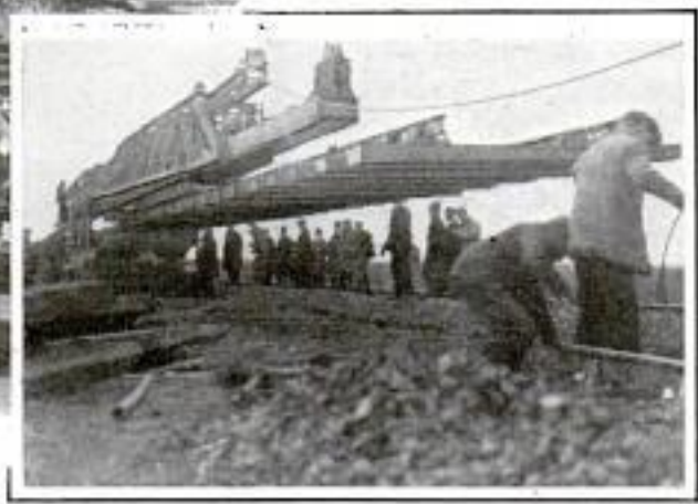
Wide World Above, Workmen Bolting Sections of Track Together; Right, Track Layer Deposits Another Section
