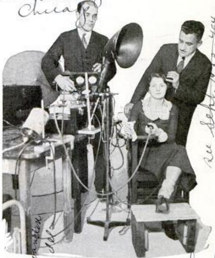
This Sleep-Inducer, with Its Low Hum, Makes the Subject Drowsy; Note the Recorders Attached to Arms, Legs and Head
