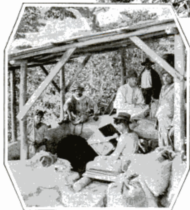
Top, Mill of Coffee Plantation with Pipe Line at Left; Below, Loading Station at Head of Line
