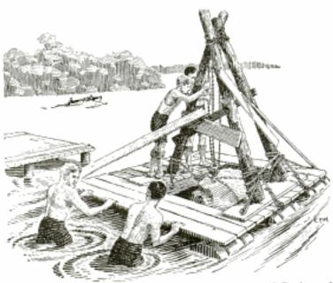
Oil-Drum Raft Fitted with Hoist to Raise Submerged Rocks and Move Them to Deep Water
