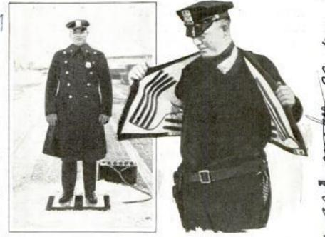
Vest and Shoes for Traffic Officers Which Are Heated by Electricity When the Policeman Stands on Metal Plate Connected to Battery
