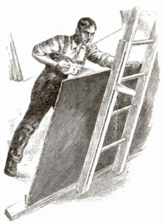
Strip of Wood Nailed to Side of Ladder Serves as Guide for Sawing Wallhoard
