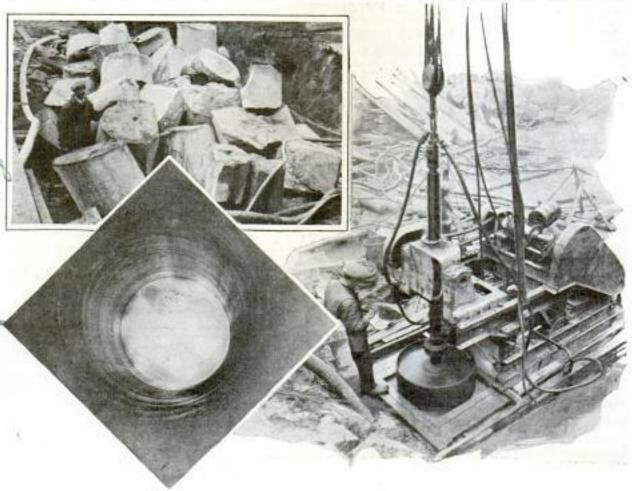
Top Left, Some Rock Cores Removed from Holes for Orchestra Elevator Shafts: Bottom Left, Looking Down One of the 42-Foot Holes; Right, Electric Drill Begins Job of Cutting Shaft in Solid Rock
