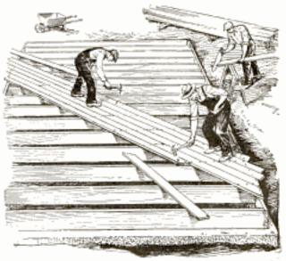
Starting Board Nailed Diagonally across Joists in Center of Room Permits Working Both Ways
