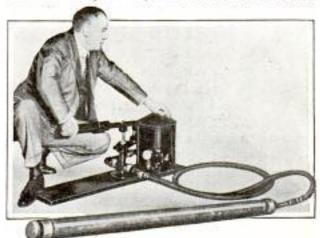
Hand-Operated Pump Forces Water through Bomb, against Coal in Safer Mining
