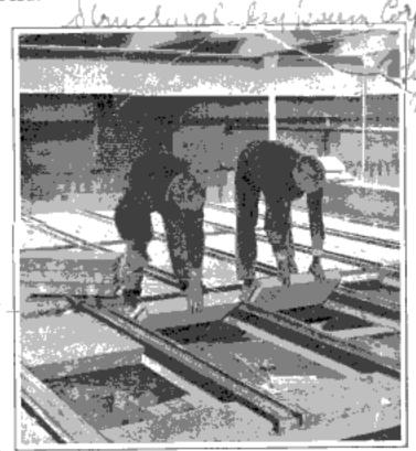
Laying Slabs of Gypsum on Steel Beams Preparatory to Pouring Concrete on Top to Form a Fireproof Floor
