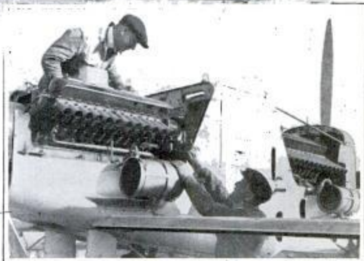
The "Do-X" in "Drydock" for Overhauling at Long Island, Above, and, at Right, Reinstalling the Engines After the Power Had Been Increased
