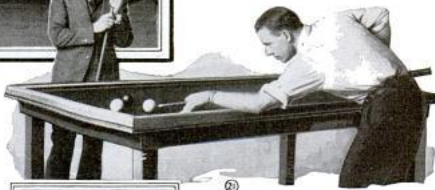
Simple Billiard Table Having a Wooden Bank Provided with a Length of Rubber Tubing Tacked On to Serve as Rebounding Strip; Pockets May Be Added or the Bank May Be Removable for Ping Pong
