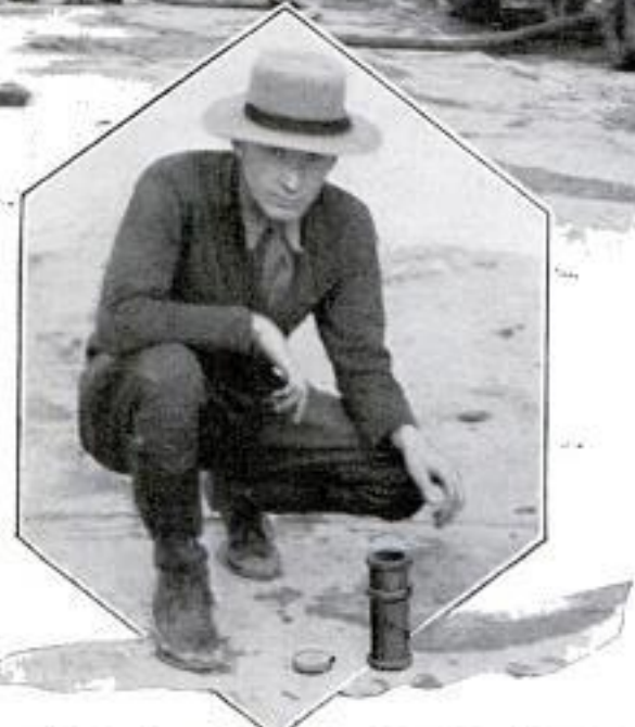
Center, Mudjack at Work; Top, Hose Nozzle beside Hole in Pavement; Below, Pipe Cast in Road to Receive Hose
