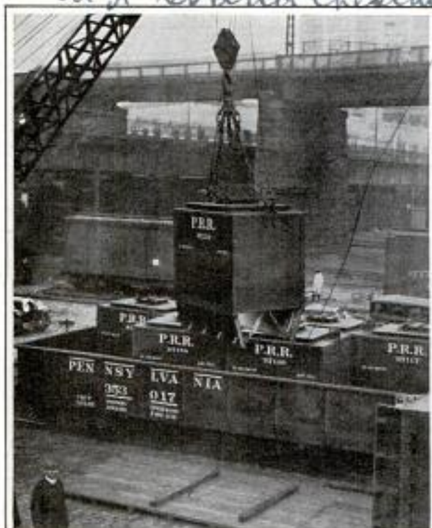
These Steel Containers for Freight Are Carried at Low Rates by One U. S. Railroad
