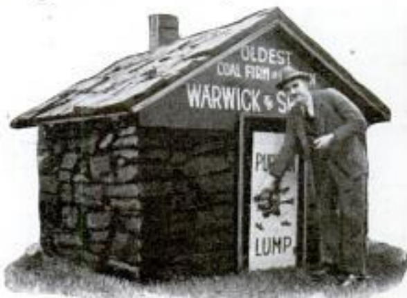
The Only Wood Used in This House Made of Coal Was in the Roof Frame and Door
