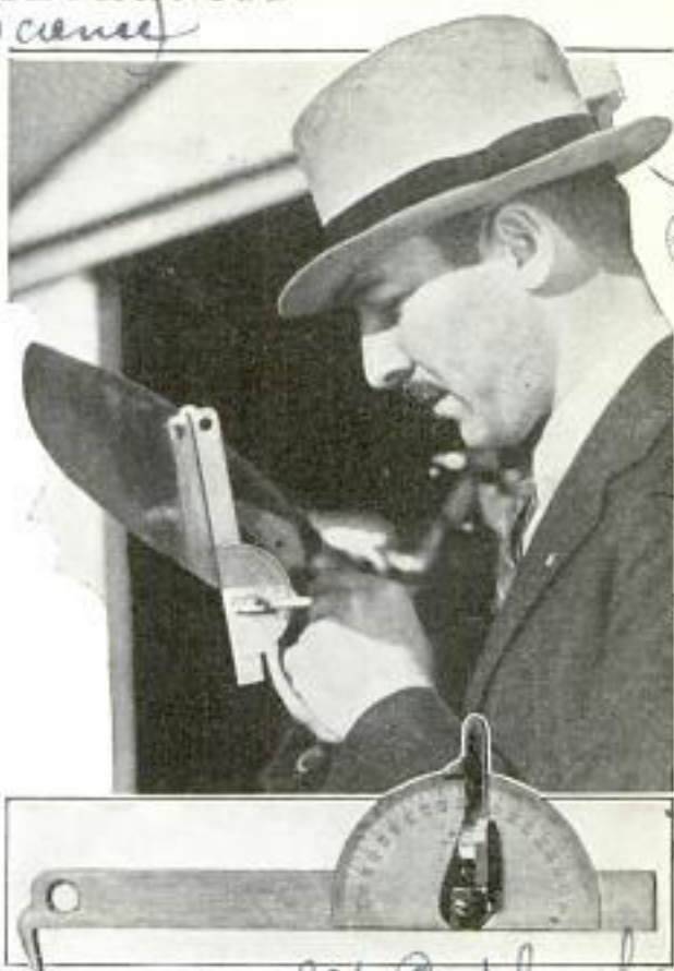
Courtesy C. LaTour, 7806 Ardleigh St. Propeller-Pitch Gauge in Use, Above, and Below, a View of the Time and Money Saver
