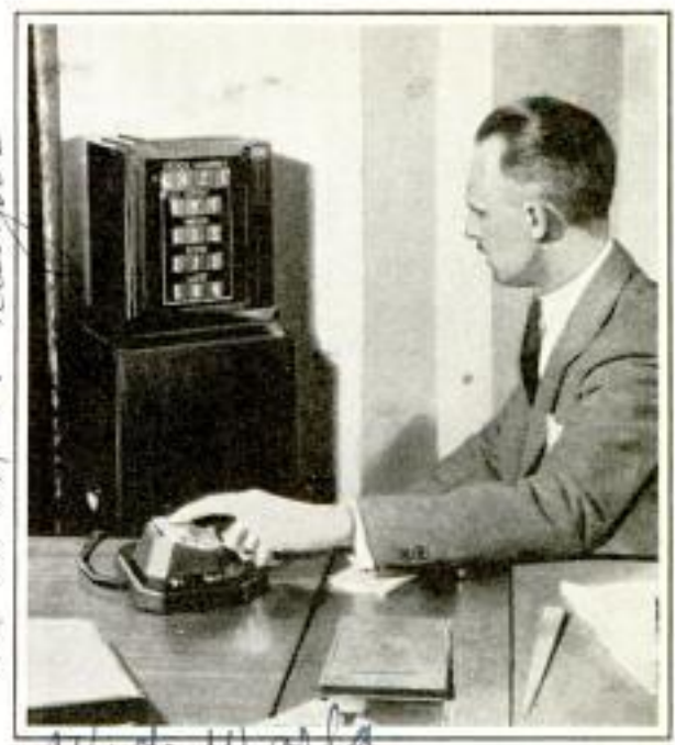
Dialing the Number of a Stock Will Bring Latest Prices on Private Office Registers Now in Use
