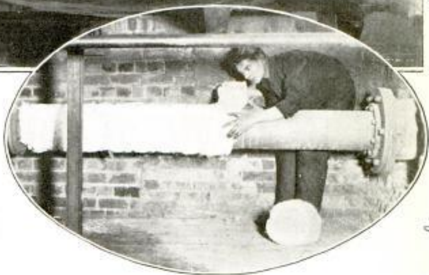
Glass as Fine as Silk Is Good Insulation; Above, Spinning Glass; Below, Pipe Being Wrapped with This Non-Conductor Material
