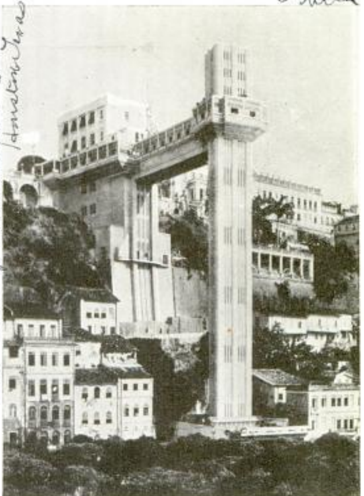
Elevator Tower Built in Bahia, Brazil, to Transport the City's Population from Lower to Upper Level
