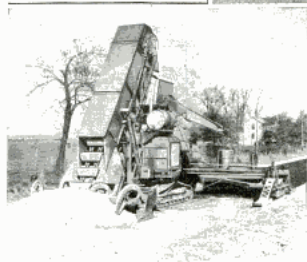
Rear and Front View of Machine That Paves Whole Road Width in One Operation without Forms
