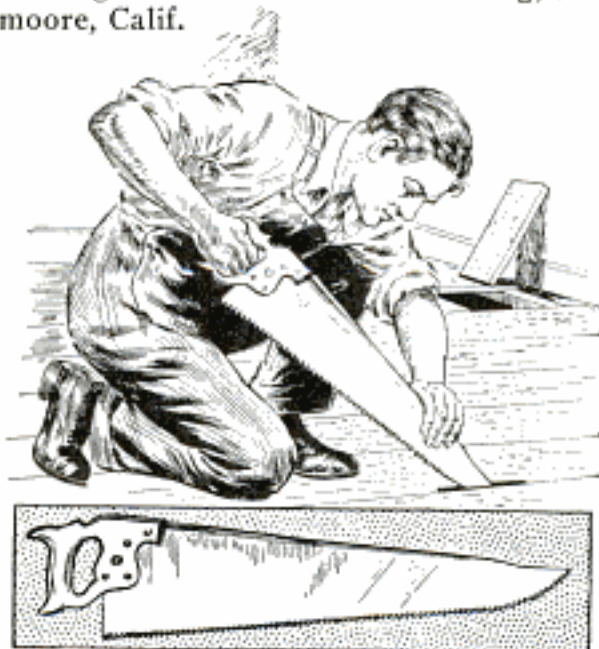
Rounding End of Handsaw Provides Means of Removing Flooring without Damage to Surrounding Surface
