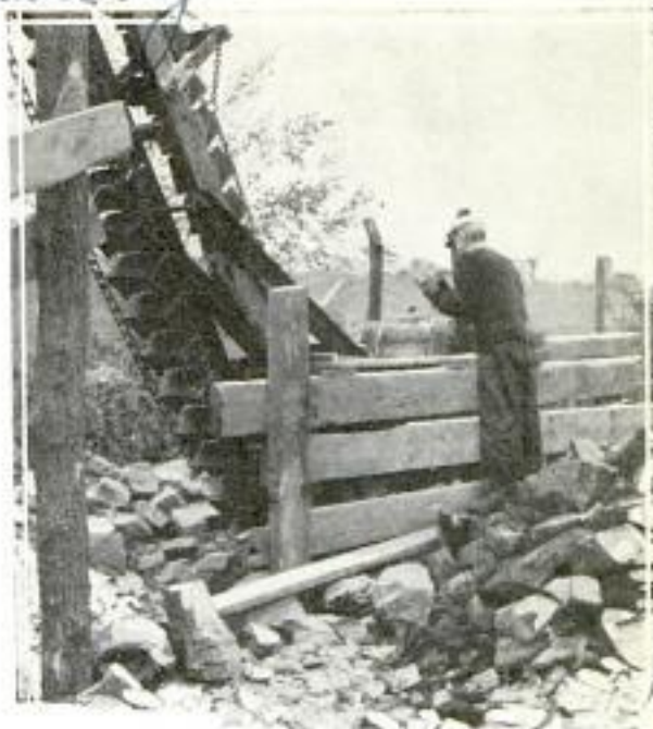
By Crushing Stone Fences, Material for Paving Rural Roads Was Obtained by One Contractor
