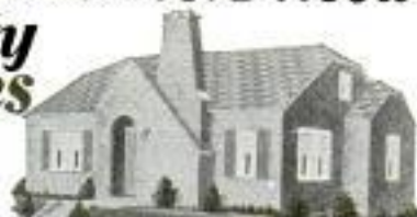
4 to 9 Room Homes
