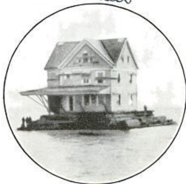
© International News Photo Moving a Frame House across a River; the Dwelling Was Loaded on a Barge and Floated
