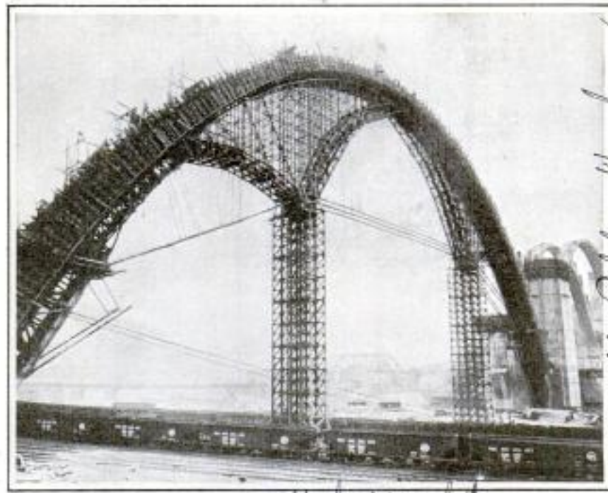
Central Arch of New Westinghouse Bridge, Which Will Shorten Autoists' Time Between Pittsburgh and the East
