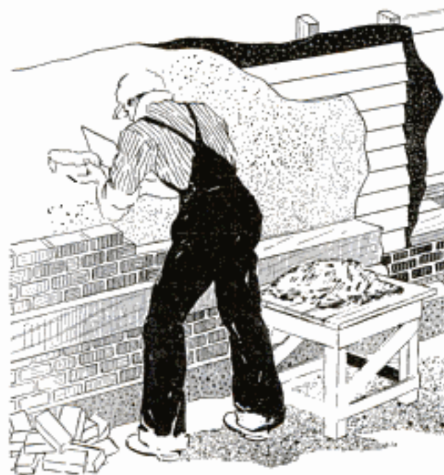
Old Homes Made Modern by Clothing Them with a Coat of Brick, Half-Timbering and Stucco, Which Also Improves Insulation
