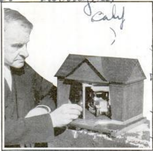
Backing Your Car Out Is Unnecessary if the Garage Has Turntable
