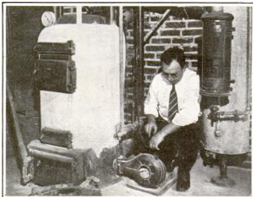
Electric Blower for the Furnace Which Creates Forced Draft and Enables Use of Cheaper Coal
