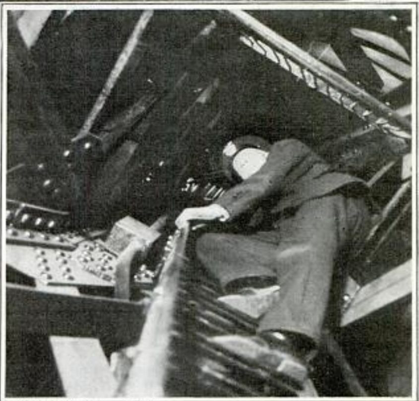
Top Photo by U. S. Army Air Corps Above, Aerial Photo of Statue Made at Night by Glare from Flashlight Bomb; Below, Guard Climbing Inside of Arm to Torch
