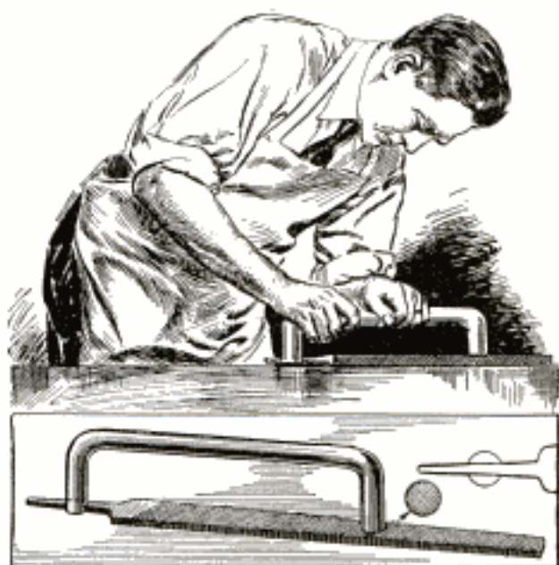
This Handle, Fitted to Tang of File, Insures Firm Grip When Surfacing Flat Work
