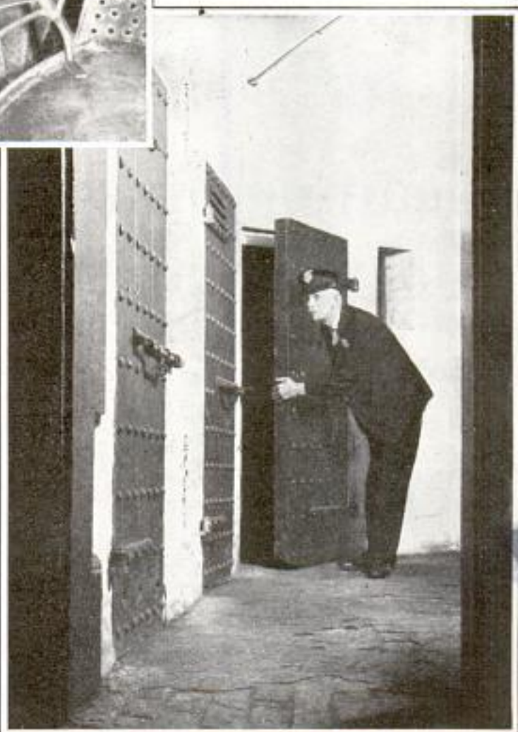
Above, 115-Foot Spiral Stair Leading to Head of Statue; Below, Mystery Prison Found beneath the Figure
