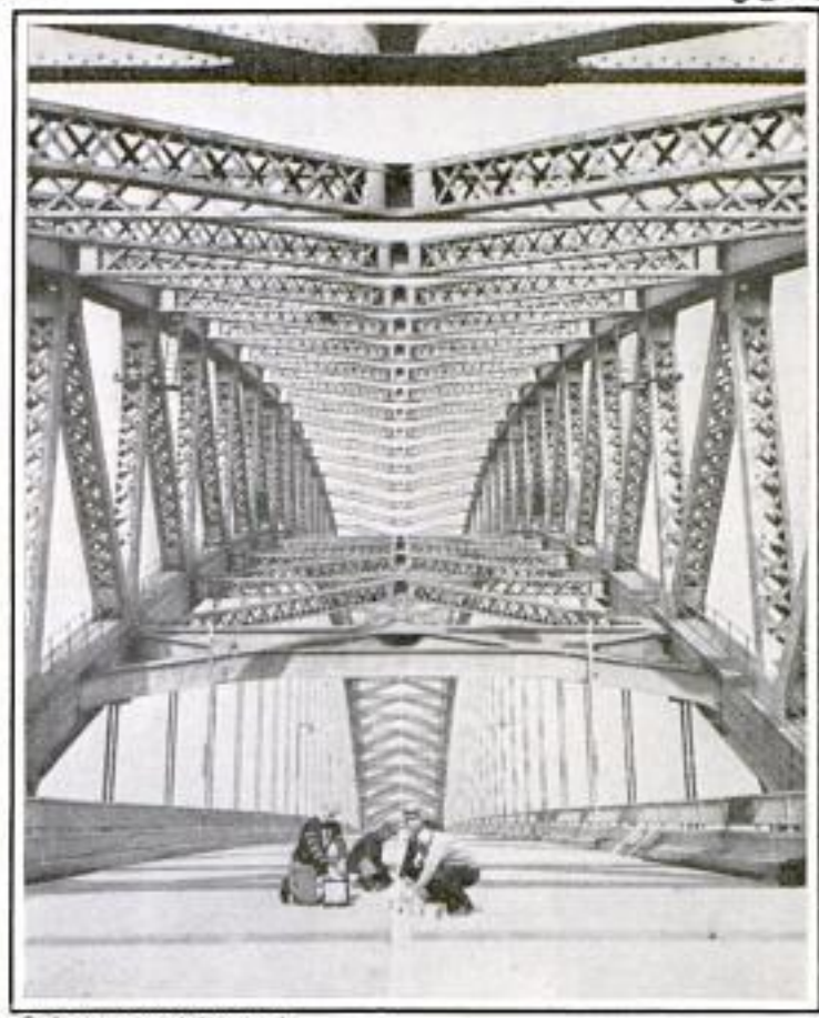
© International Newsreel A Section of the 1,675-Foot Arch Span of the Kill Van Kull Bridge, Linking Staten Island with New Jersey
