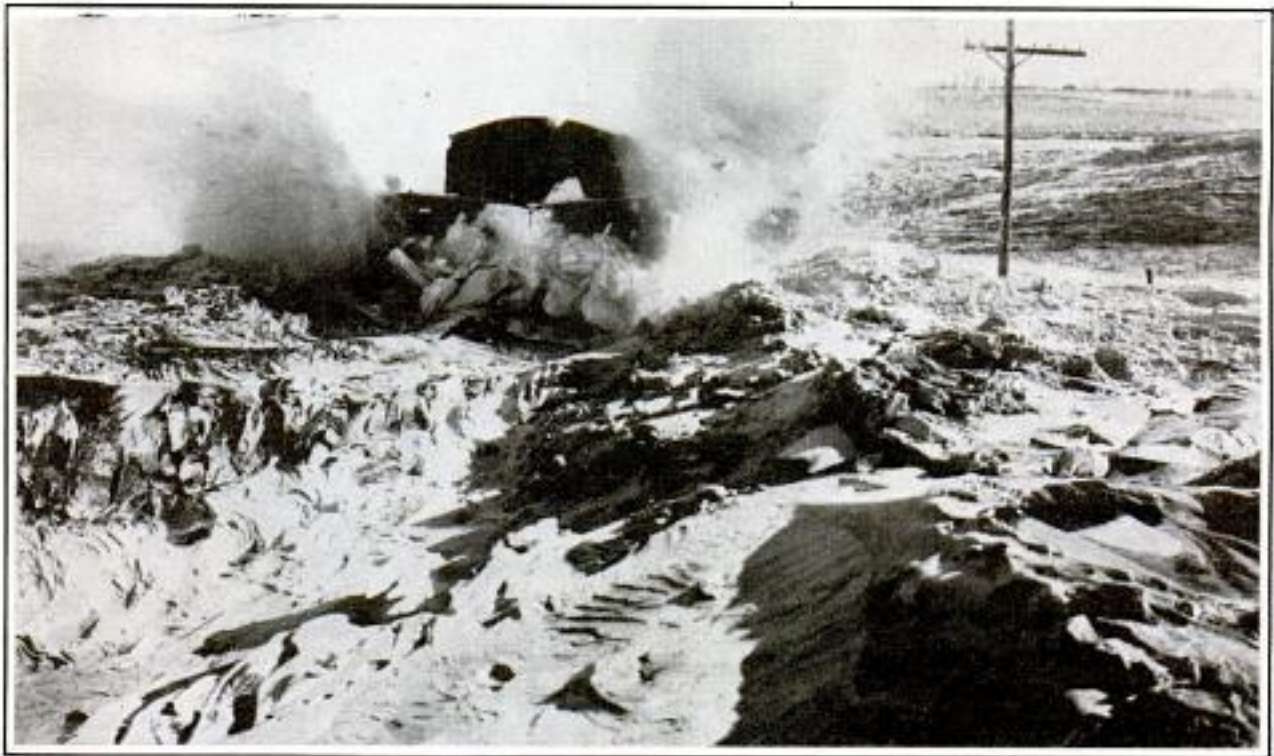
Here Is the Way a Snow-Blocked Road in South Dakota Looks After the Flakes Have Quit Coming Down; the Highway Is Being Opened by a Tractor and a Rotary Plow
