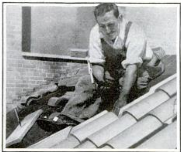
Weighing One-Tenth of Other Roofing Materials, Bakelite Is Used as Waterproof Covering
