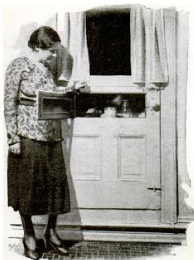
Box Fitted to Outside of Door with Hinged Panel Provides Convenient Cooler
