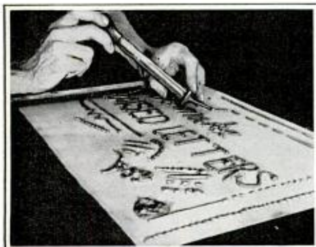
Raised Lettering on Show Cards and Display Signs Formed by Squeezing Paste through Hydrometer
