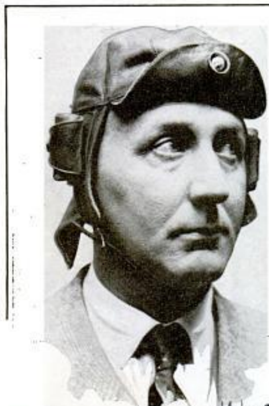
Flyer's Helmet with a Light in the Visor for Reading Maps; Batteries Are in the Ear Rolls
