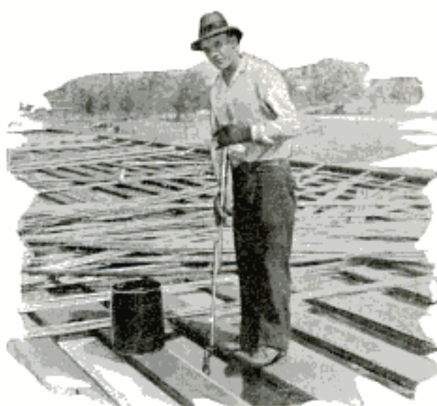
Painters Can Stand Erect When Painting Flat Surfaces by Using This Extension Handle
