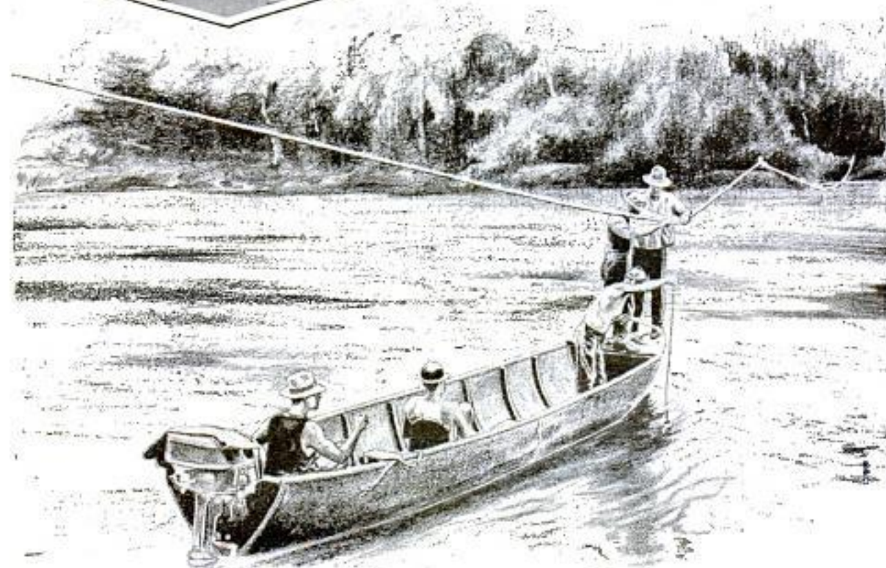
Suspension Bridge across River at Camp Deakne, Top; Sounding the San Juan River Was Accomplished by Hanging onto Ropes Stretched across the Stream
