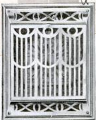
Electric Heater, Set into the Wall. Shown Above, Is Turned On and Off Automatically by Time-Control Clock Just above Wall Grill
