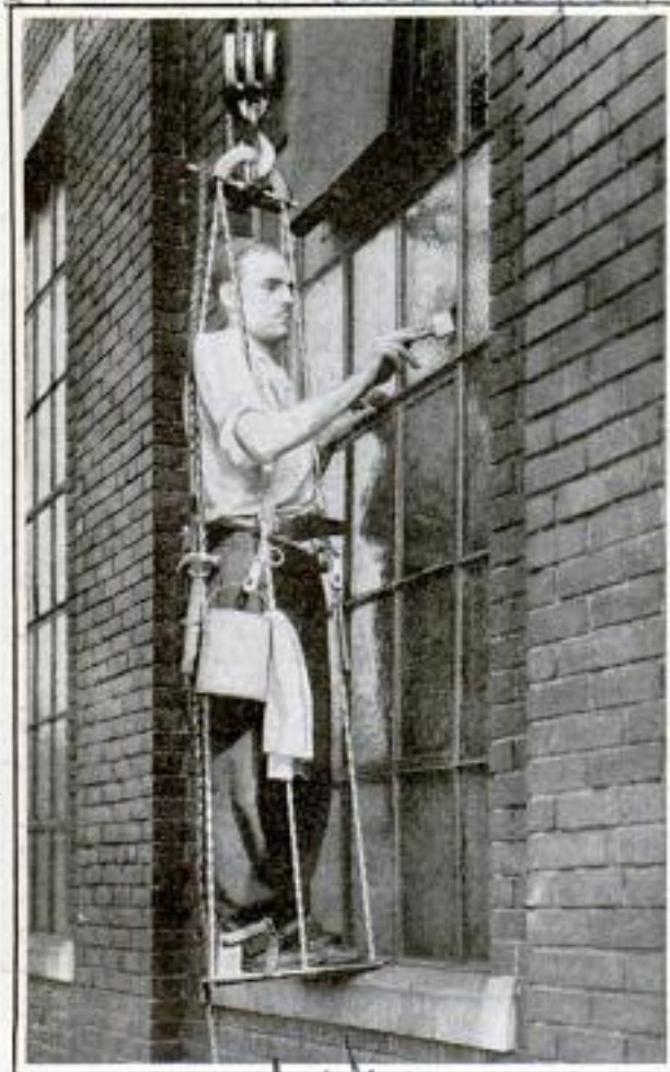
Aerial Stand for Window Washers and Painters; Note How the Feet Are Strapped to Base
