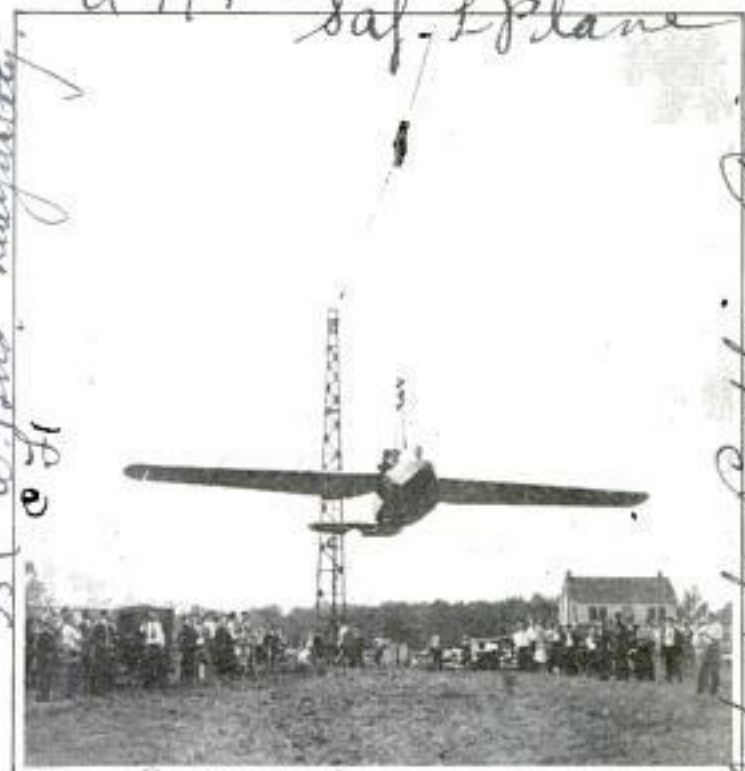
Crashes of Student Planes Are Eliminated by Suspending the Training Ship from a 1,000-Foot Cable
