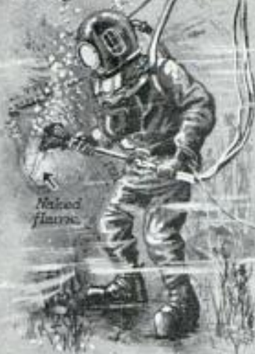
Using an Oxy Acetylene Cutting Torch under Water.
