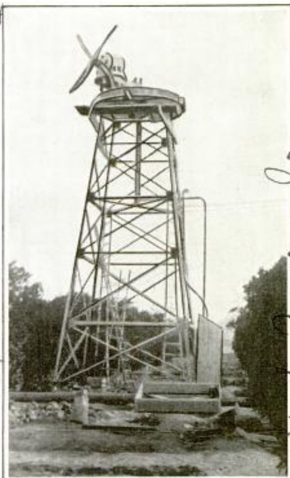
Warm Air, Drawn from Above, Is Fanned over Fruit Trees to Guard against Frost
