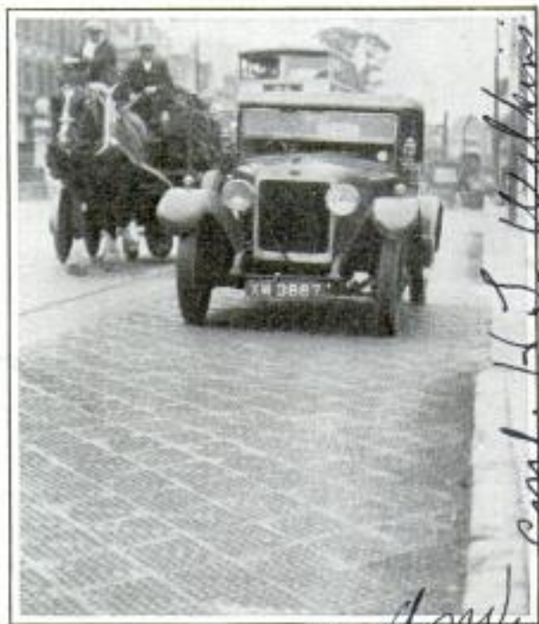
London Street Surfaced with Slabs of Cast Iron to Resist the Wear of Heavy Traffic
