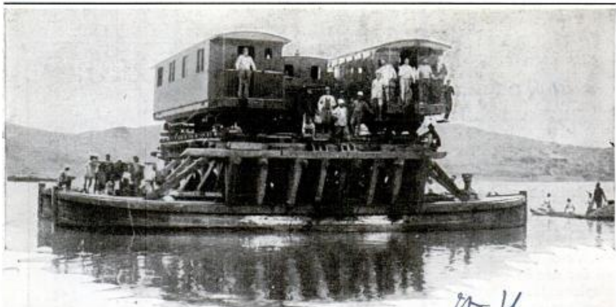
Elevated Ferry Made by Lashing Two Boats Together and Building a Superstructure on Which Trains Can Be Run in Sections from the Level of the Bank
