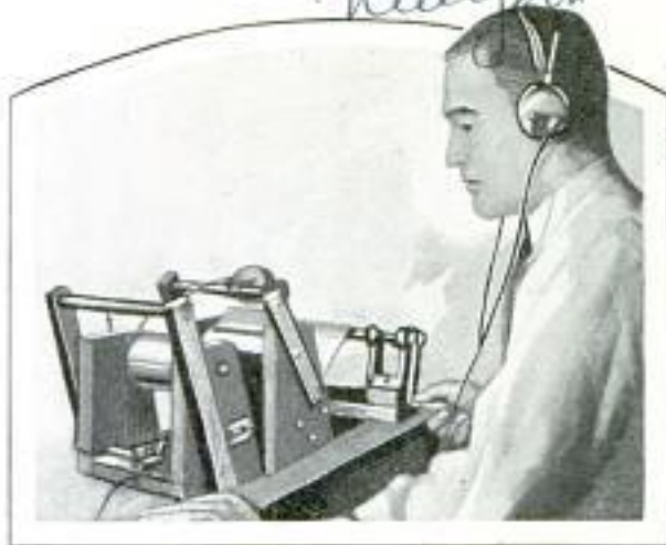
Listening for Metallic Specks Imbedded in Condenser Insulating Paper
