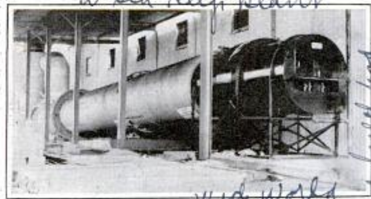
Dehydrating Plant That Turns Seaweed, or Kelp, into the Finest Flour at Temperature of 1,200 Degrees
