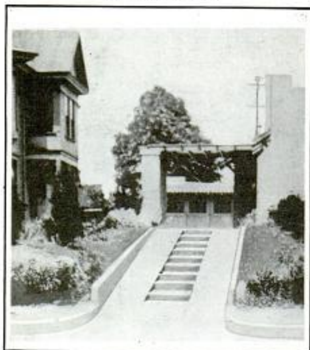
Steps May Be Combined with an Auto Ramp on a Sloping Lawn Without Sacrificing Space
