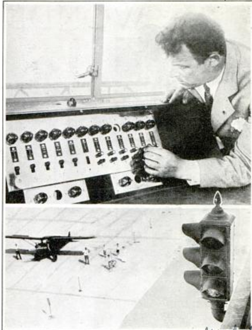
Traffic Signal for Airport Like Ordinary Stop-and-Go Street Light, and Control Board from Which Airport Lights Are Operated
