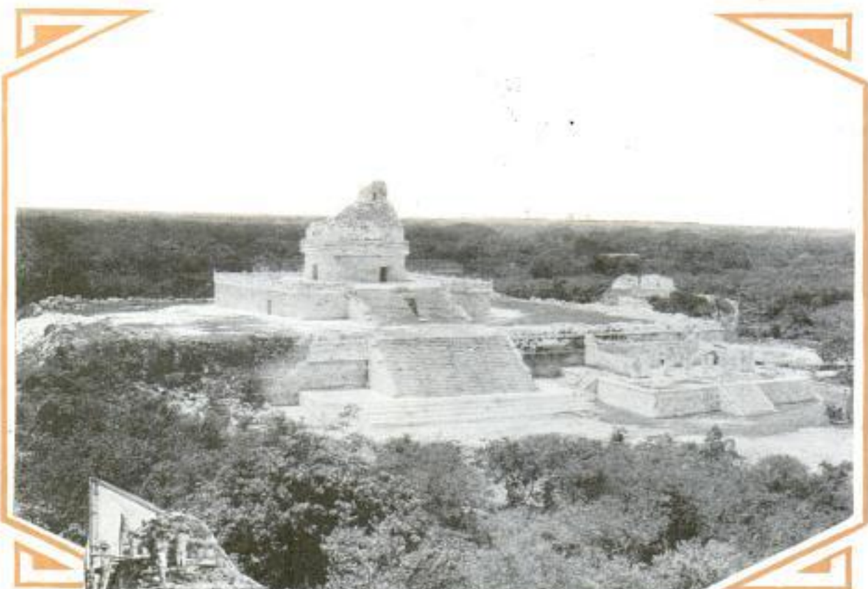
Older Structures Have Been Discovered Beneath Previously Restored Maya Edifices; Note Two Levels in Photo Above; Digging a Temple Out of a Bush-Covered Hill, at Left
