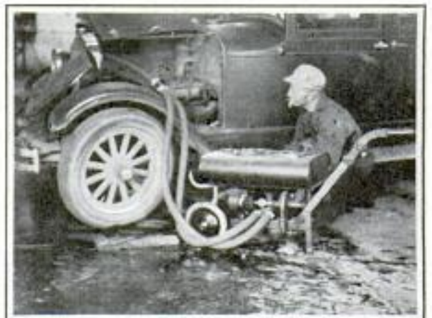
Automatic Flusher Containing Chemical Compound Which Removes Rust from Auto Radiators
