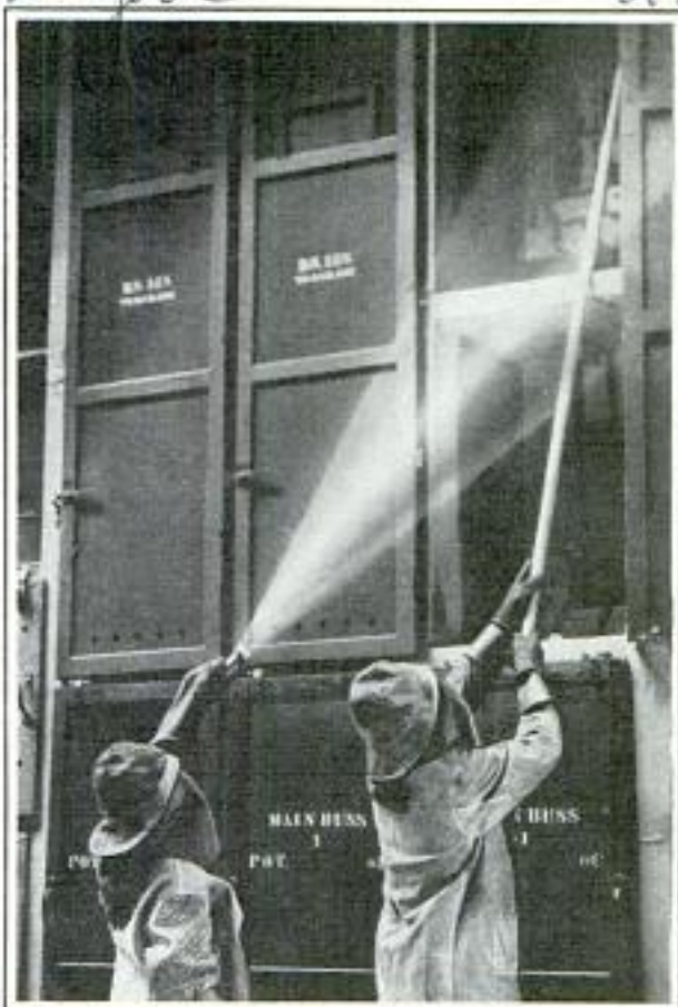
Courtesy Union Gas & Electric Co. Operating High-Voltage Switches While Protected from the Flash by Leather Suits
