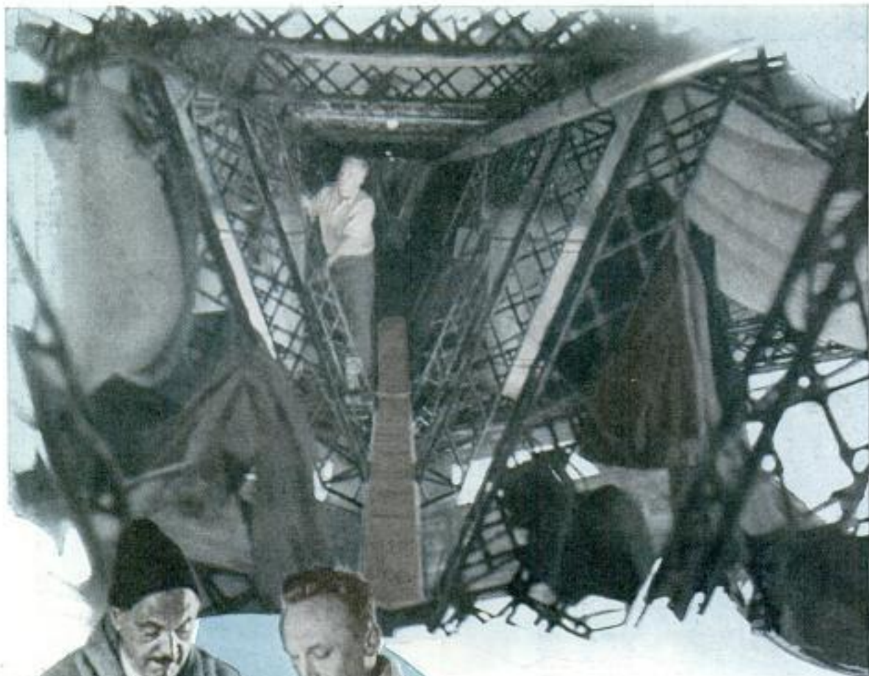
The Above View of the Catwalk of the "Graf Zeppelin" Indicates the Great Size of the Interior and the Crew's and Passengers' Means of Travel from Cabin to Cabin
