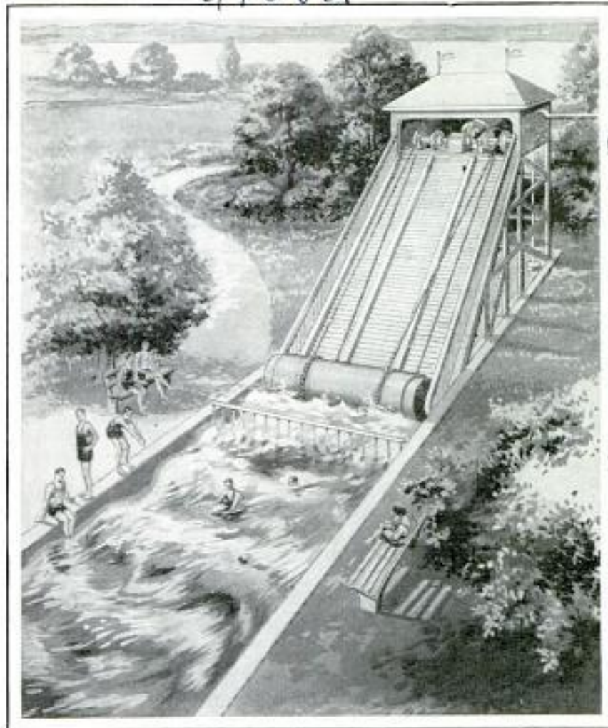
Drawing of Surf Machine to Provide Artificial Ocean Waves for Swimming Pools; the Big Roller Is Operated by an Electric Motor
