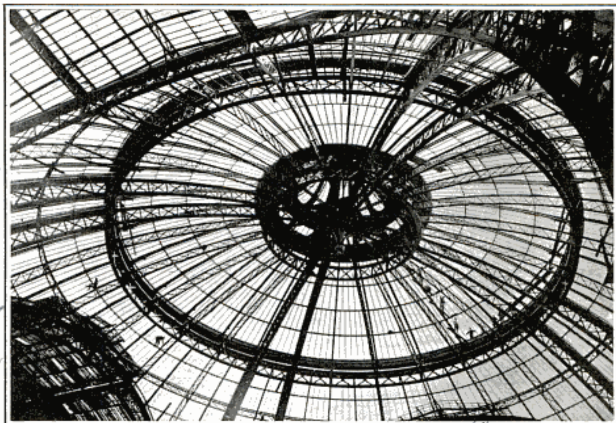
Workmen, Engaged in Re-Covering the Grand Palais, Paris, with a Network of Steel and Glass, Look Like Flies Caught in a Giant Spider's Web; the Roof Is 150 Feet High
