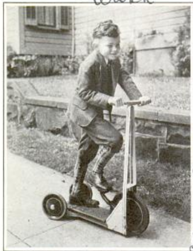
Free-Wheeling Scooter with Pedal Operating a Ratchet Device Which Permits Coasting
