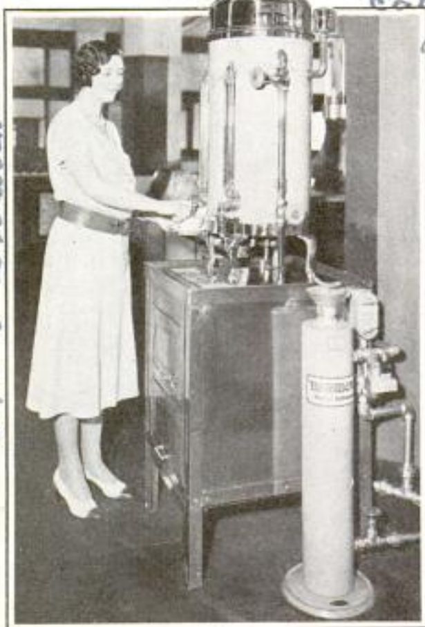
Water Softener Helps to Reduce Costs of Operating Coffee Urn by Removing Minerals
