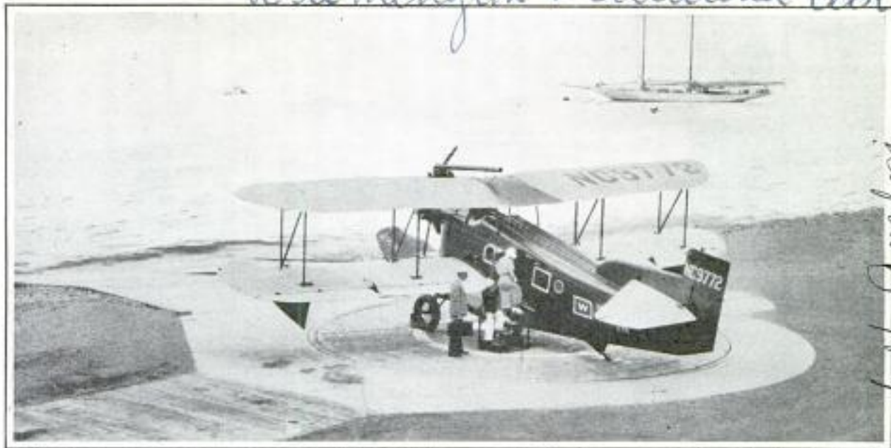
Electrically Operated Turntable for Amphibian Airplanes at a Beach Airport on Catalina Island; the Beach Is Too Small for the Planes to Be Turned without Its Use
