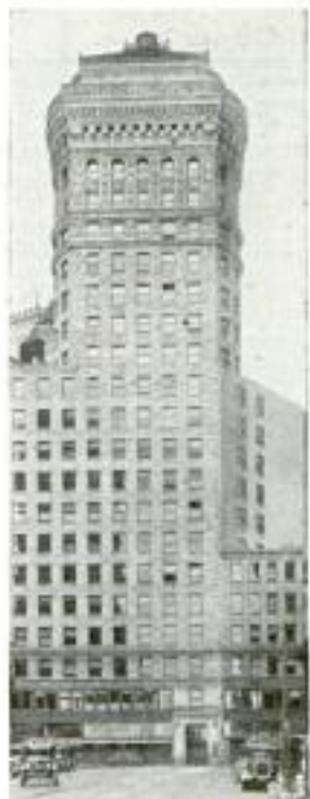
Our San Francisco Office Suite 1010 Hobart Building
