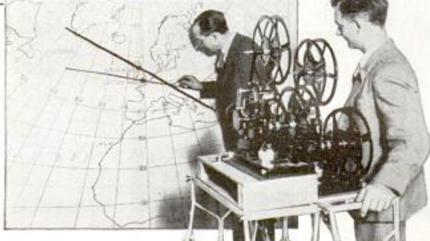
"Pictures" of Storms Are Taken with Machine Above; Right, Picture Projected onto Map to Locate Storm
