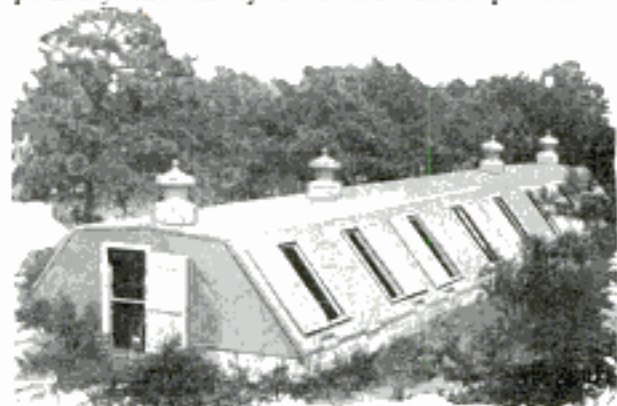
Poultry House with Slanting Walls Allows Sunshine to Reach All Parts of the Floor
