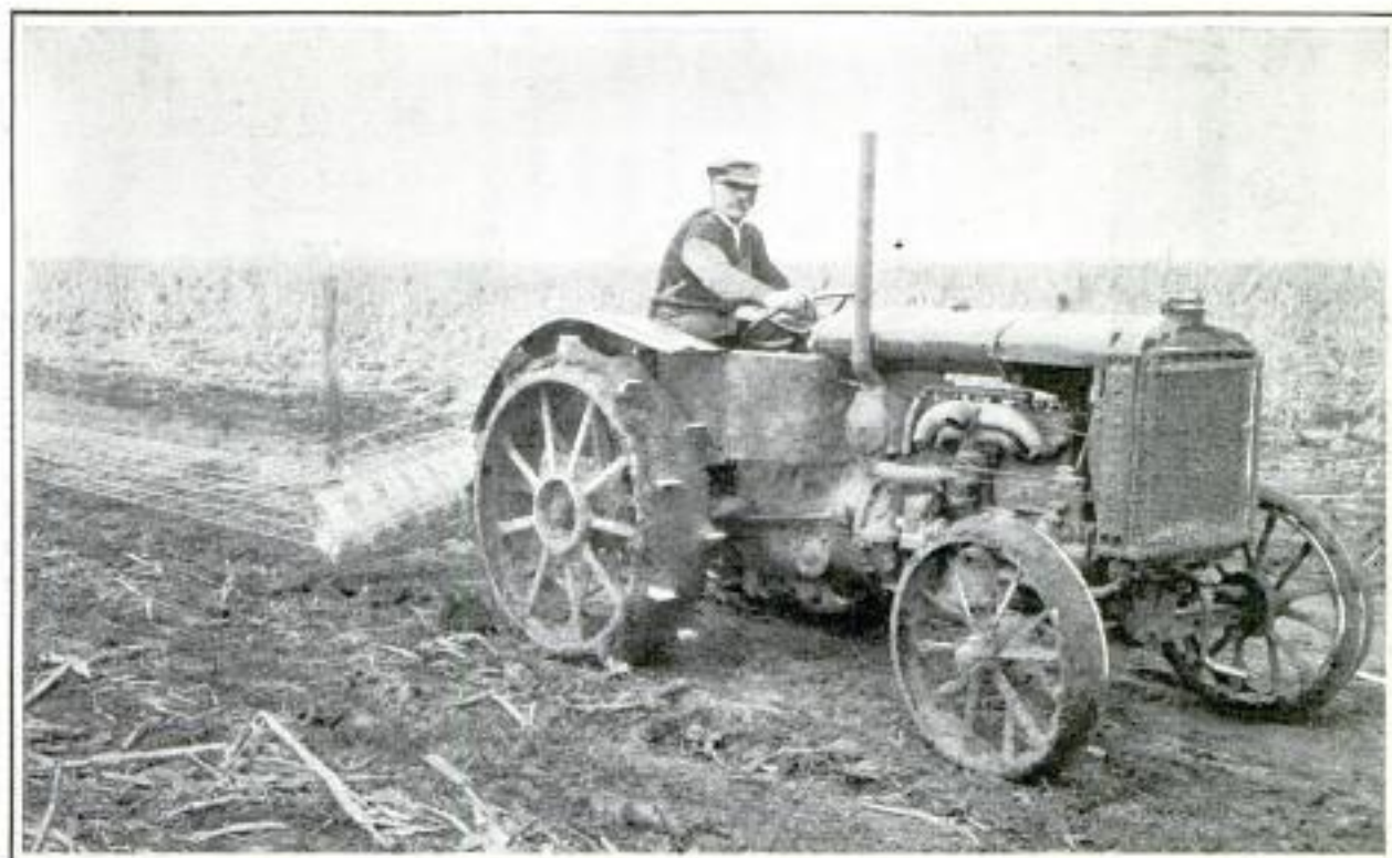
Using Your Tractor to Hold Woven-Wire Fencing Taut While Stapling It to Posts at Regular Intervals, Makes a Neat and Sturdy Fence besides Saving Time and Work
