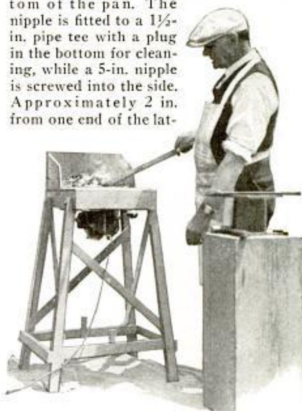
Vacuum-Cleaner Motor Provides Draft of Air, the Volume of Which Can Be Controlled
