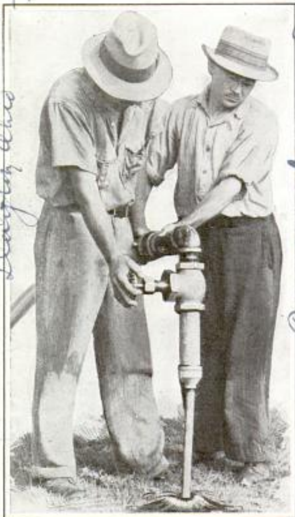
Water Pressure from Long Nozzle Is Digging a Hole to Water Roots of Trees
