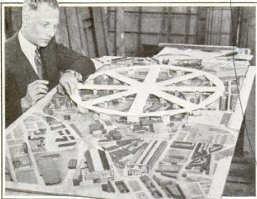
Model of Proposed London Airdrome to Be Constructed over Two Railway Stations; Note the Wheel-Shaped Design Suggested by the Architect
