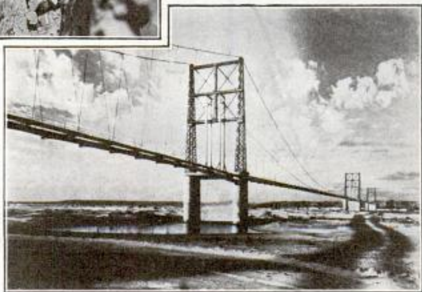
Difficulties of Pipe-Laying in the Blue Ridge, at Top; Bridge, 2,522 Feet Long, Built Only to Carry Pipe in Texas
