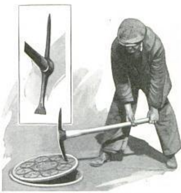
Pickax Properly Shaped Enables One to Remove Manhole Covers Single-Handed
