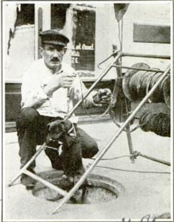
"Lion" Being Lowered in a Manhole to Draw a Brush through the Drain to the Next One
