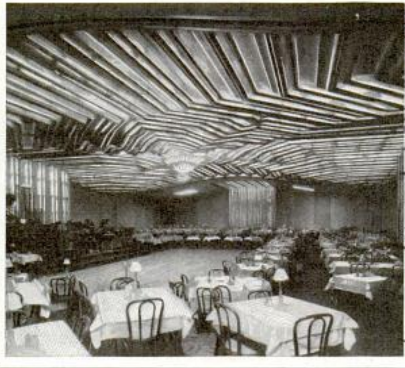
Sheet-Metal Ceiling Illuminated by Hidden Lights Which Make It Appear Like Colored Glass of a Modernistic Pattern
