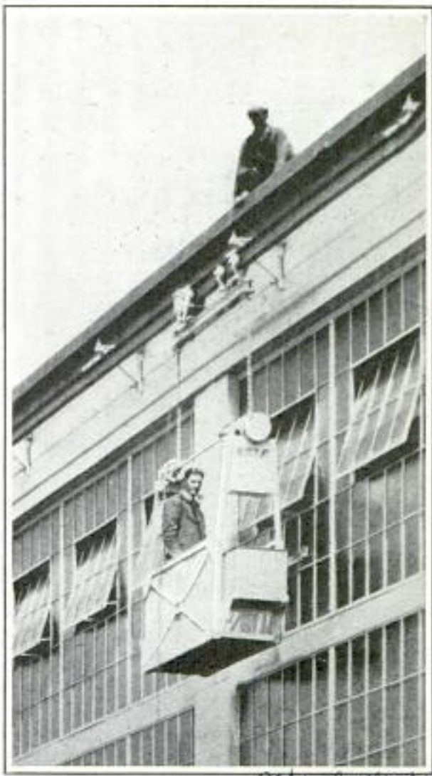
Window Cleaners "Take the Trolley" around Huge Building to Wash 30,000 Panes of Glass
