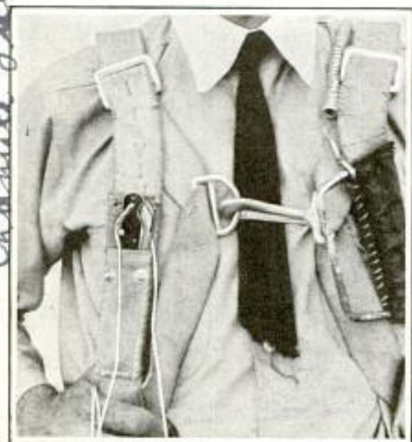
Parachute Harness Equipped with Safety Knife to Enable Jumper to Free Himself in Emergency
