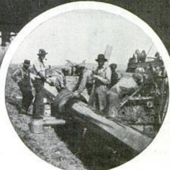
Photo by Ewing Galloway Oil Derricks at Night Reflected in the Sump; Right, Burning Tires Heat Pipe for a Bend
