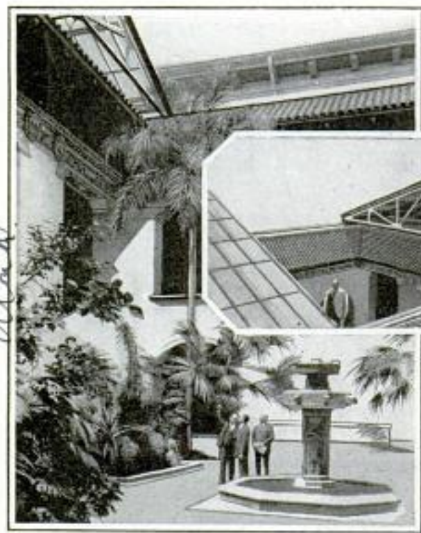
Tropical Garden Covered by Sliding Skylight, and Inset, How the Roof Rolls on Wheels
