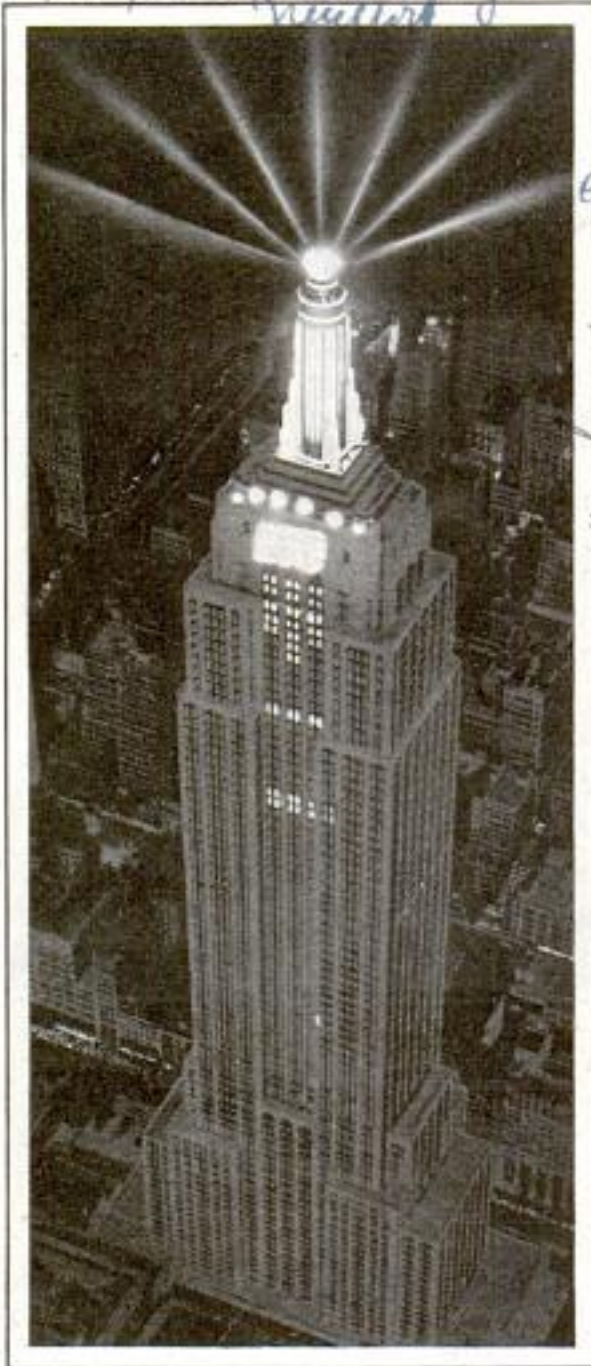
Lighthouse on Empire State Building Is 1,200 Feet above the Street and Can Be Seen for Fifty Miles
