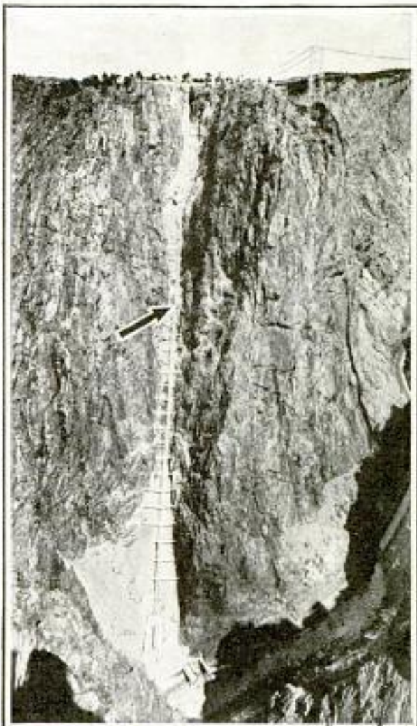
View of World's Steepest Railway, Which Is Built up the Side of the Royal Gorge
