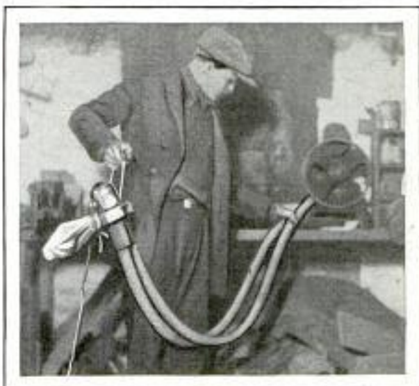
Old Vacuum Cleaner, Provided with Flexible Hose, Salt Bag and Handle, Cleans the Shop
