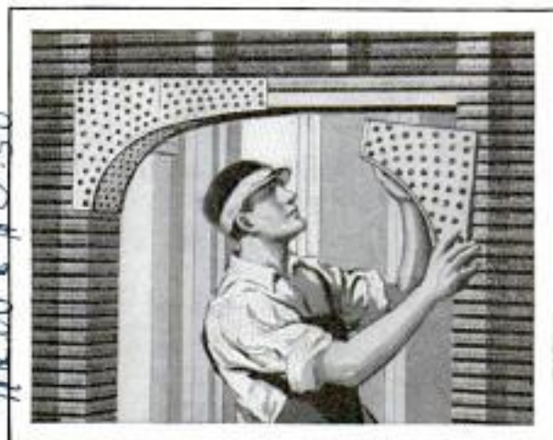
Ready-Formed Metal Arches Which Provide a Symmetrical Plaster Base for Such Types of Doors
