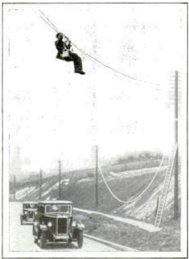
Lineman Riding Telephone Wires over a Busy Highway on a Seat Suspended from a Cable
