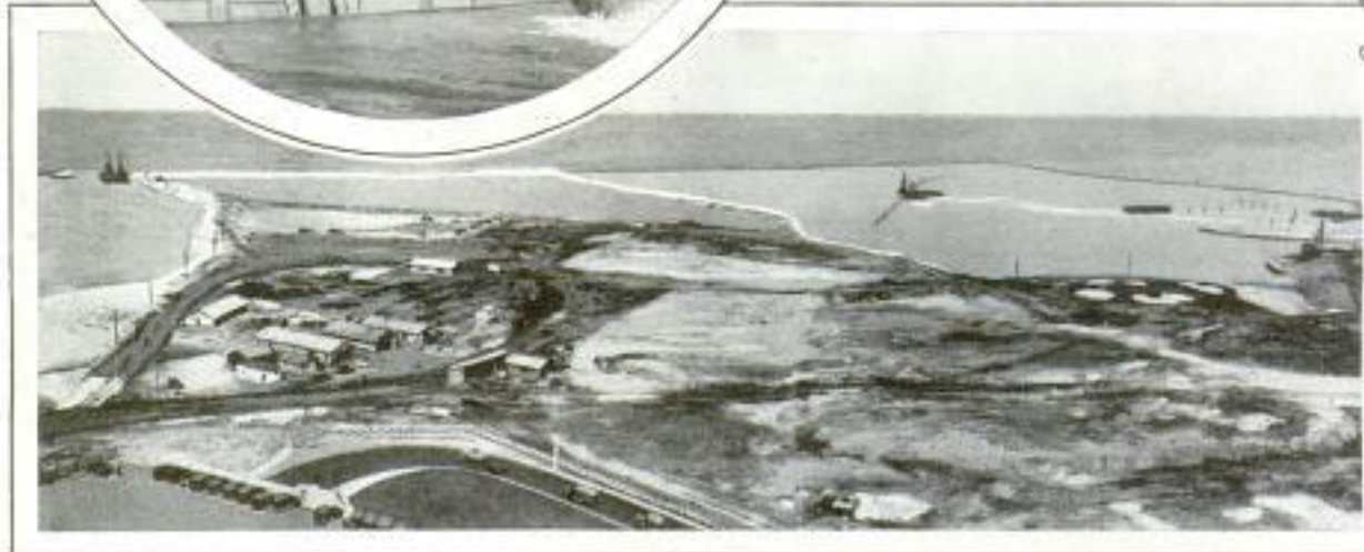
General View of a Section of Chicago's Lake Front Composed of "Made" Land, Formed by Filling in Sand along the Shore Line; Above, One of the Big Sand Boats Dumping Its Load
