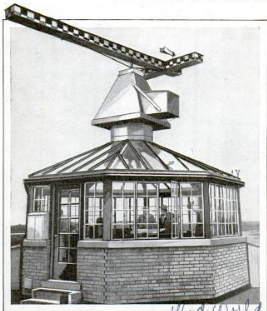
Airport Traffic Tower from Which Pilots Receive Orders by Radio; the Tower Operator Also Controls the Lights for the Field
