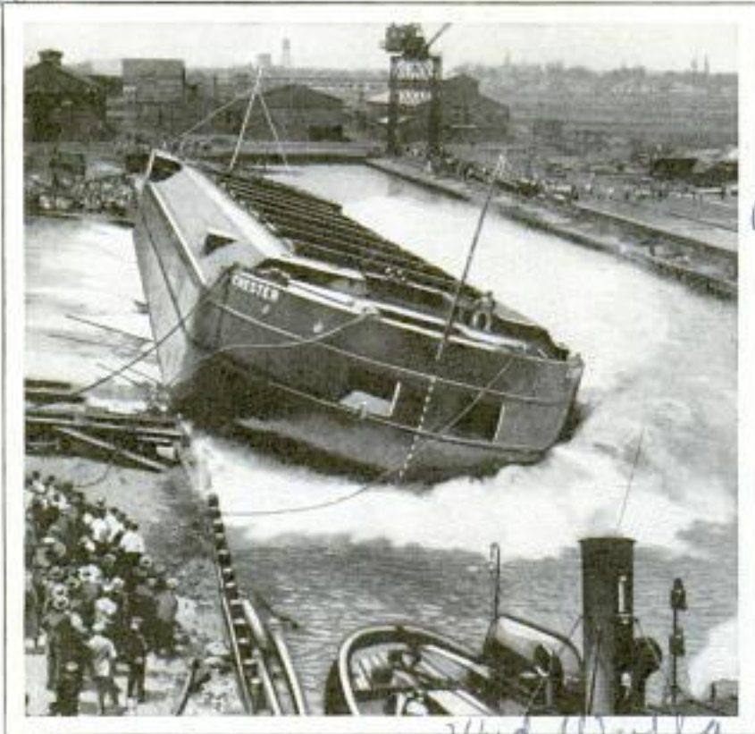
Launching a Turbine Ship Which Will Carry Automobiles from Detroit to Atlantic Seaboard; the Vessel Is 300 Feet Long
