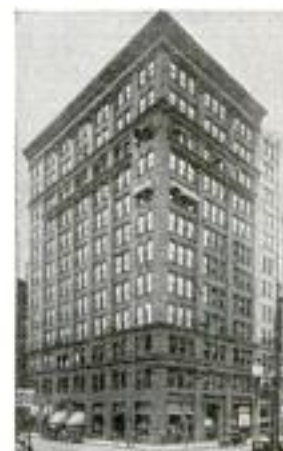
Our Pittsburgh Office Suite 514 Empire Building
