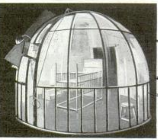
One-Way Screen Which Permits Observers to Watch Infants in Nursery without Being Seen
