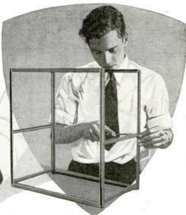
Lightweight Angle Iron Used for Assembling Small Transmitter Frames May Also Be Employed for Constructing Shielded Metal Cabinets to House Homemade Radio Receivers
