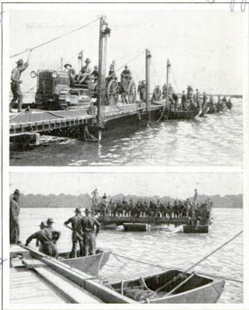
Whole Section of Horse-Drawn Artillery Is Ferried across River on Motor-Driven Pontoons; Top, Two Sections of Motorized Ordnance Land
