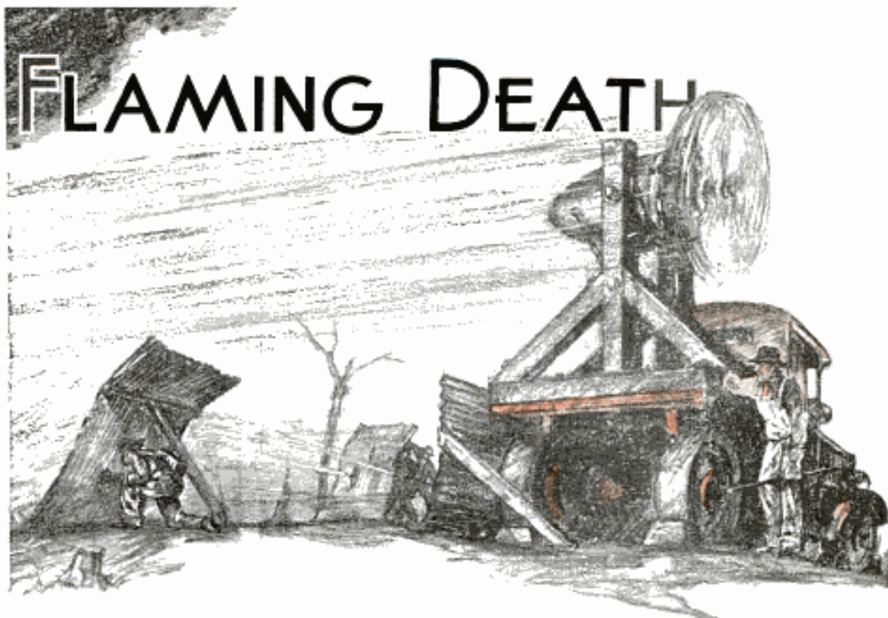
An Airplane Engine Mounted on a Truck Blew a Blast of Air against the Inferno, While Chains Were Carried Forward to Snake Away the Hot Machinery
