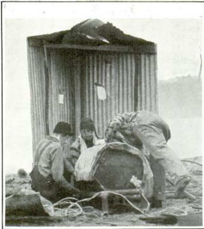
Courtesy Dallas News Preparing a Seventy-Quart Charge of Nitroglycerine to Blow Away a Joint That Was Diffusing the Flaming Spray
