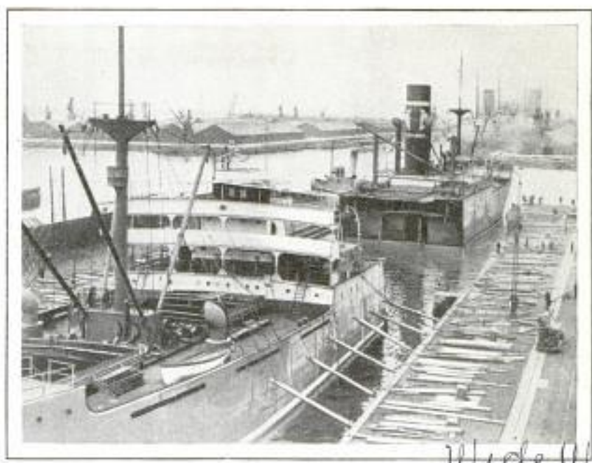
Preparing to Join Together the Halves of a Large Steamer After Vessel Had Broken in Two When It Went Aground in a Fog
