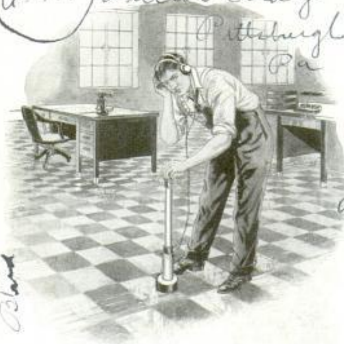
Using a Modern Divining Rod to Which Headphones Are Attached in Locating Electrical Wiring Hidden under Floors
