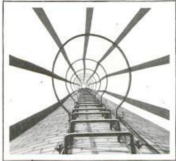
Looking up the Side of a Tall Chimney; Metal "Spiderweb" Protects Workmen on Ladder
