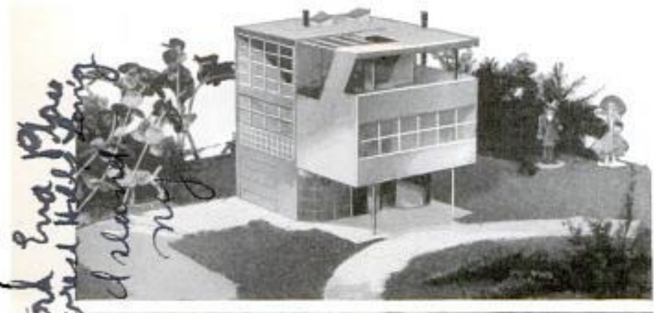
Model of a Home of Aluminum and Glass; Structural Work Is Entirely of Metal and the Walls Are Composed of Aluminum Sheets
