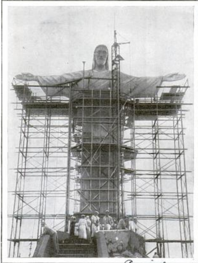
Partly Completed Statue of Christ on a Mountain in Brazil; It Is 150 Feet Tall and the Spread of the Arms Is 125 Feet
