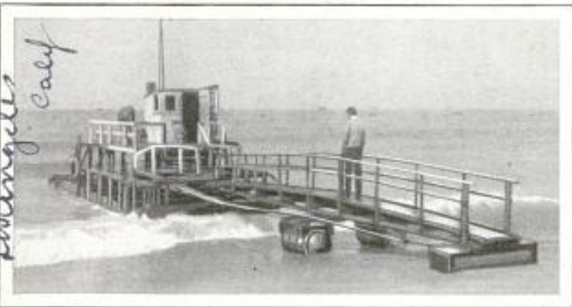
Wharf That Serves as a Ferryboat and Moves into Water to Meet Other Vessels; Note the Pier with Rollers That Travel in Sand
