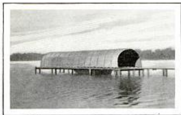
Huge Canvas Tarpaulin, Stretched over Curved Framework on the Dock, Forms an Excellent Boat Shelter
