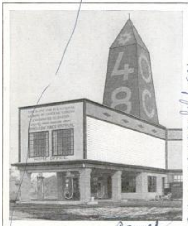
Aerial Guidepost Which Carries Latitude and Longitude Markings for the Airplane Pilot to Read
