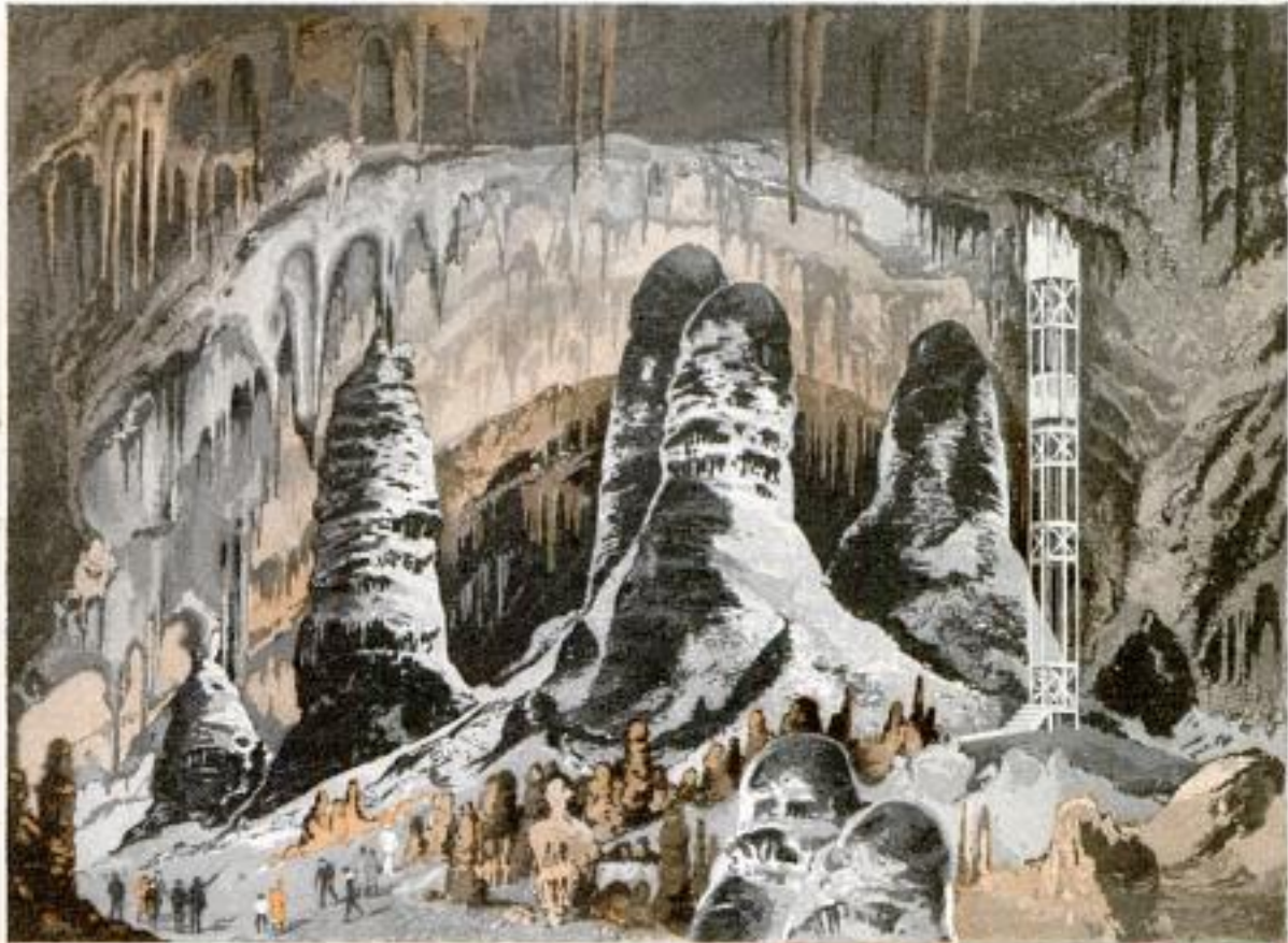
Drawing of Elevator Being Constructed to Descend into Carlsbad Cavern; the Shaft Will Rise 750 Feet, Making It the Longest Single Lift in the World
