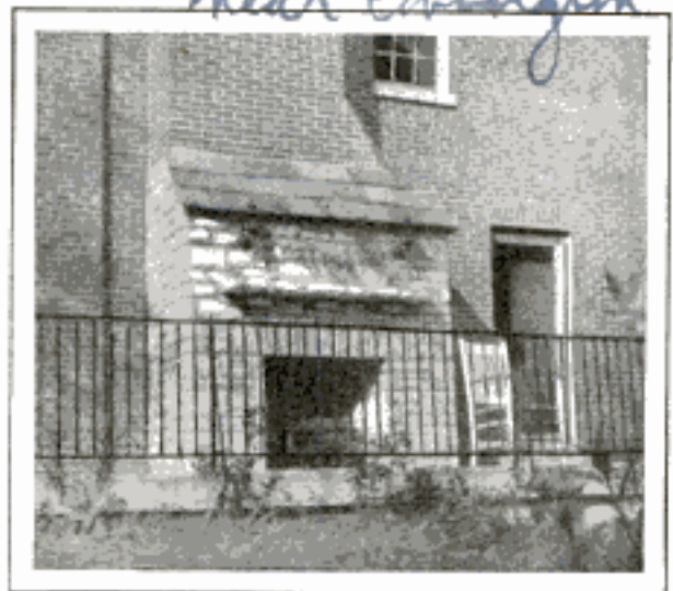
Residence with Open Fireplace in an Outer Wall; It Warms a Veranda on Cool Evenings
