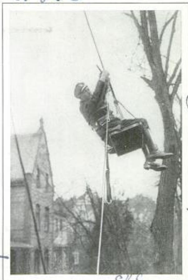
Aerial Tramway and Seat for Lineman; He Is Pulled along Auxiliary Wire by Workman on Ground
