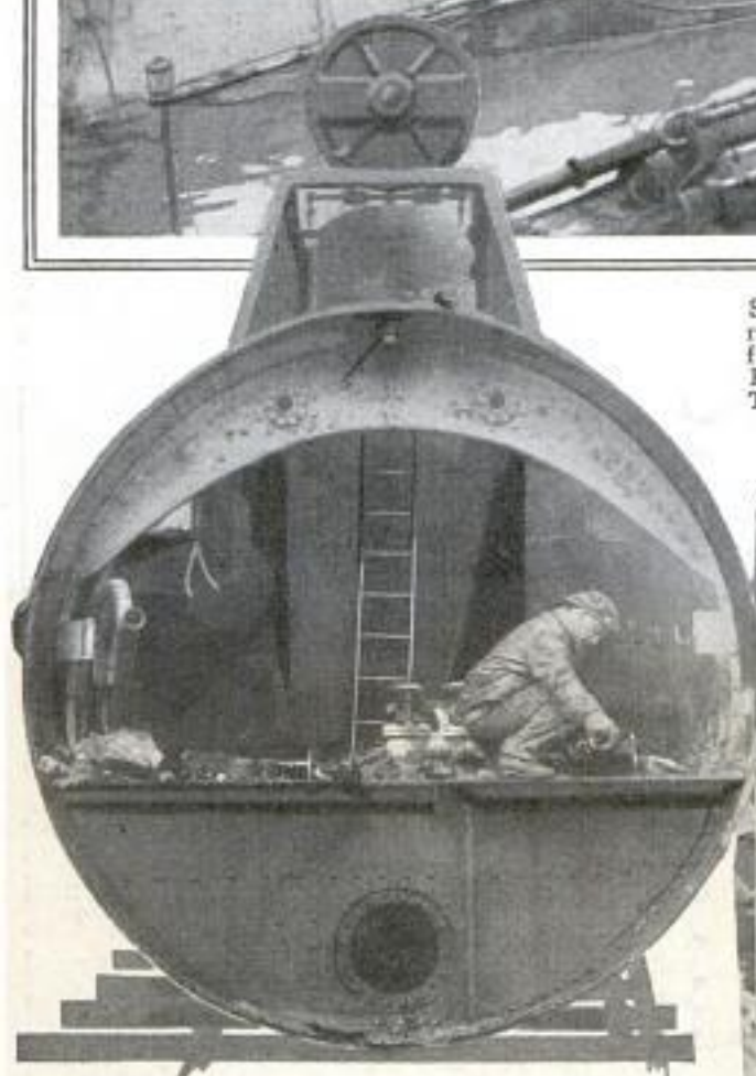
Using Acetylene Torch to Cut the Steel Plates of One of the Decommissioned Subs; the Metal Will Be Sold as Scrap Iron; at Right, Cutting Away the Control Room of an Undersea Craft Which Has Outlived Its Usefulness and Is Now Being Dismantled and Consigned to the Junk Heap
