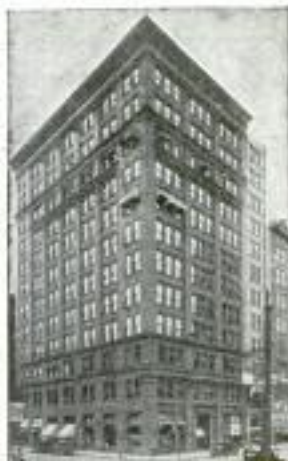
Our Pittsburgh Office Suite 514 Empire Building
