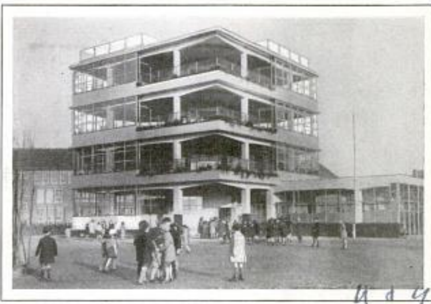
Grammar School in Holland with Glass Walls; the Walls Are Easily Opened, Thus Placing Pupils Virtually Outdoors in Good Weather
