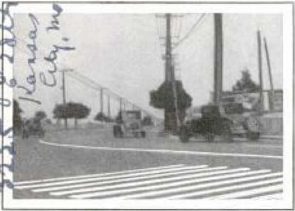
Stripes across Road Are Samples of Paint under Test to Find the Best for Road Marking
