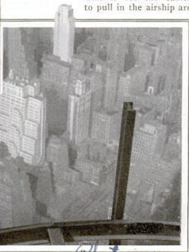
Above, Cross Section of the Mooring Mast on Empire State Building and Manner of Operation; Below, a View of New York Taken from the Top of the Mooring Mast
