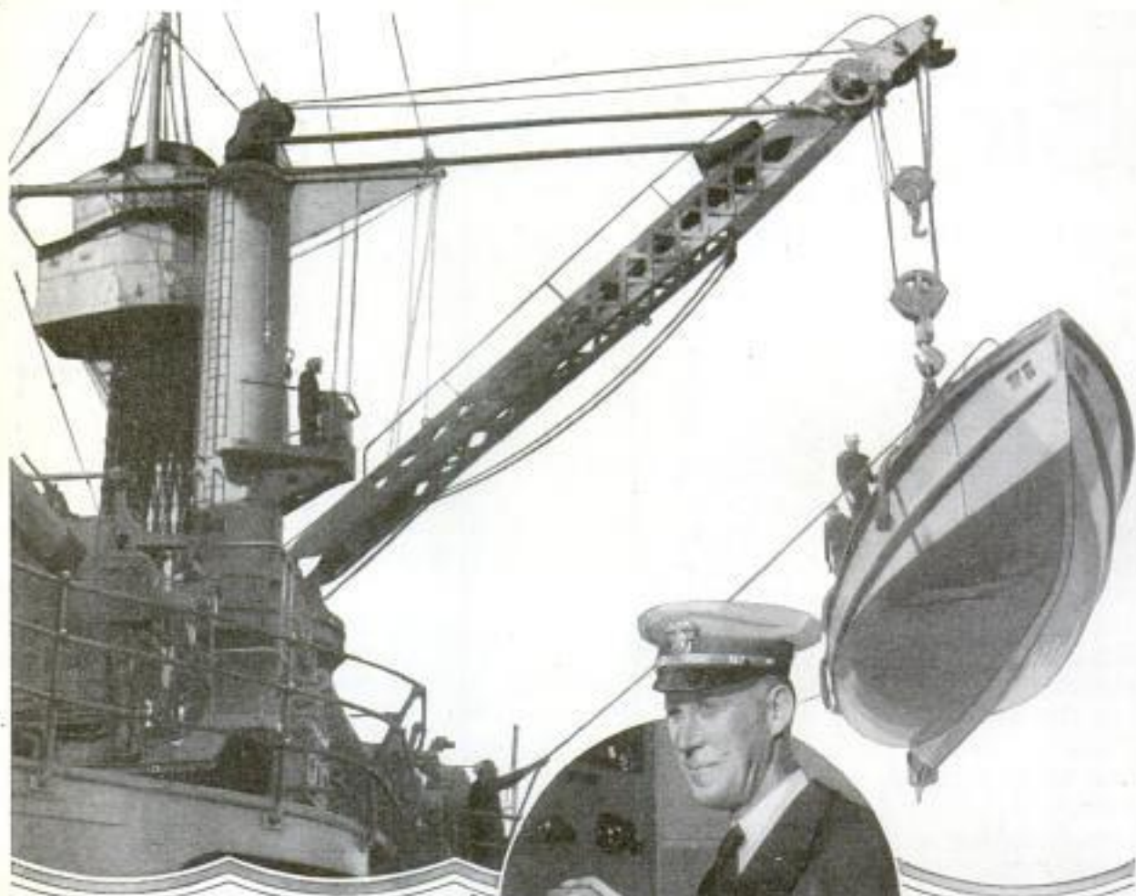
Above, Hoisting a Large Launch aboard a Battleship; in Circle, Three-Pronged Fork Used to Measure the Heat of the Bearings on Any Motor; Right, Seaplane Ready to Be Hoisted aboard Ship after Flight from a Catapult; the Pilot Attaches the Hook to Four Cables Leading to Points on the Plane
