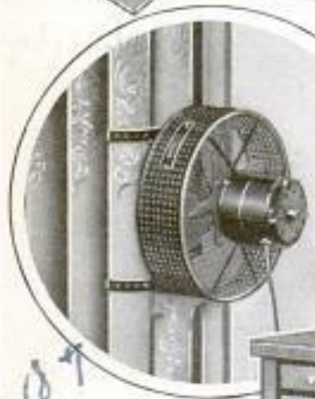
Electric Radiator Fan Which Increases Radiation by Forcing a Larger Amount of Air over Radiator, Resulting in Quicker Heating
