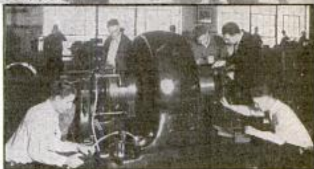
Students working on a large synchronous Converter
