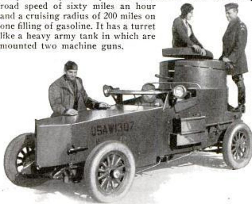
Light Armored Car Tested for the Army; It Can Travel Sixty Miles an Hour and Has a Cruising Radius of Some 200 Miles
