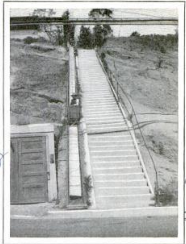
Electrically Operated Car on a Track Which Saves Climbing Steps to This California Home
