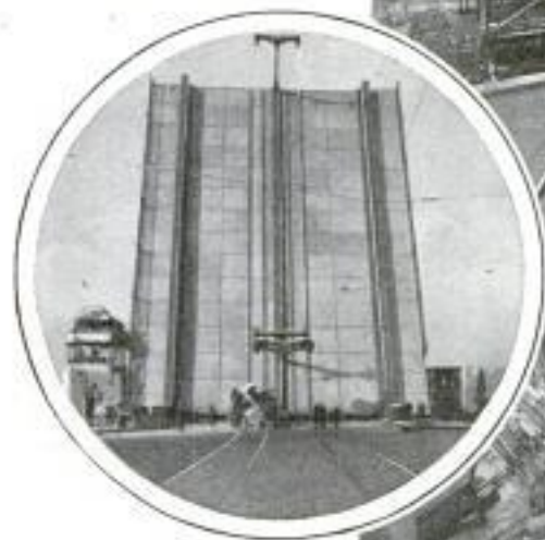
Lift-Bridge Floor of Non-Skid Concrete Slabs; Before Floor Was Laid, and Placing a Slab
