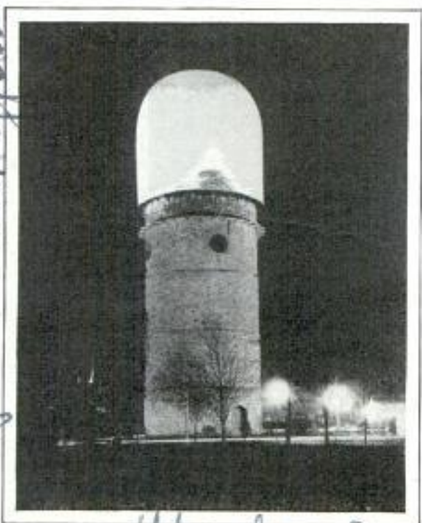
© C. E. Lamb. Ypsilanti Mich Floodlighted Water Tower Which Serves Also as a Landmark for Aviators Flying at Night
