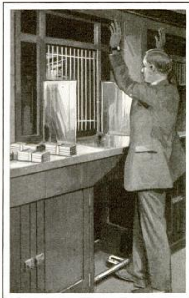
Foot-Operated Bank Alarm Which Rings Continuously When the Pedal Bar Is Moved Upward
