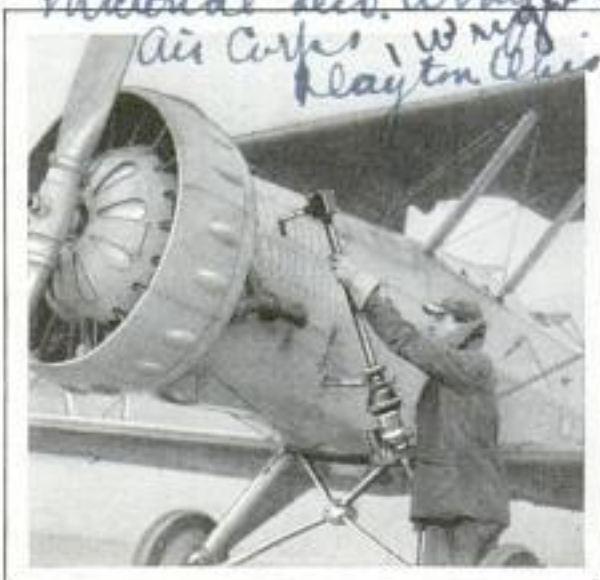
Electrically Operated External Airplane Starter Which Fits over Crank of Hand Starter
