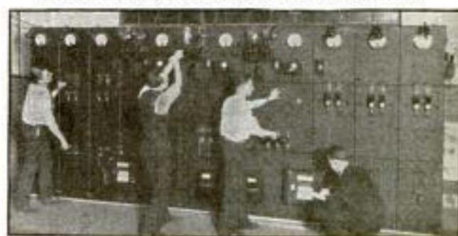
Students learning switchboard work by actual practice
