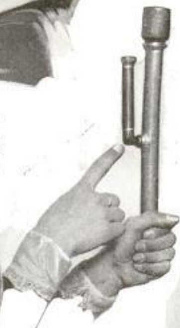
At Right, a Simple Device to Keep Water Pipes from Bursting if They Freeze; the Small Valve Attachment Allows for Expansion and Helps Prevent Freezing; It Is Easily Installed and Requires No Attention
