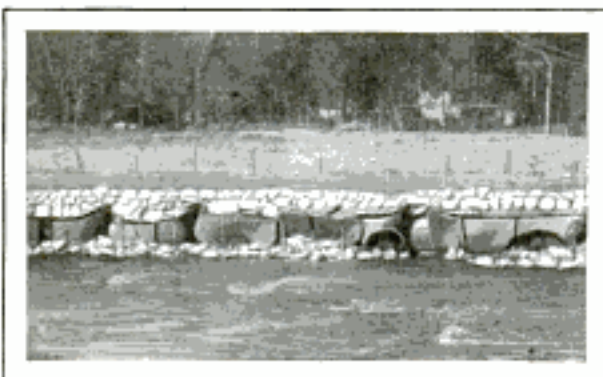
Old Auto Bodies Lined on River Bank and Filled with Rocks Make a Strong Water Wall
