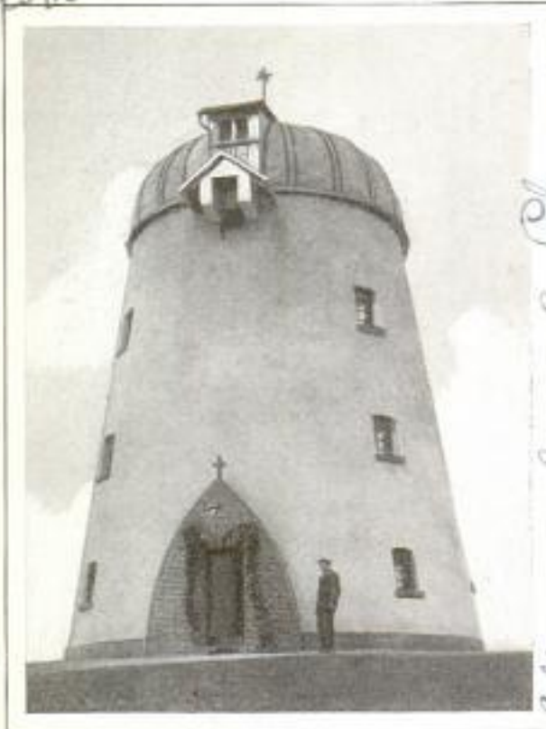
Windmill Tower Converted into Church: the Bell Is Suspended in Niche of Old Hub Opening
