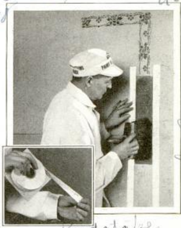
Holding Stencil with Special Tape While Painting, and Close View of a Roll of the Tape
