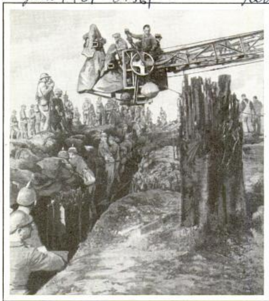
Courtesy Je Sais Tout Camera on a Swinging Crane for Taking Crowd Movies: the Crane Is Mounted on a Truck, Thus Affording Great Maneuverability
