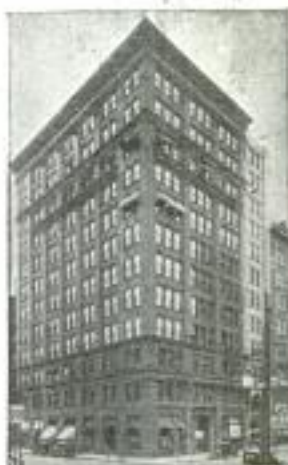
Our Pittsburgh Office Suite 514 Empire Building
