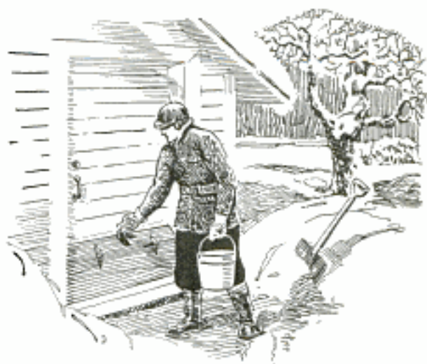
This Wooden Guard with Hinged Flap, Keeps Snow Away from Outside Doors
