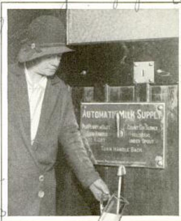
Automatic Dairy Which Delivers a Mug of Milk When a Coin Is Deposited and a Handle Turned
