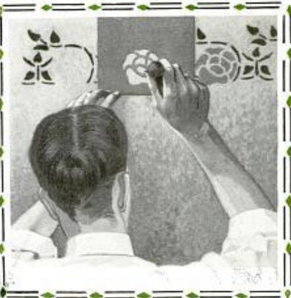
Applying the Second Color: Below. Notice How the Brush Is Held and Pounced against the Stencil
