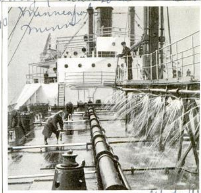
Sprinkler System Supplies Artificial Rain to Cool Deck and Cabins of British Oil Tanker in Tropical Waters
