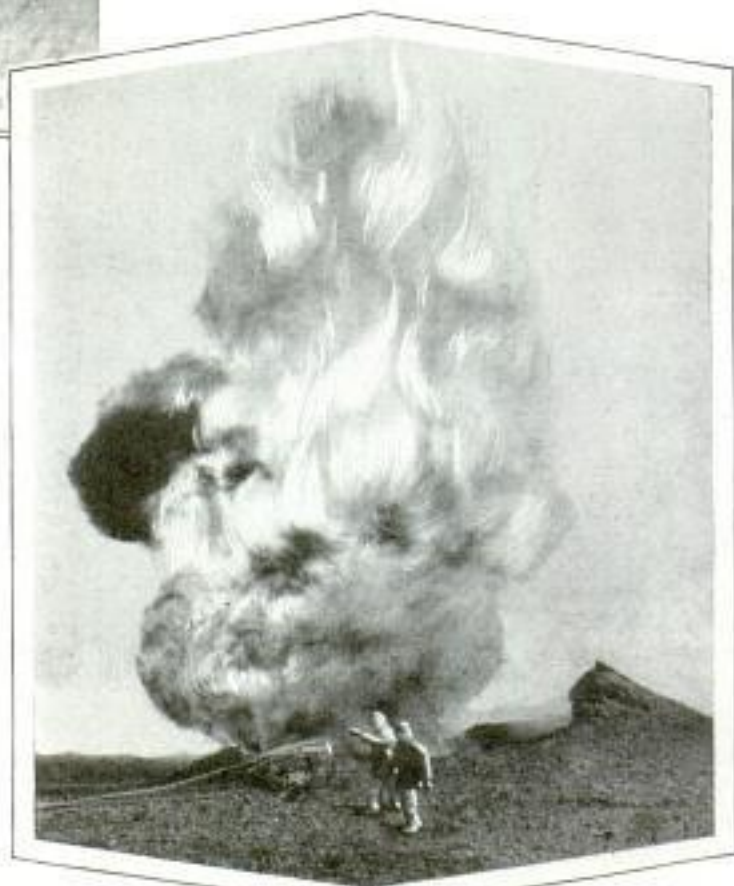
Tex Thornton and His Gun of Nitro near Oil-Well Fire, and, Below, Clad in Asbestos Suits, Preparing to "Shoot" a Crater Fire
