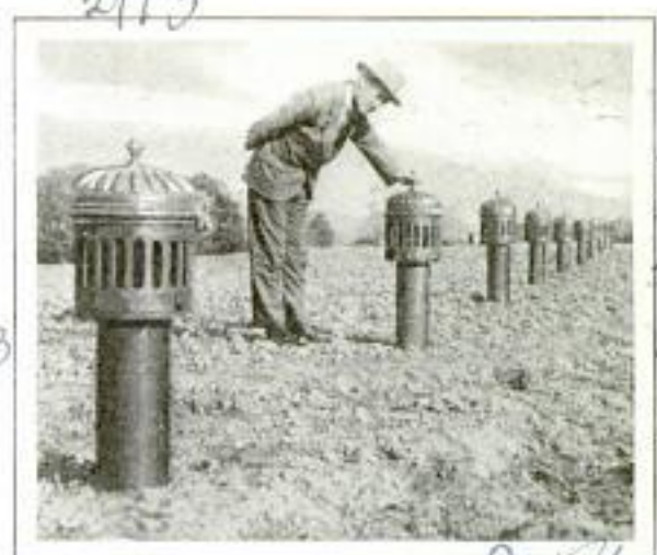
The Row of Pipes Leads to an Underground Lake Supplying an English Town with Water
