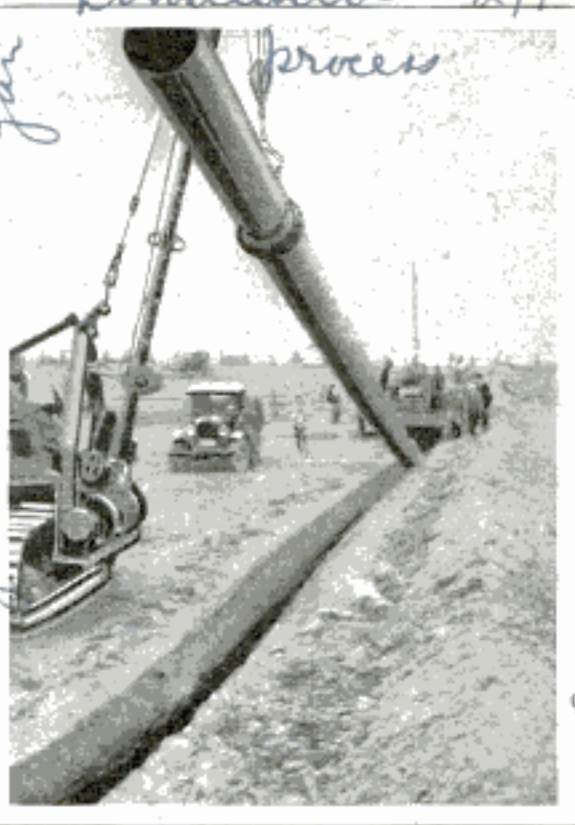
Laying a Section of Pipe That Has Been Welded under Improved Process That Saves Time
