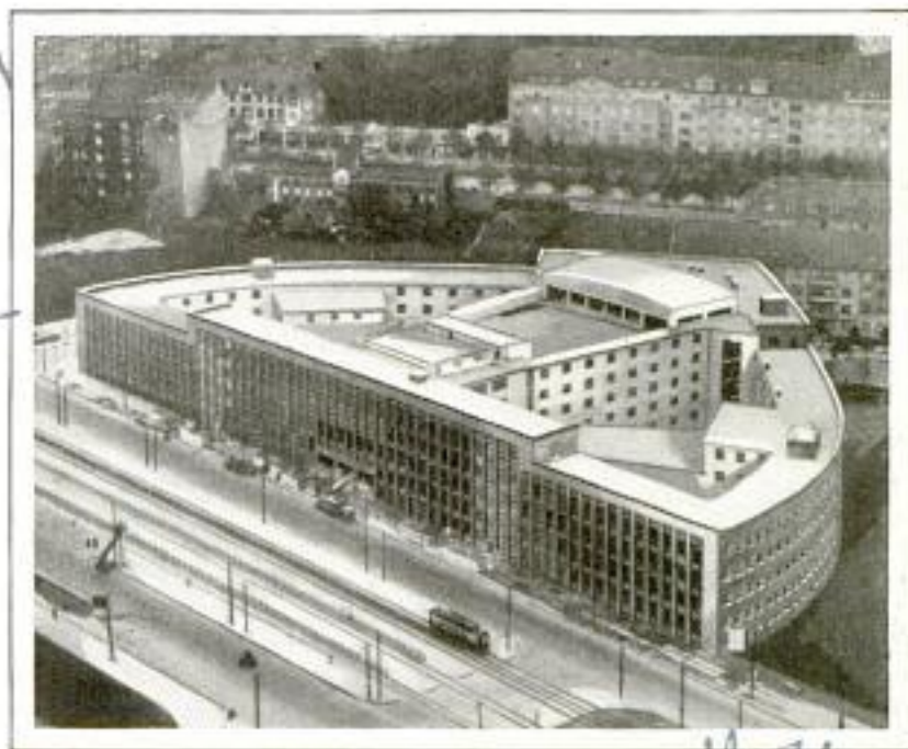
Berlin's "Radio City": Huge Building Which Contains Broadcasting Studios and a Large Radio Museum, Displaying Pioneer Equipment
