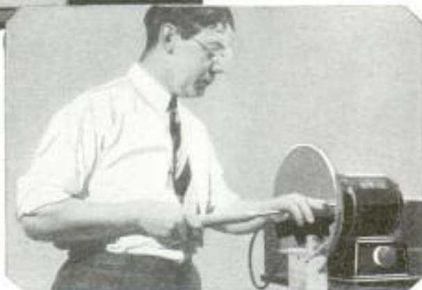
Turning the Tray on the End of the Headstock
