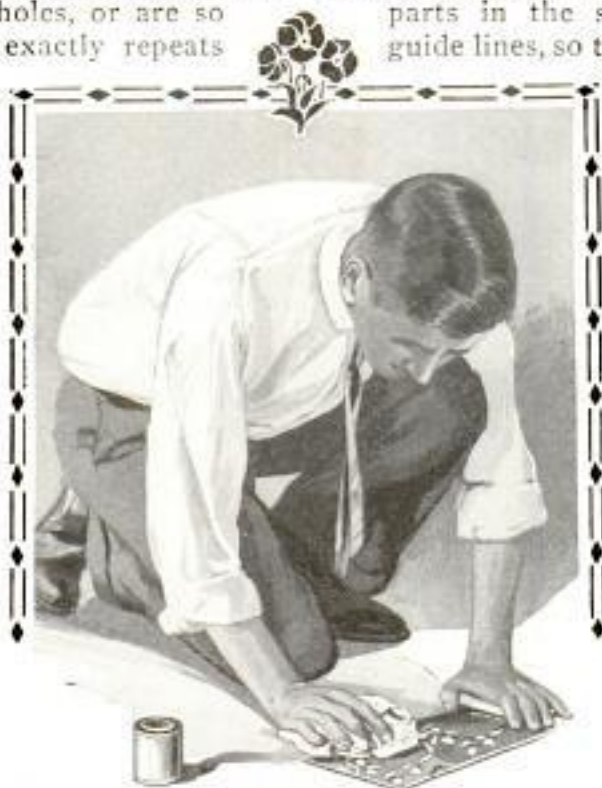
Wiping Off the Back of the Stencil between Settings, to Prevent Smearing the Wall
