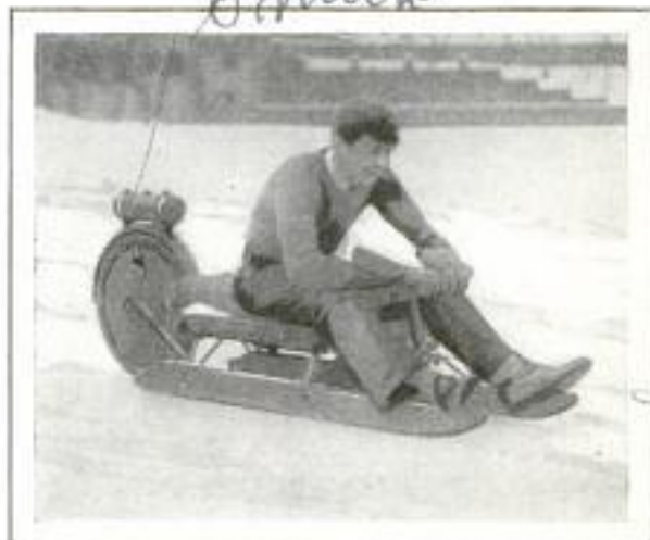
Ice Sled Propelled by a Gasoline-Driven Motor Wheel Adds Speed to This Winter Sport
