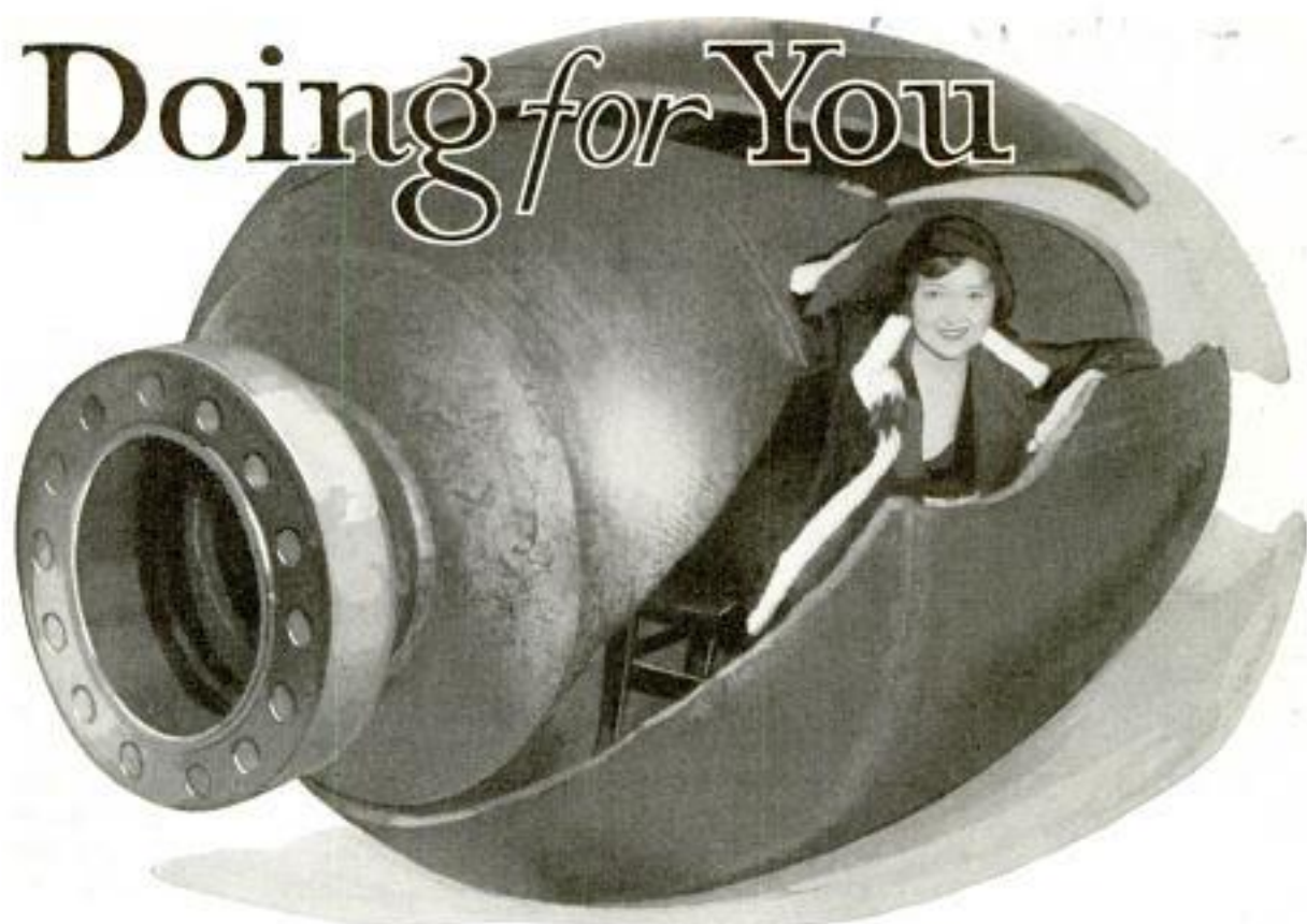
This Steel Ball Burst under Heavy Pressure, but the Break Did Not Occur at the Welded Spots, Indicating the Efficiency of Modern Welding Methods
