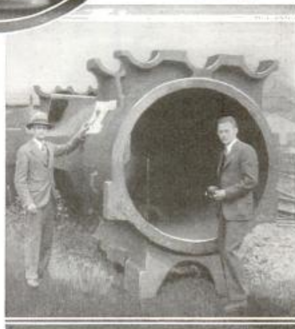
Close View of Radium Torch, "Shadowgraph" of Valve and Preparing to "Gamma-Ray" Large Casting
