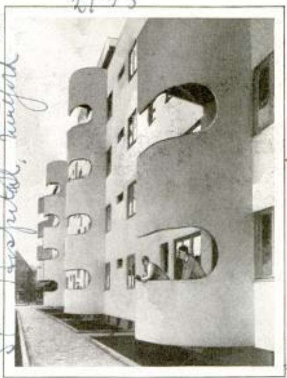
Curved Balconies of German Building, Which Resemble Niches Cut in Semicircular Columns
