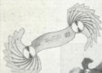
Screw Pitch Gauge No. 610
