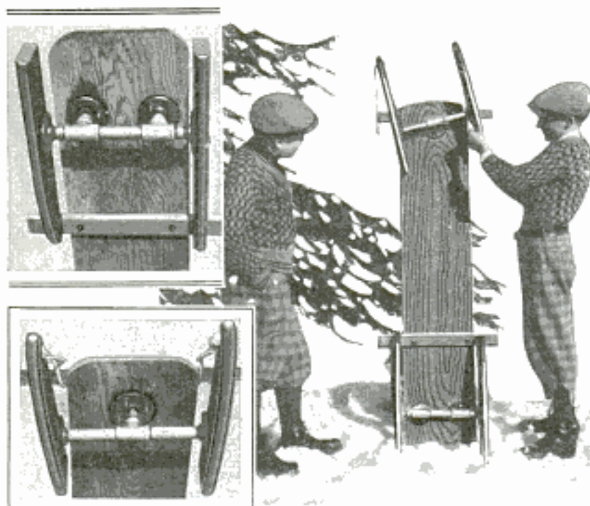
In the Construction of This Bobsled, Pipe and Pipe Fittings Were Found Highly Suitable
