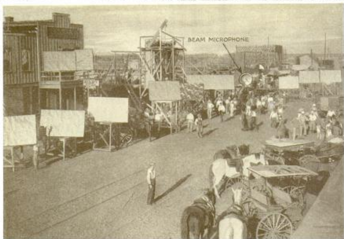
Getting Ready to Take a Scene for "Cimarron"; Note Arrow Pointing to Beam Microphone and the Light Reflectors Adjusted on Set Opposite One to Be Filmed
