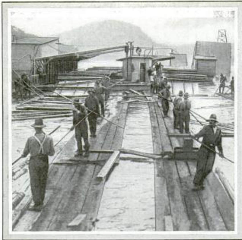
One of the Sorting Gaps in a Quebec Lumber Camp, Where Over 250,000 Logs Are Handled Daily by Experienced Workmen
