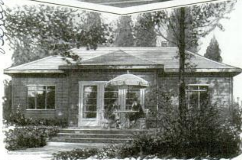
Above, Erecting a Copper Cottage, a Task Requiring Only Twenty-Four Hours; Below, the Completed Home a Day Later
