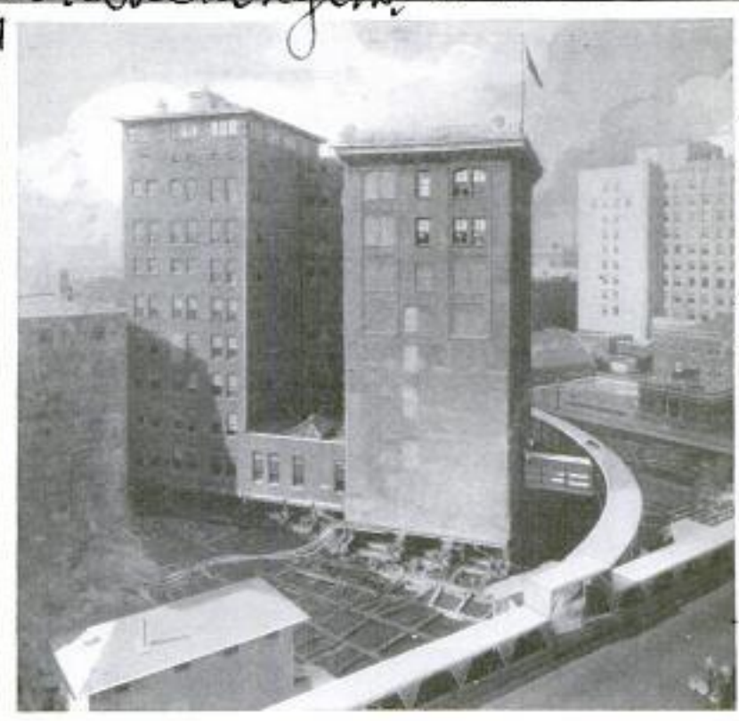
Moving an Eight-Story Office Building Weighing 11,000 Tons; the View Shows the Structure After It Had Been Turned Around
