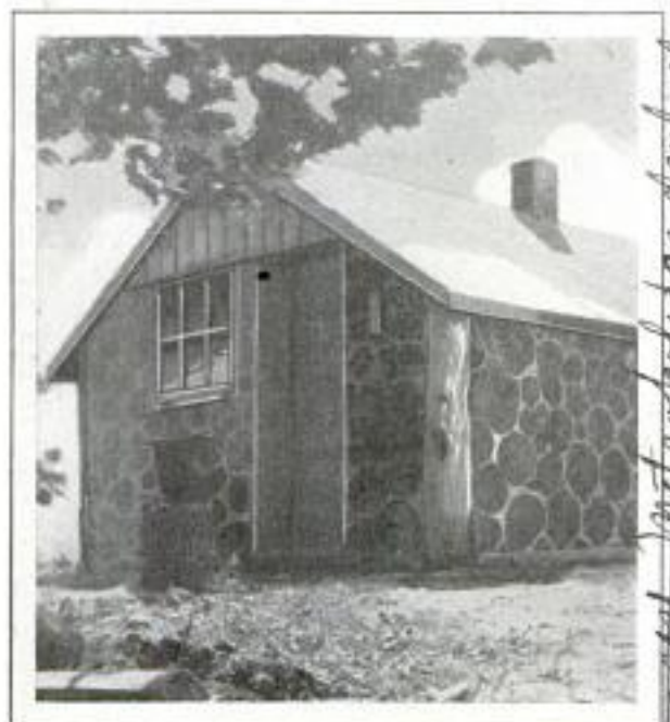
Blocks Sawed from Logs and Set into Mortar Form the Walls of This Attractive Cabin
