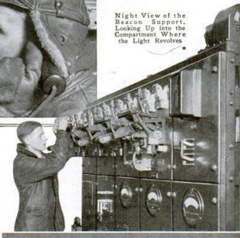
Laibly at Phone Which Communicates with Watchman and Attendants of the Palmolive Building; at Right, About to Throw the Switch Which Turns on the Light; the Beacon Is Polished Daily, and, during the Time It Is Burning, the High-Intensity Carbons Are Changed Once an Hour; the Elevator Takes the Keeper About Twenty-Five Feet below the Light; the Remainder of the Journey He Climbs by Ladder; Warm Clothing Is Necessary during the Winter Watches
