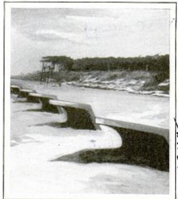
Portable Breakwater Units Shaped Like a Ship's Bow, Which Protect Bathing Beaches from Waves
