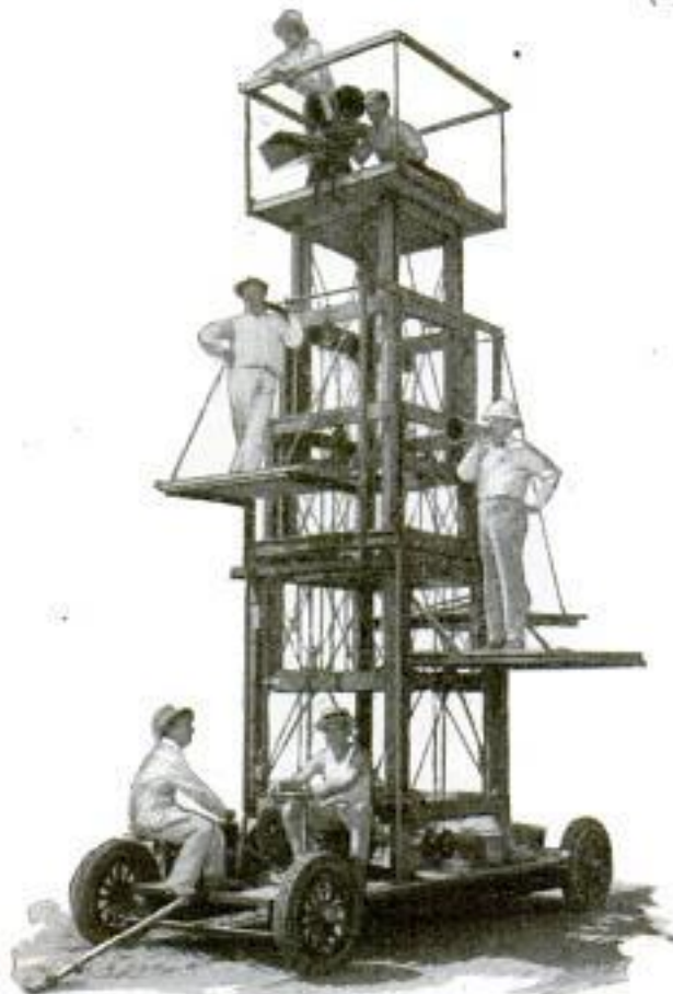
A Tower on a Truck Used in the Movies for Quick Transportation and Elevation of Cameras
