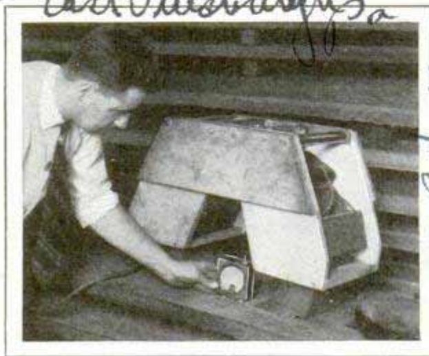
Magnetic Apparatus and Gauge Being Used to Test Efficiency of an Electric Welding Job
