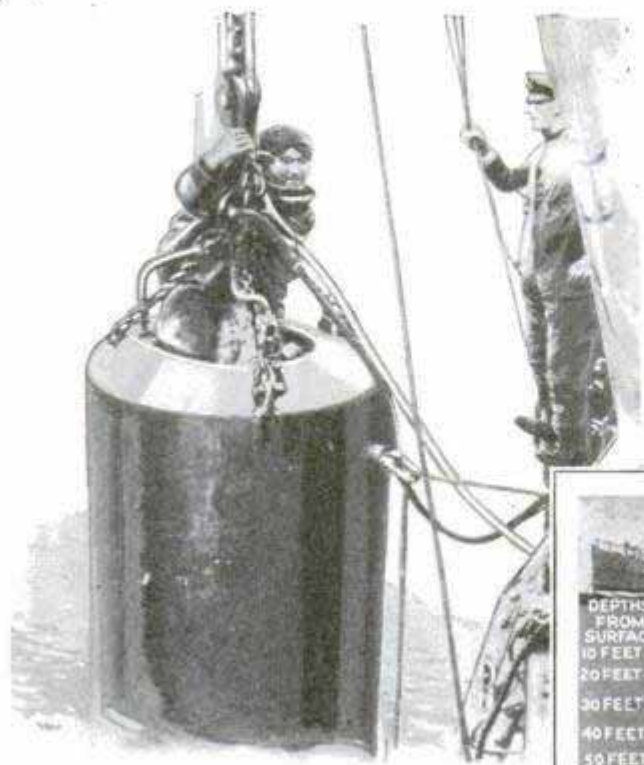
Views of the Compression Chamber Used by British Divers; Dives to Fifty-Eight Fathoms Have Been Made with It
