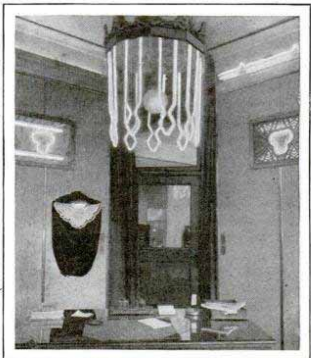
Chandelier Composed of Neon Tubes in Different Colors, Which Combine to Give a White Light
