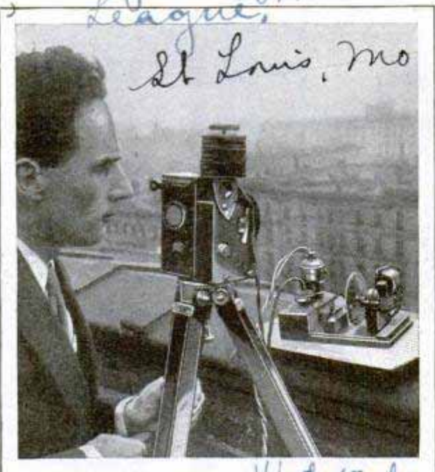
Camera Actuated by Time Clock, Which Takes Pictures of Smoking Chimney at Minute Intervals
