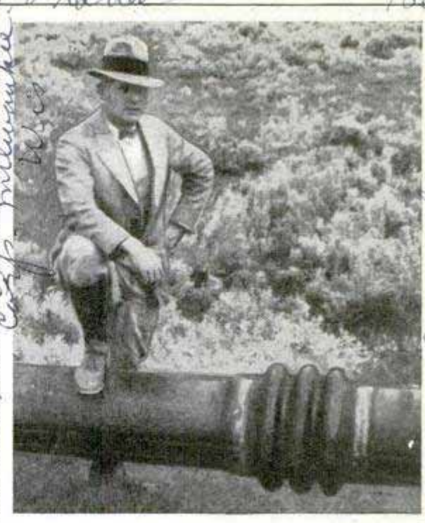
Corrugated-Steel Expansion Joint for Pipe Line, Which Allows It to Contract or Expand
