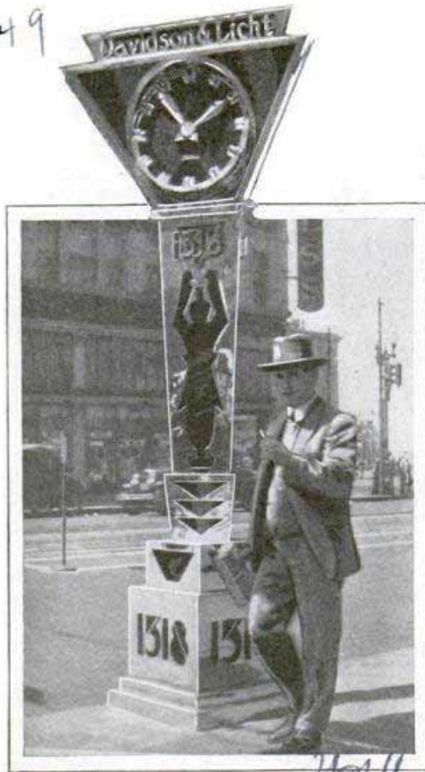
Modernistic Street Clock Operated by Electricity; the Base Is of Chromium and Vitrolite
