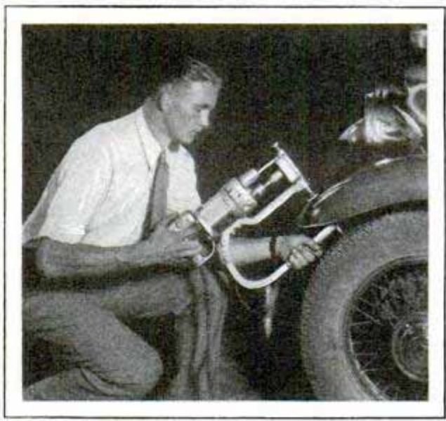
Electric Hammer and Anvil Employed in Ironing Out the Dents in Auto Fenders and Bodies
