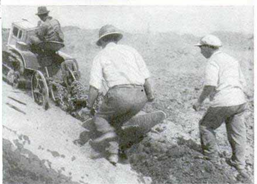
Top, Steel Framework of Water Tanks Rising Where the Children of Israel Wandered; Below, Workmen Excavating a Feeder Canal
