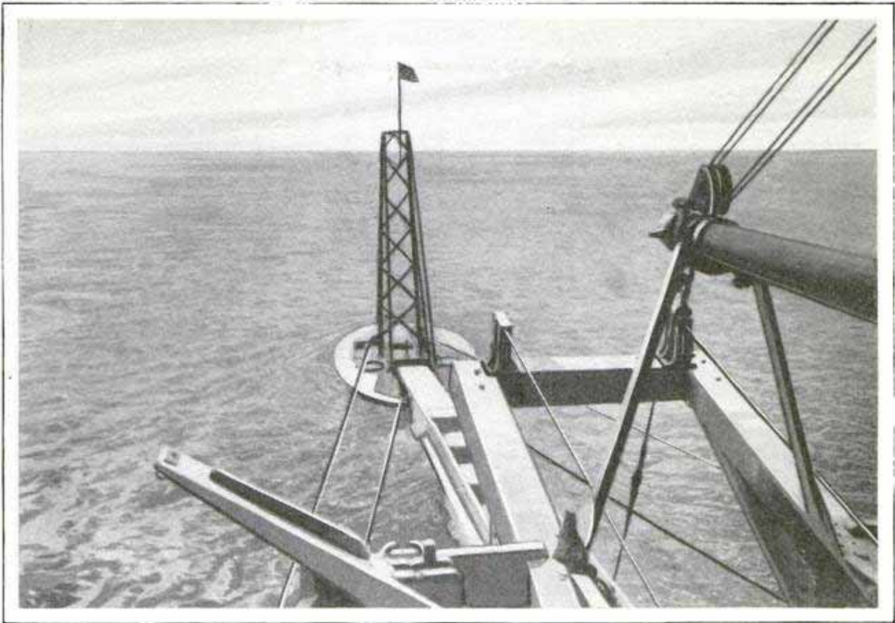
Submarine Tube and Chamber for Use in Depths of Fifty Feet and Less; the Tower with Flagstaff Warns Surface Craft and Protects Submerged Tube
