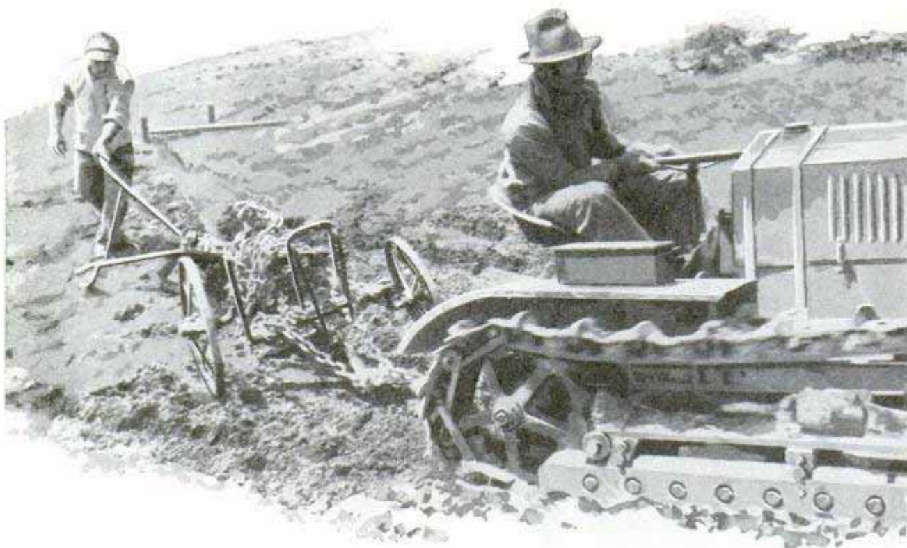
Excavating One of the Canals in the Development of This Biblical Territory; the Project Is Expected to Make Available Minerals and Chemicals Worth Millions of Dollars
