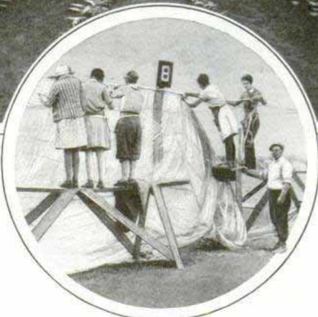
Tent, over a Connecticut Tobacco Field to Increase Humidity; Below, Placing One of the Tents in Position
