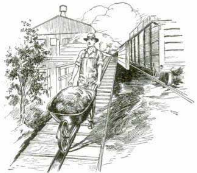
Length of Channel Iron Laid on Cleated Runway Guides Wheelbarrow
