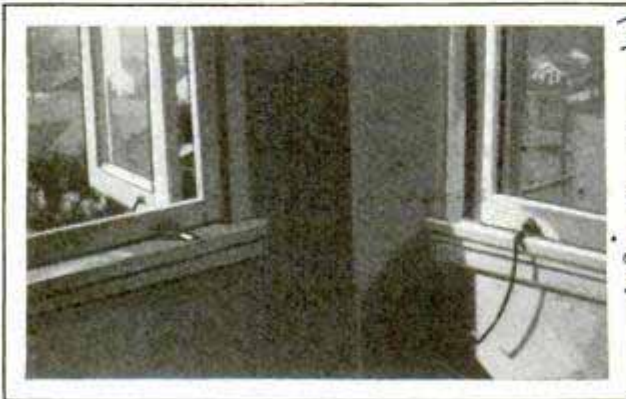
Casement-Window Adjuster Which Operates through the Screen
