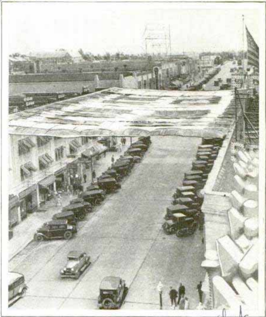
Awning Containing 6,000 Square Yards of Canvas Stretched over a Business Street to Protect Shoppers from Sun and Rain
