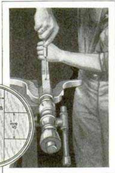
Top, the Completed Table, with Fluted Column and Reeded Legs; Bottom, Screwing a Leg to the Column
