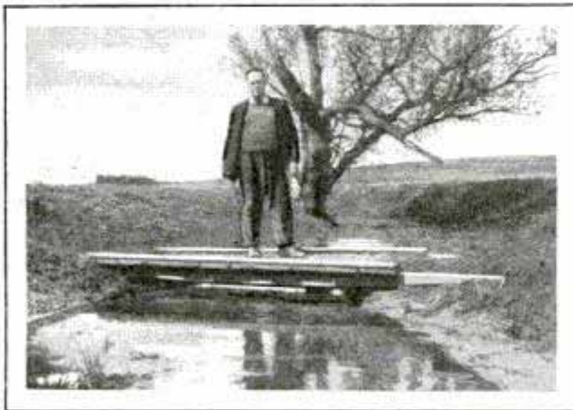
Improved Pasture Bridges Made from Old Auto Frames Are Cheap and Sturdy
