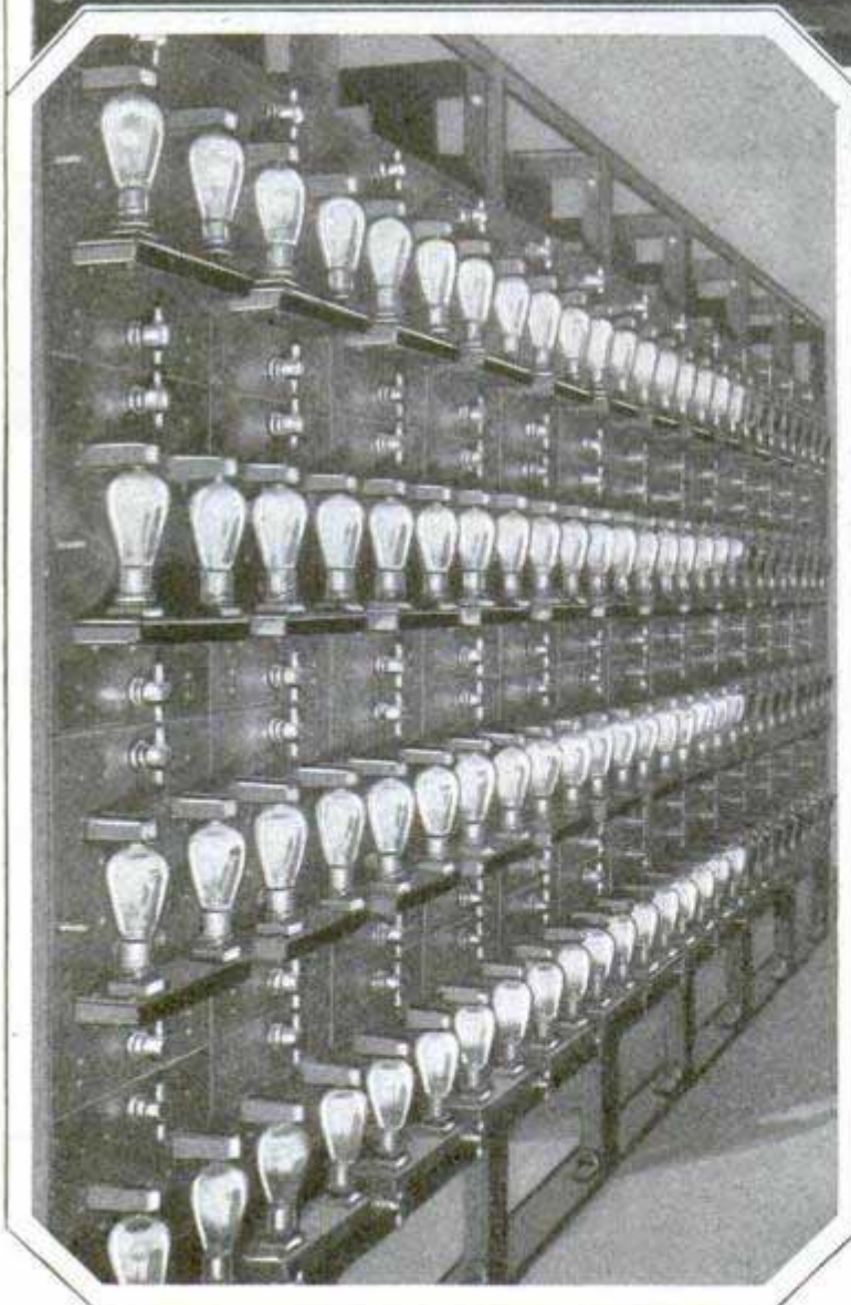
Scene from "Love of Three Kings," and Thyatron Rack for Chicago Civic Opera Installed Eleven Floors above Stage
