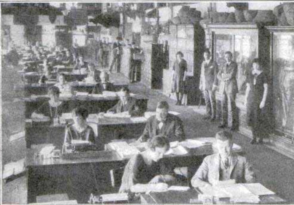
MAIN OFFICE, VICTOR J. EVANS & CO.—VICTOR BUILDING, WASHINGTON, D. C.
