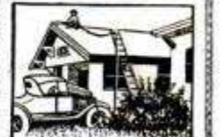
Painting Shingle Roof
