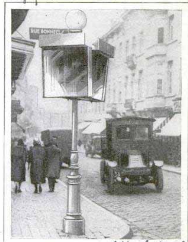
Mirrors at Intersections of Narrow Streets in Brussels Give Auto Drivers a View of Traffic
