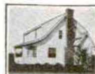
In this Mentor, Ohio, home, designed and built by R. M. Case Co., Masonite added little to the cost.
