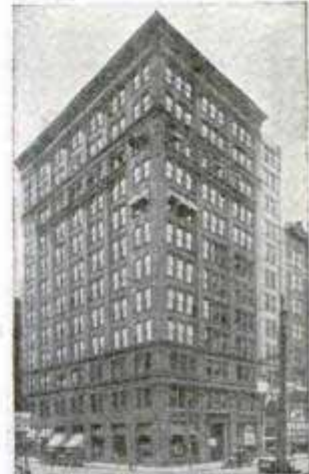
Our Pittsburgh Office Suite 514 Empire Building
