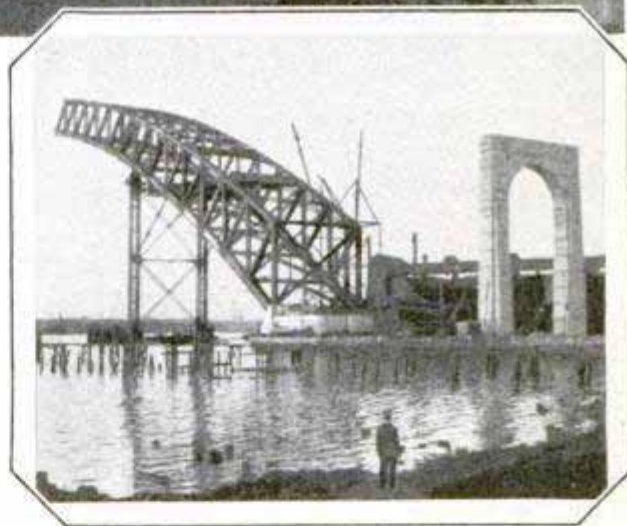
Concrete Arches and View of Partly Completed Span of the Kill Van Kull Bridge
