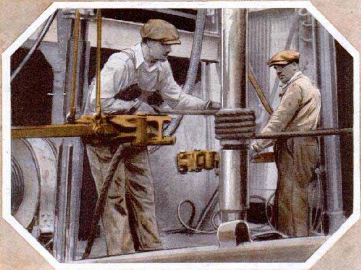
Members of a Well Gang Spinning In a Length of Drill Pipe over a New Deep-Zone Well at Santa Fe Springs, California; the Huge Tongs, Used in Tightening the Connection, Are Just Being Swung into Place; This Is One Reason Why a Deep Well Cannot Be Drilled in a Day
