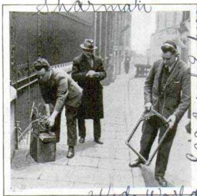
Using Radio Apparatus to Locate Buried Pipe Line
