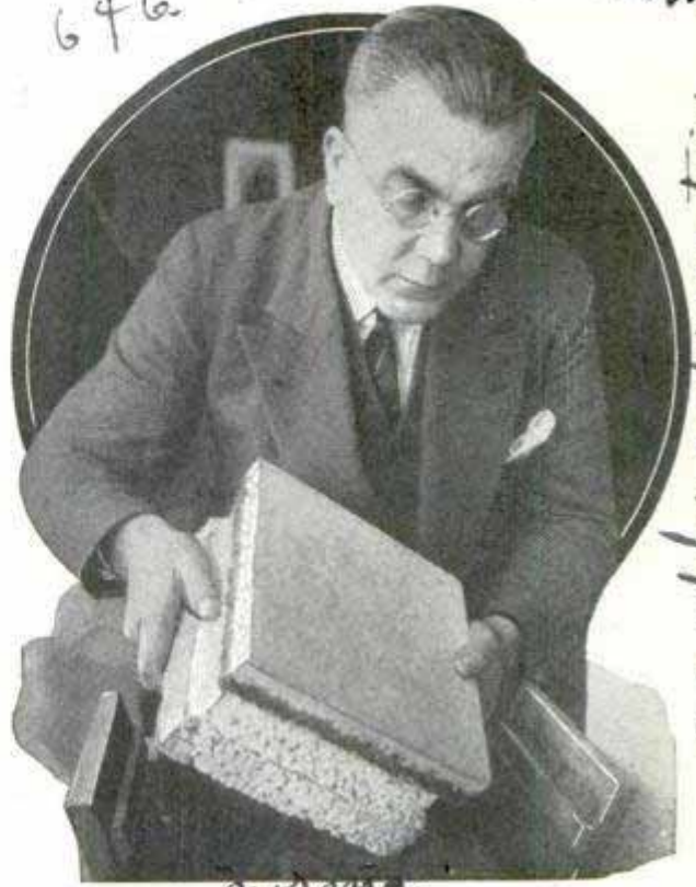
Special Concrete Building Block, Showing the Smooth, Waterproof Surface, and Center Structure
