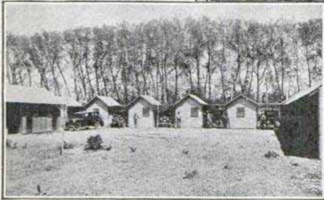
Roadside cabins can be built economically of Presdwood and they stand the weather well.
