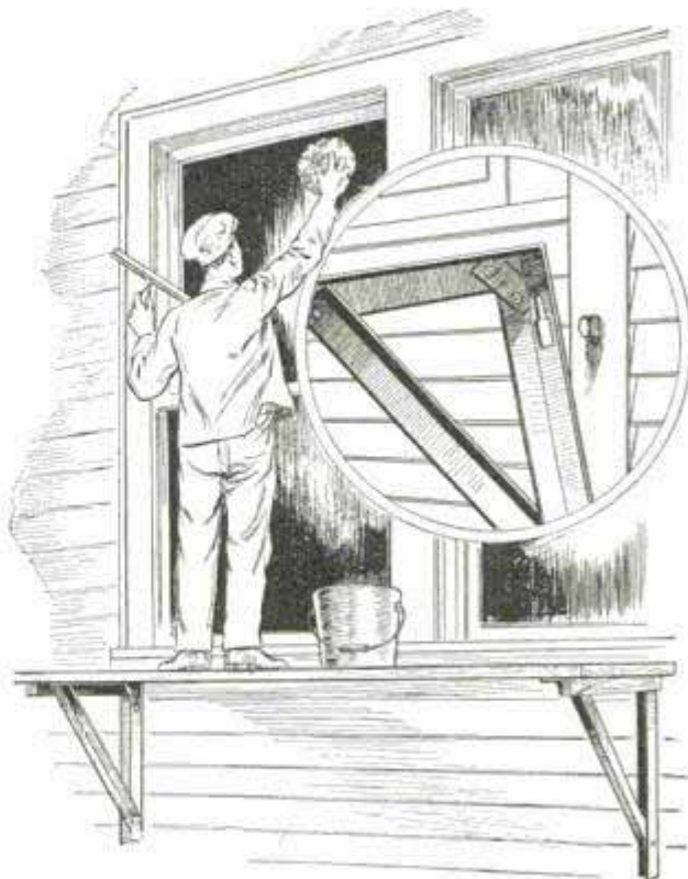
Slotted Supports for Scaffold Are Slipped on Permanent Lagscrews in the Wall
