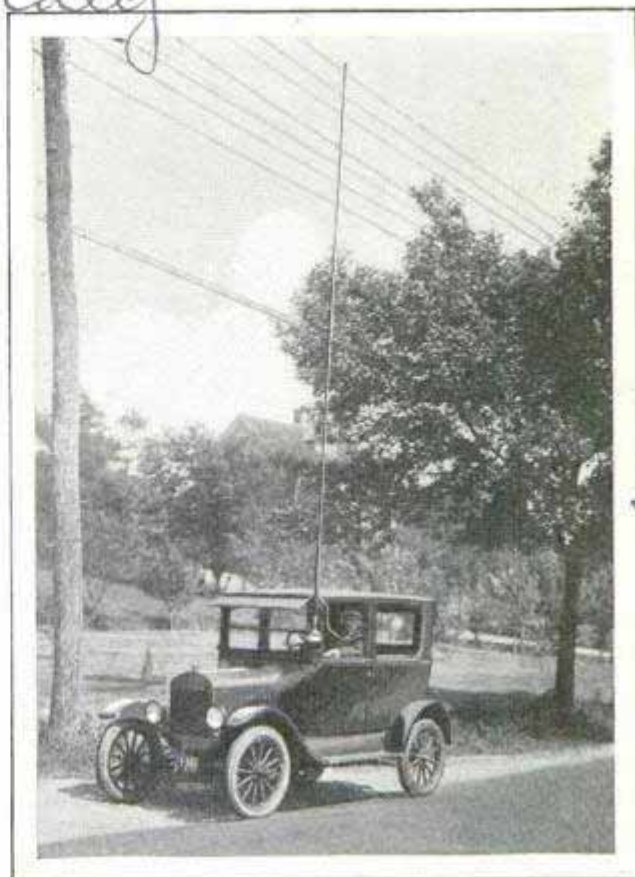
Auto Containing Equipment for Locating Source of Radio Interference; Note the Rod Antenna
