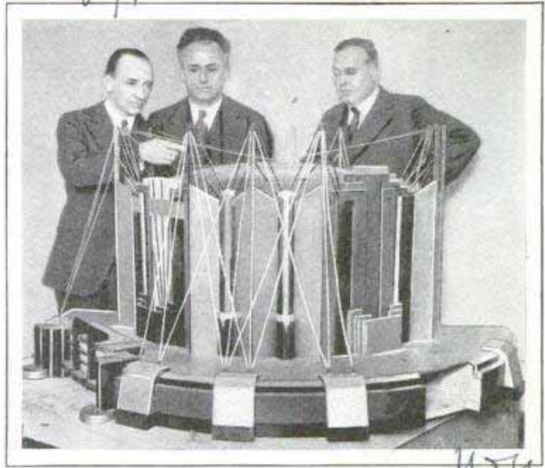
Scale Model of Section of a Building Supported by Specially Braced and Arranged Hooks Instead of Columns
