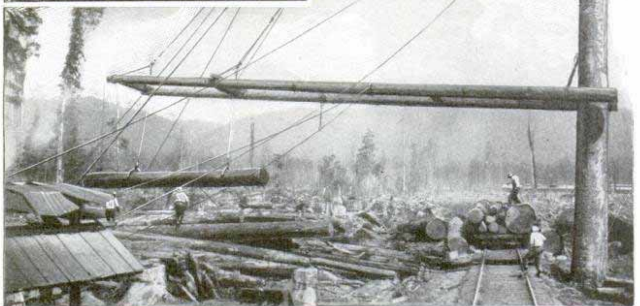
Topper Descending from a Tall Tree after Cutting Off the Top and Branches, and Loading Logs on Cars by a Boom Rugged to a Spar Tree
