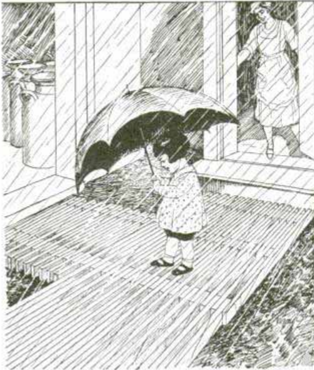
Cheap Sidewalk Made of One-by-Four-Inch Boards for Muddy Patches between Farm Buildings
