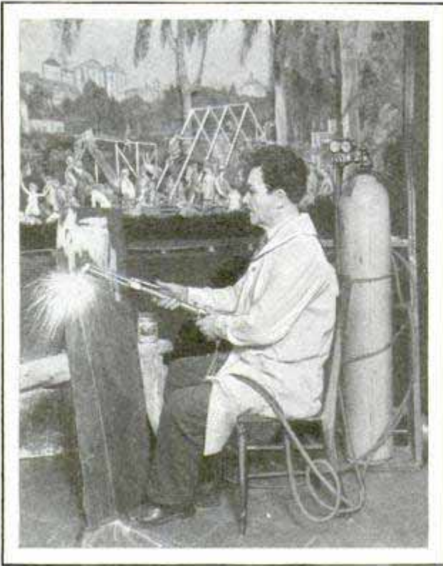
Sheet Metal Is Used as Substitute for Wallboard in Miniature Exhibits
