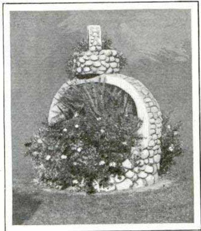
Large and Small Flower Baskets Made of Concrete and Cobblestones
