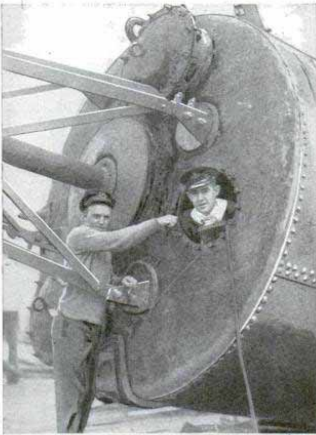
Two Views of Coast-Guard Employees, Giving Spring Housecleaning to a Whistling Buoy Before It Was Taken to Sea to Be Placed in Service
