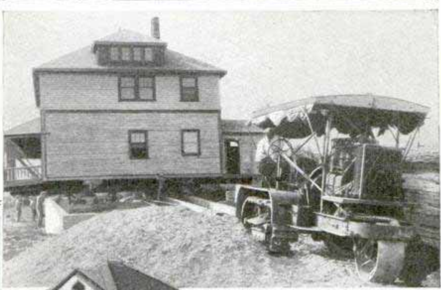
Pulling a House over River on Temporary Bridge with Tractor
