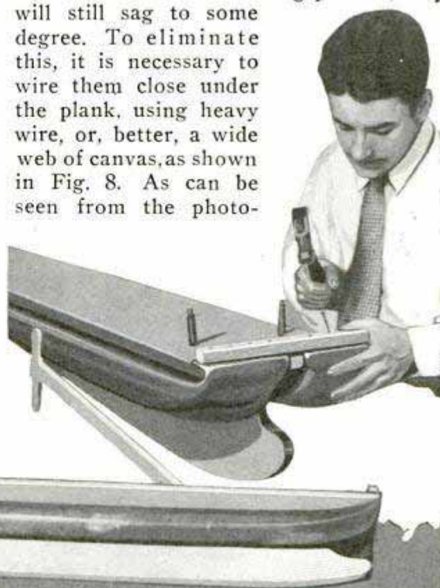
Fig. 3, Left, Nailing the Vulcanized End to the Plank; Below, Stretching Tube to Opposite End •
