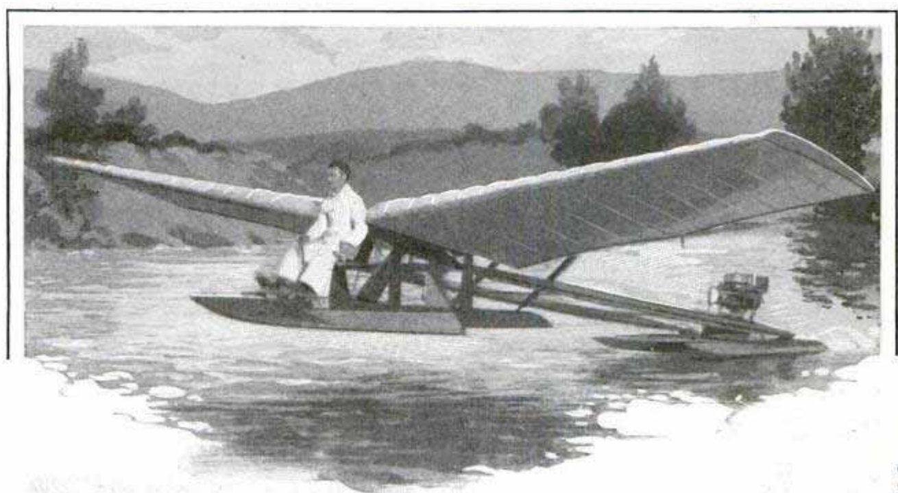
Motorboating and Flying Are Combined in This Waterplane, a Boat That Flies and an Airplane That Swims, All in One; an Outboard Motor Furnishes the Power to Fly or Float
