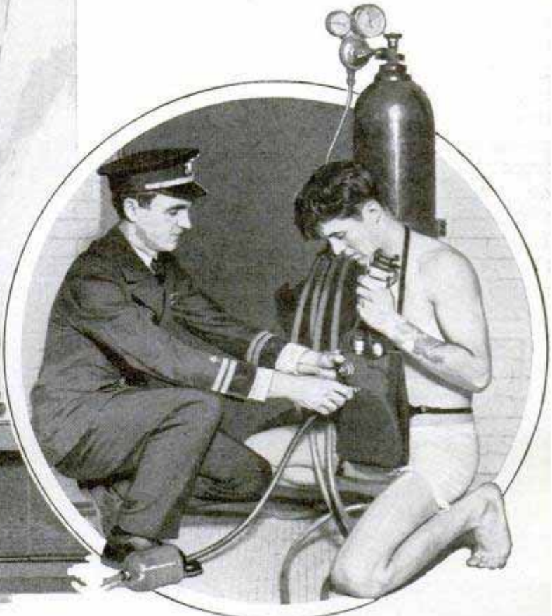
Left, 130-Foot Water Tower for Training Submarine Crews to Escape from Disabled Craft; They Enter the Tank through a Regulation Submarine Hatch at the Bottom and Float to the Top; Right, an Artificial Lung for Breathing during the Rise through 100 Feet of Water
