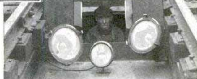
Above, Photo Taken from Pit under Track in Which an Inspector Watches Moving Railroad Cars for Defects; Right, Inspectors at Work
