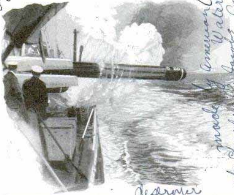
Torpedo Being Launched from British Craft during Fleet Target Practice; the Missile Was Fired with Compressed Air
