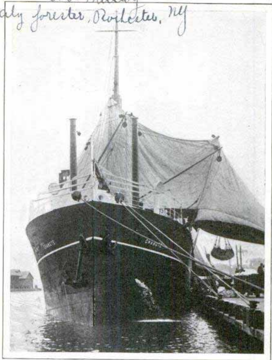
Huge Canvas Canopy over Deck of Vessel and Dock, So Flour Can Be Taken Aboard in a Rainstorm without Damage
