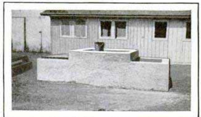
Center Portion of Stock-Watering Tank Shaded from the Sun to Keep Water Cool
