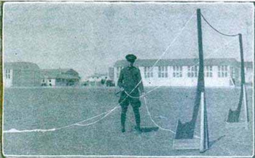
Setting Up Standards of the Message-Hook Apparatus Whereby Planes Pick Up Communications from the Ground as They Fly Low; the Artist's Sketch Shows Pursuit Planes Nearing Bottom of a Dive and Keeping Almost Perfect Alinement
