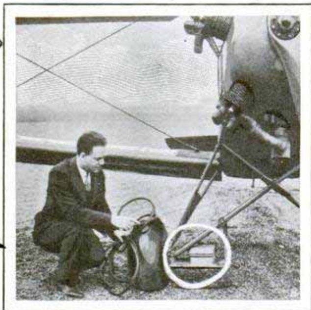
Shock Recorder Attached to Airplane Landing Gear
