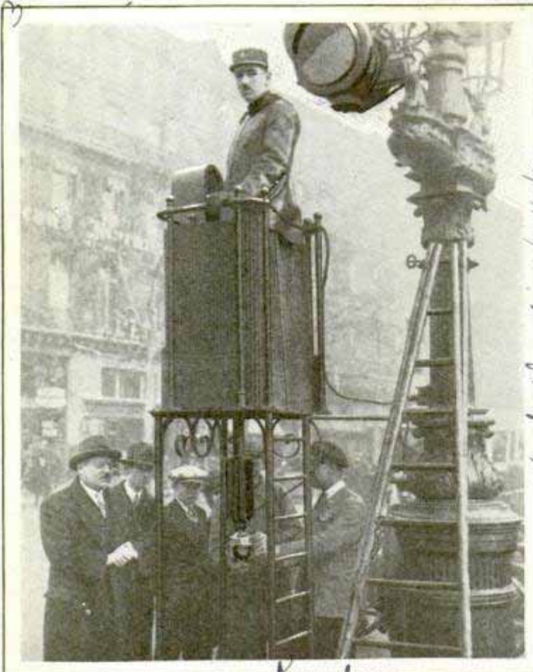
Paris Traffic Tower Equipped with Gas Heater beneath the Floor, to Keep the Traffic Officer's Feet Warm
