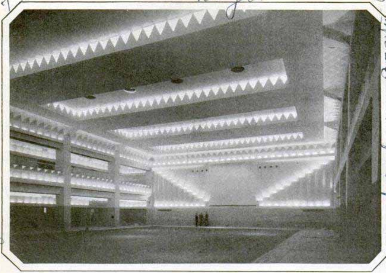
Courtesy General Electric Co. Seven Thousand Electric Lights, Controlled by One Person at the Console of a Color Organ, Provide the Only Decoration for This Ballroom, the Walls of Which Are Solid White
