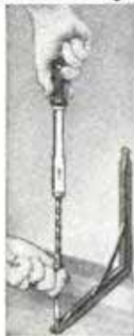
Driving screws at express speed.
