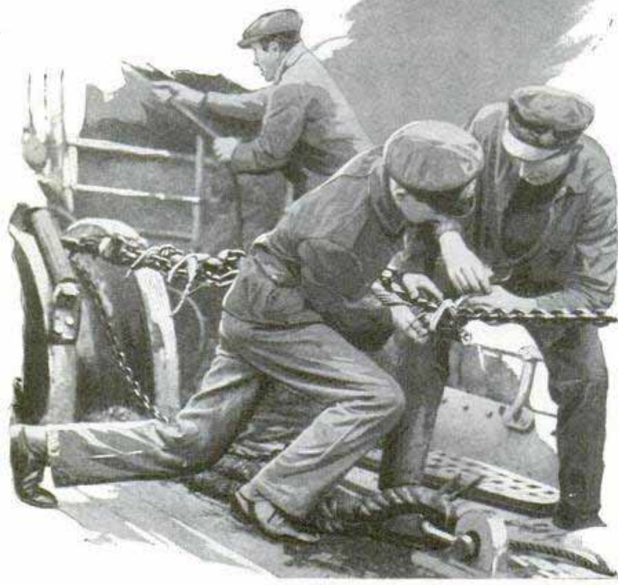
Top, Rigging On a Mark Buoy of One of the Veteran Cable-Repair Ships; Below, Repairing a Broken Cable After It Has Been Raised
