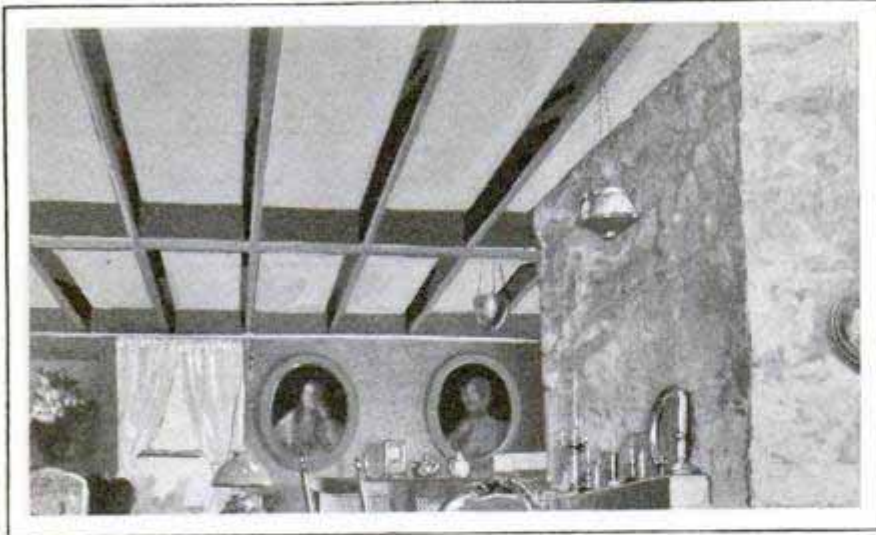
Beamed-Ceiling Effect, Obtained by Exposing the Joists, Adds to the Attractiveness of the Cottage or Lodge
