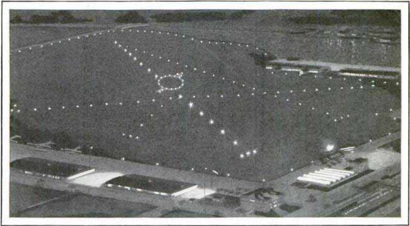
Landing-Field Lights and Wind Arrow Which Are Illuminated Automatically to Indicate the Runways and Show the Direction of the Wind for the Guidance of Pilots at Night
