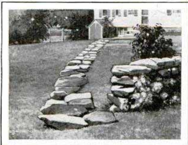
Flagstones Laid Out on the Lawn to Get Good Arrangement before Setting Them Permanently
